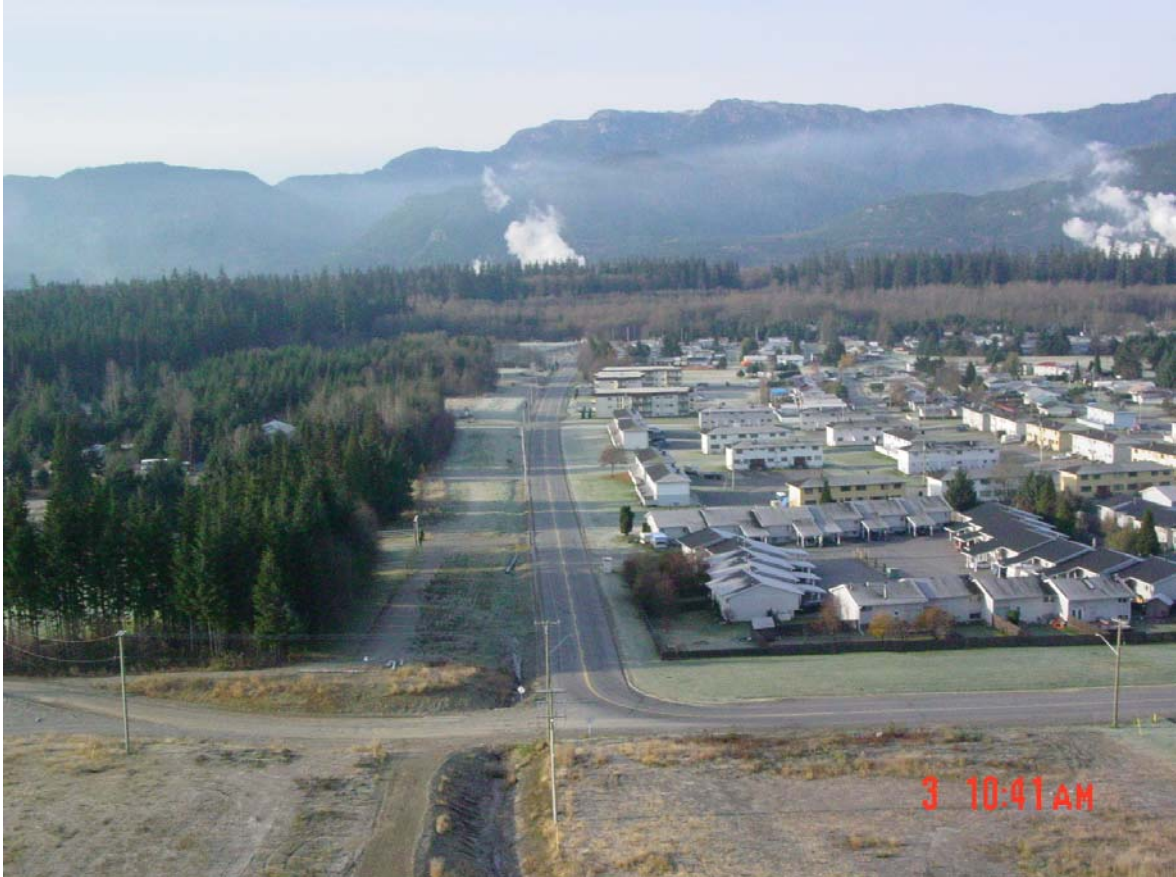
Figure 7. Typical existing right-of-way in the Kitimat Village area.
