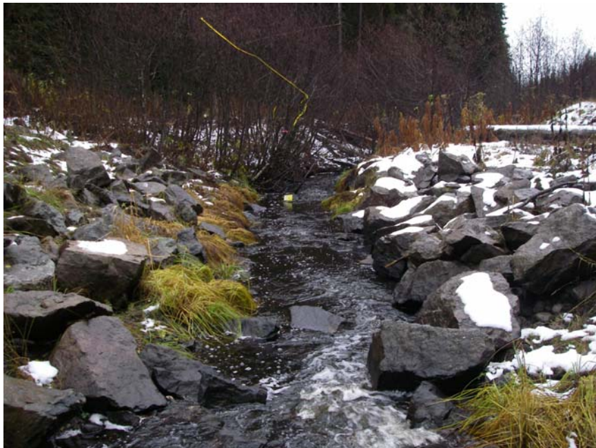
Photo 5: Crossing – view downstream.
