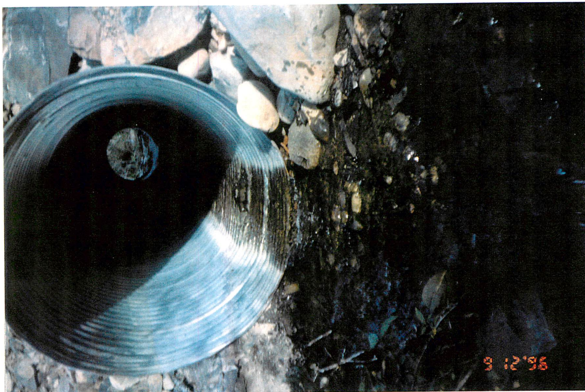
Photo #: A-2-19, 12-Sep-96 Site #: A14, Upstream view through culvert.
