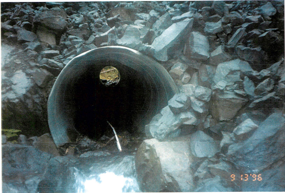
Photo #: A-2-24, 13-Sep-96 Site #: A15, Culvert parallel to flow.
