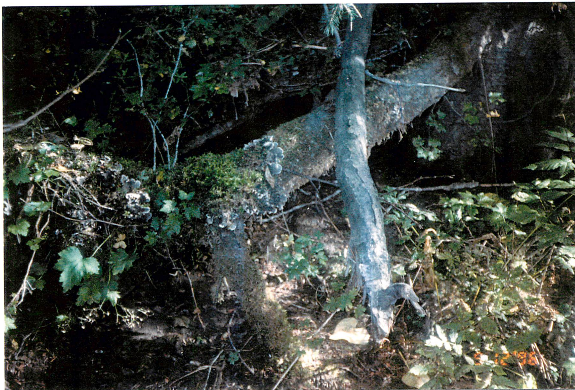
Photo #: A-2-16, 12-Sep-96 Site #: A13, Tree roots exposed by high flows.
