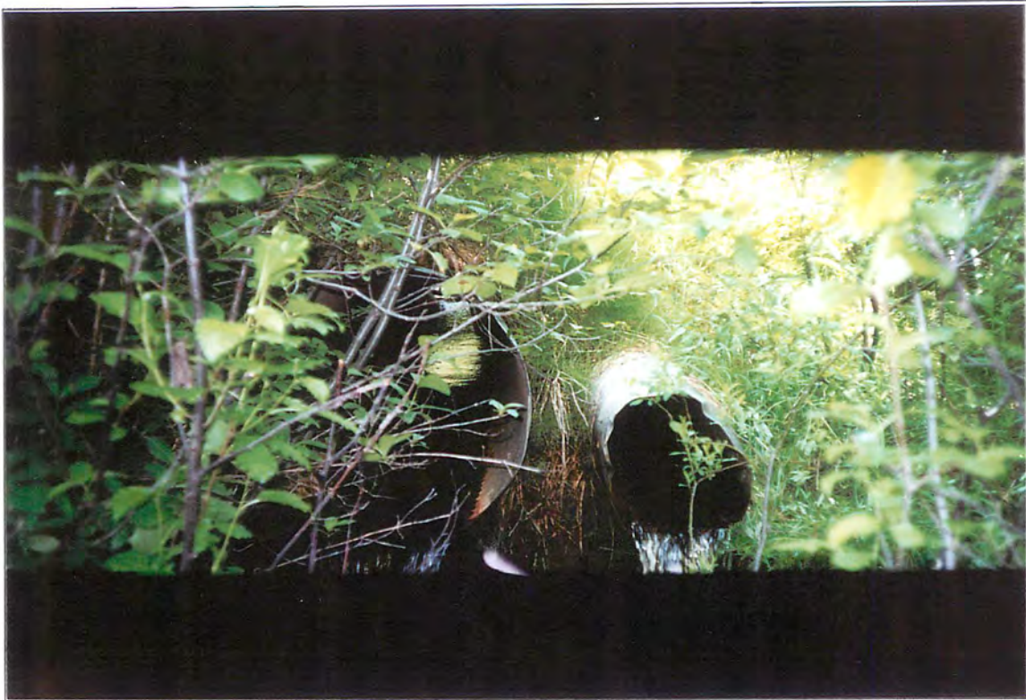
Site #65, twin culverts, 450mm and 900mm, 40cm and 35cm drop, 60cm pool. Roll #6, Frame #04, Date: 2001/07/11
