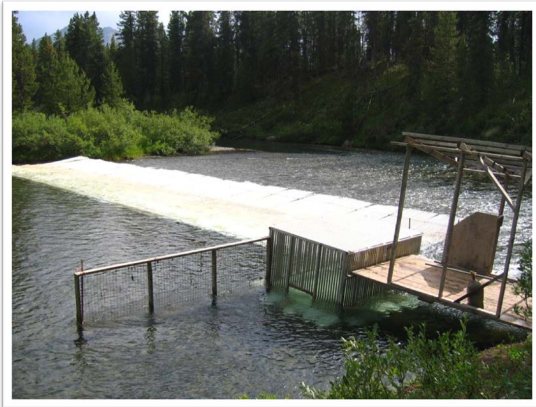
Figure 3. Upper Sustut Steelhead enumeration fence, looking downstream. Photo courtesy of Brome and Leaf Steffey.
