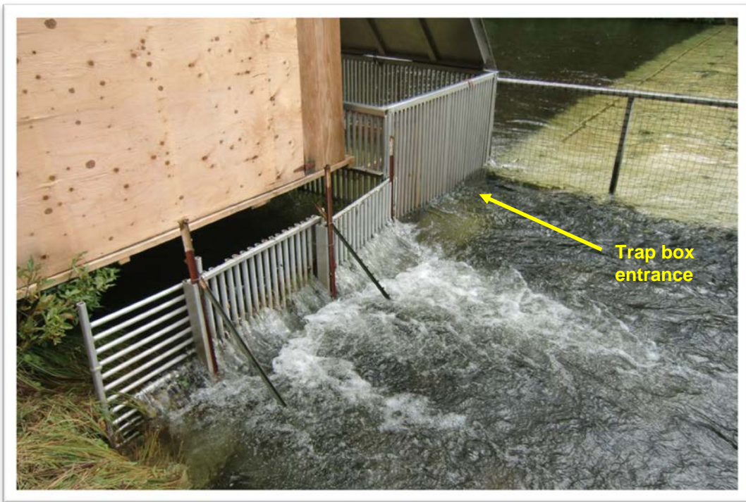
Figure 7. Trap box entrance looking upstream. Photo credit Mark Beere.
