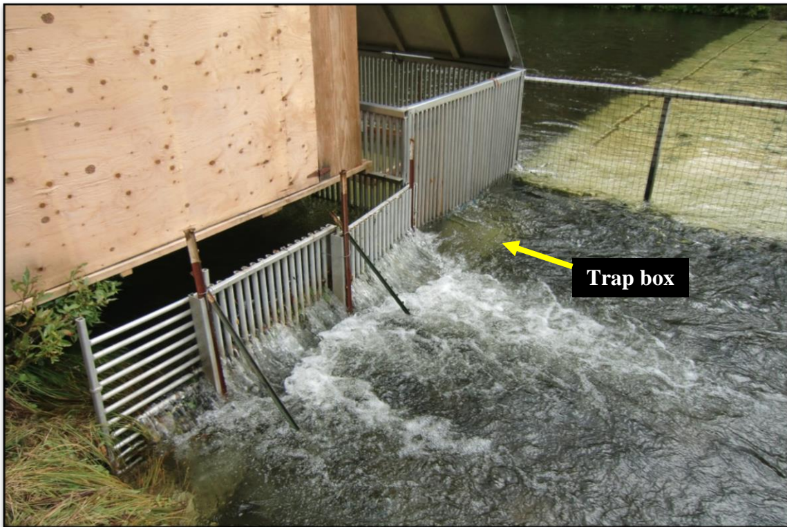
Figure 7. Sustut enumeration weir trap box entrance Photo courtesy of Mark Beere
