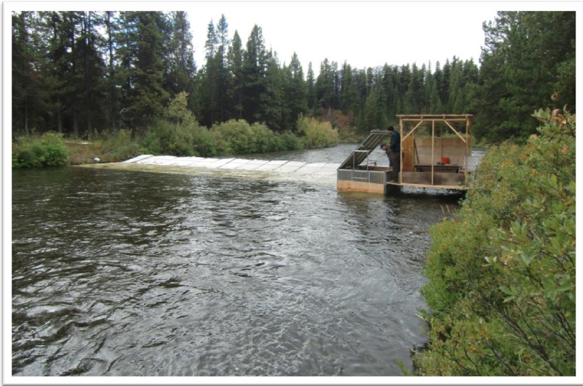
Figure 5. Sustut enumeration weir looking downstream Photo courtesy of Mark Beere
