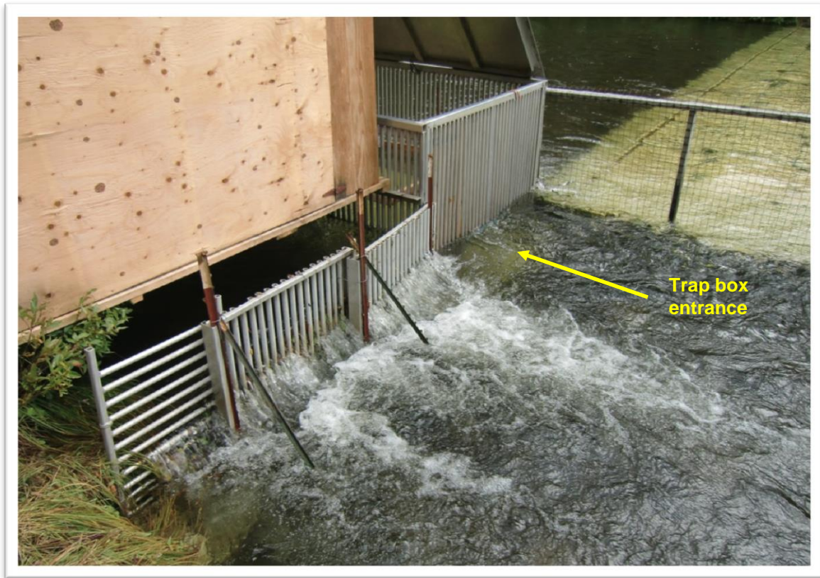
Figure 7. Sustut enumeration weir trap box entrance Photo courtesy of Mark Beere
