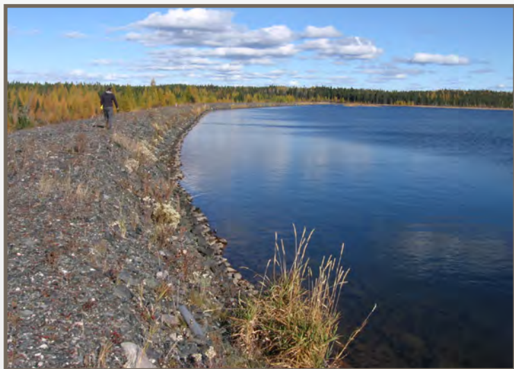
Dam C at North End of Tailings Pond
