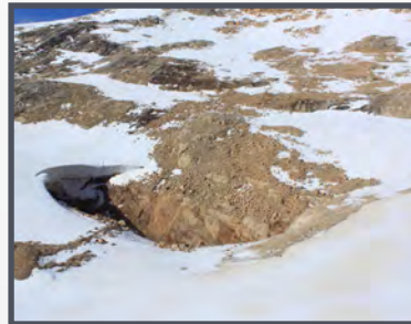
Sinkhole by Kodiak B underground
