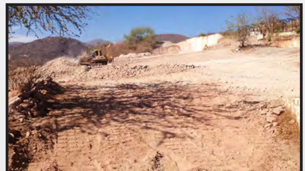
Mill Area After Earth Works
