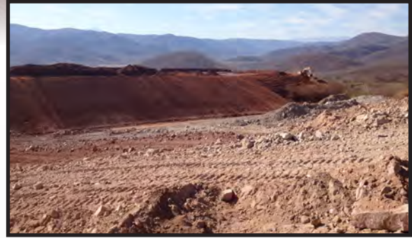
Plant Site After Earth Works
