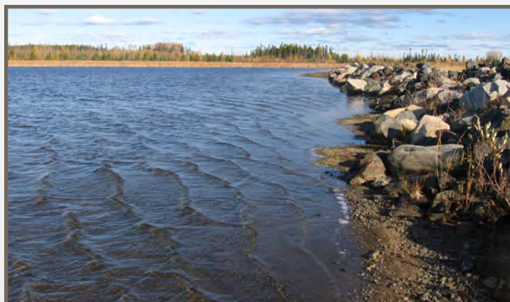
Erosion Protection Between Tailings Pond & Dyke 3 Beach
