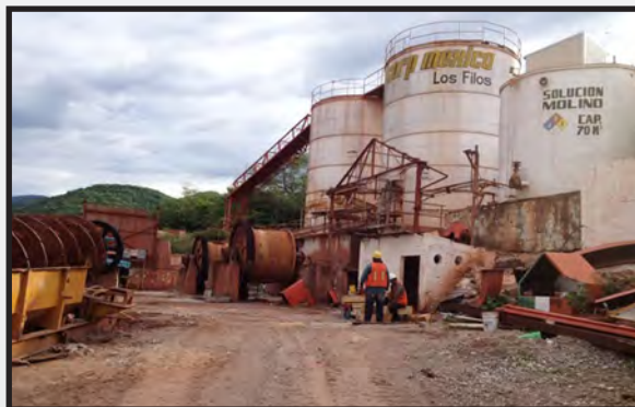
Tanks That Were Removed
