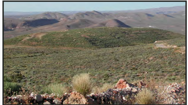
Reclaimed Heap Leach Facility
