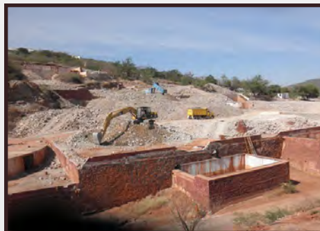
Filling Plant Area
