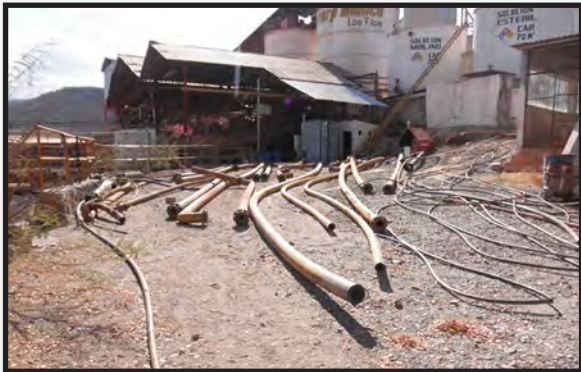
Pipelines Before Reclamation
