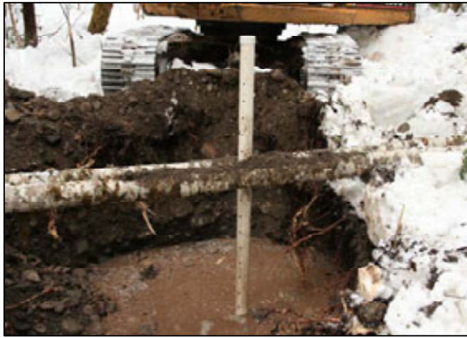
Figure 28. Standpipe back-filling.
