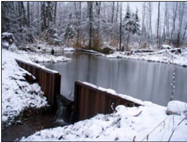
Figure 42. Water augmentation dam and supply for the spawning channel shown above.
