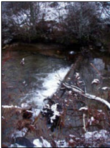
Figure 43. Perpendicular log weir spanning Scully Center Channel. Figure 44. View downstream on Scully Center Channel.
