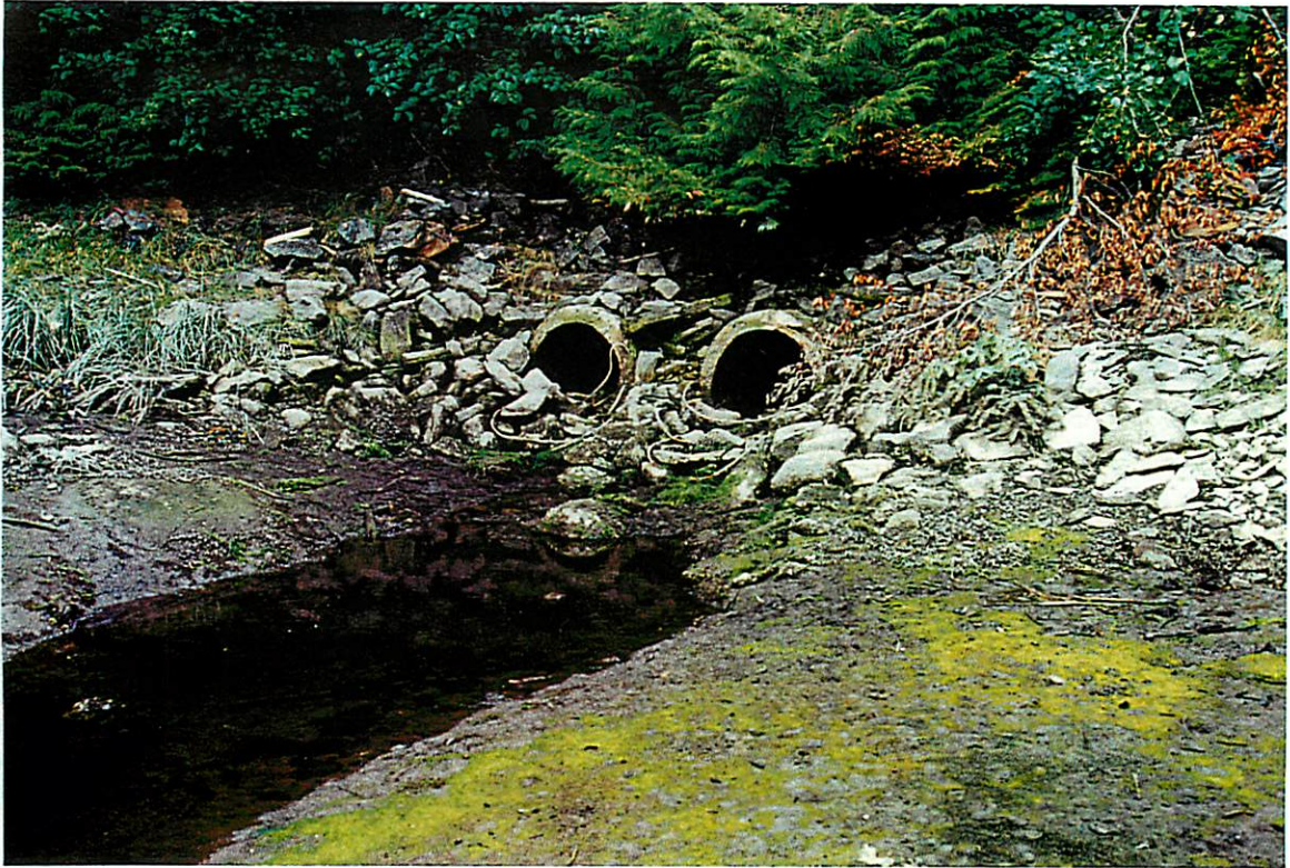
Photo 4.5-1 Culvert of unnamed creek east of site
