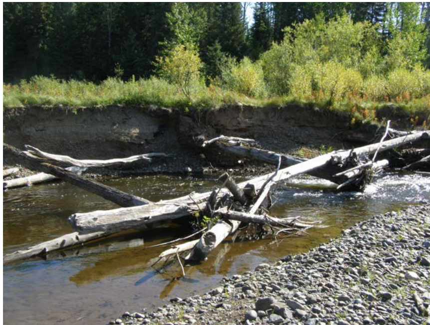
Looking across stream at undercut bank. Habitat structures still provide influence but extreme flows have down cut channel.
