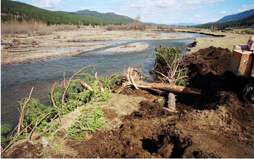
Figure 5: A habitat structure is placed downstream of the previous structure. The tops of the material from the upstream structure protect the downstream structure.
