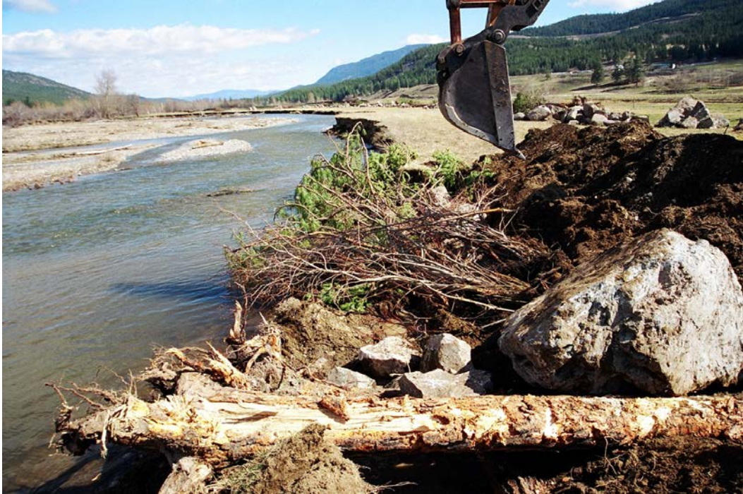
Figure 4: More brushy material including live willows are added and secured with rock and soil. Care is taken while the trench is being backfilled not to displace the dirty water into the river. It is removed from the trench with the bucket or a pump and moved far enough from the river that there is no sediment returning to the flowing water.
