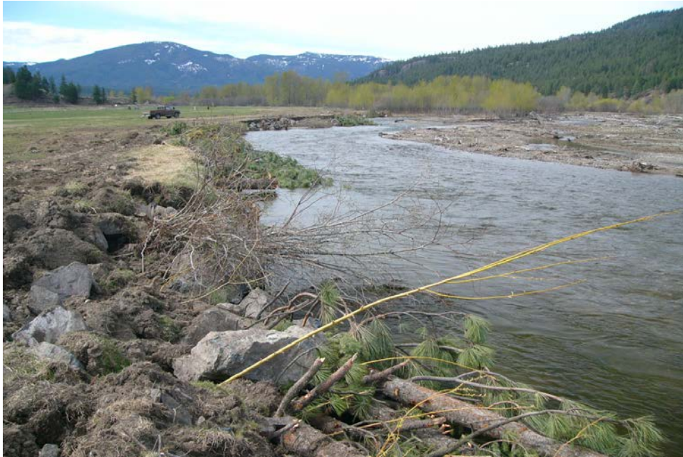
Figure 6: The structures are placed close enough on this outside corner to overlap and appear continuous. Eventually, the soil berm that was left during construction may be eroded, leaving the rock toe with overhanging wood. The live willow, placed with the roots below the high water table, continue to grow through the rock and wood. Cattle are reluctant to walk on the rock and debris to graze the willow overhanging the river.
