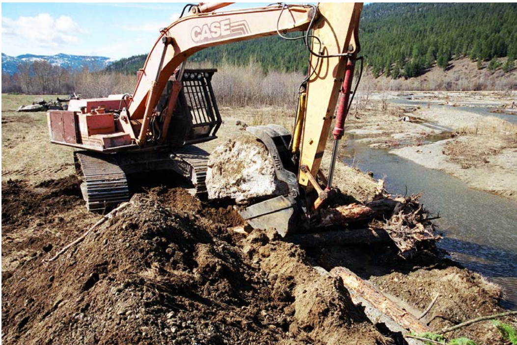
Figure 3: Rock is placed along the bank side of the berm to secure the toe of the bank and is used to anchor the wood.
