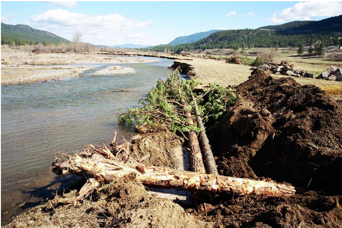
Figure 2: Wood and brush are placed in the trench extending over the water. Care is taken to leave the berm in tact and the work area isolated.
