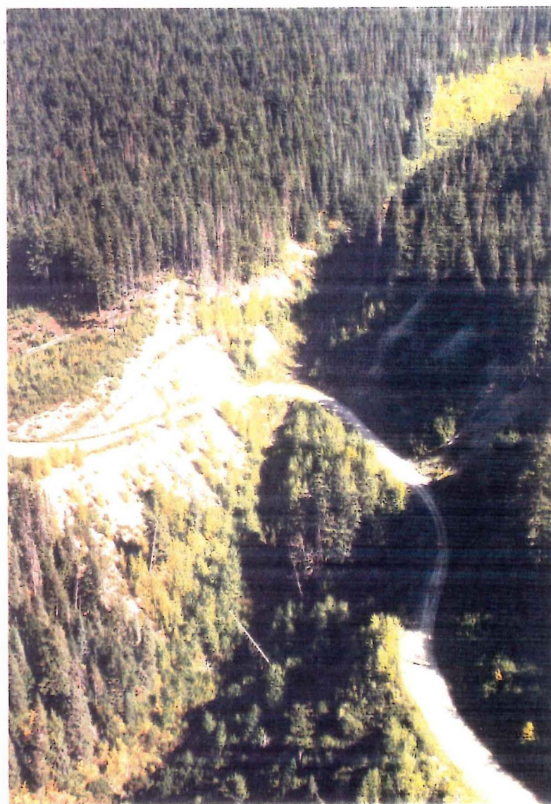
Photo 6. Cut and fillslope erosion into tributary of Natlan Cr. 93M 034.
