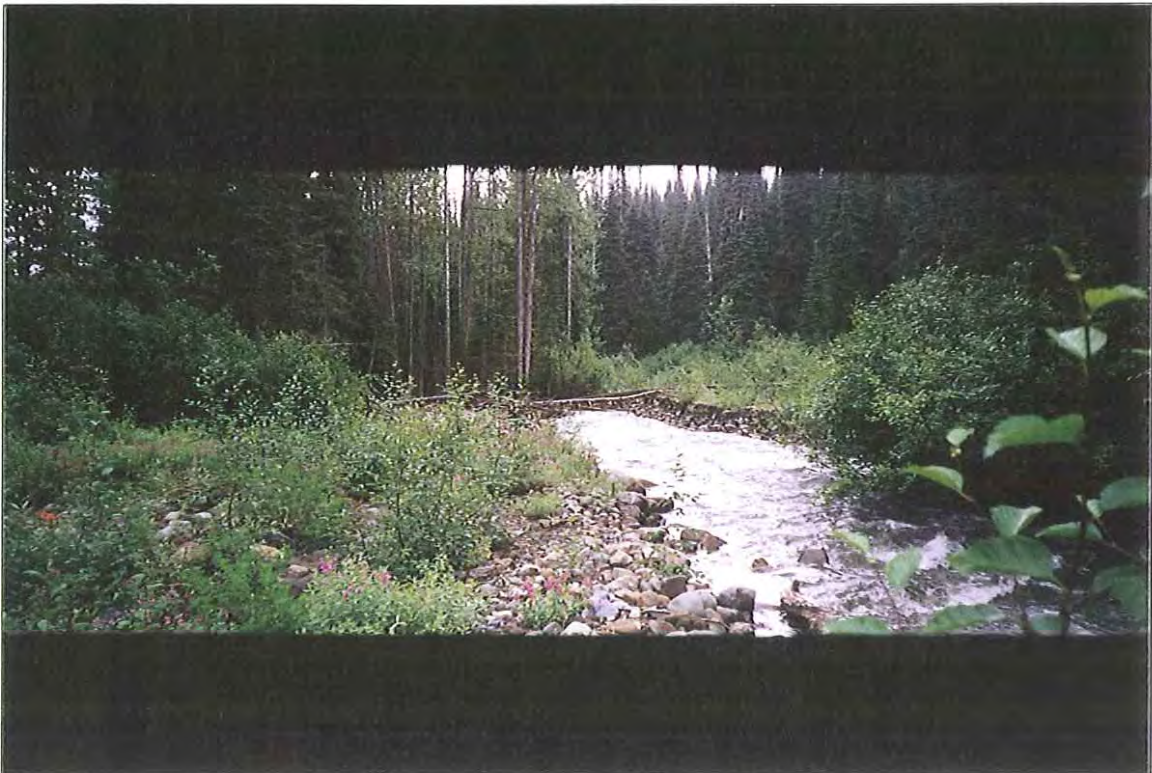
Site #12, Downstream photo of open section with spanning LWD. Roll #2, Frame #2, Date: 2001/08/06
