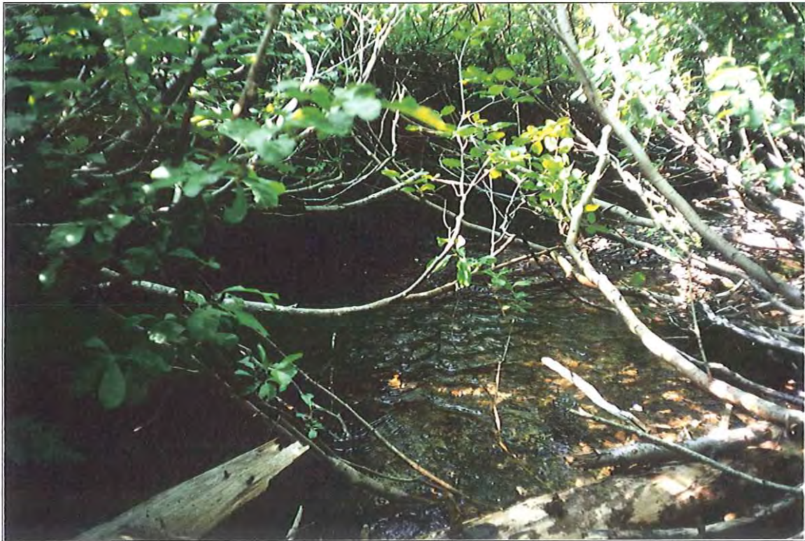
Site #242, Downstream photo of heavily overgrown section. Roll #23, Frame #23, Date: 2001/08/09
