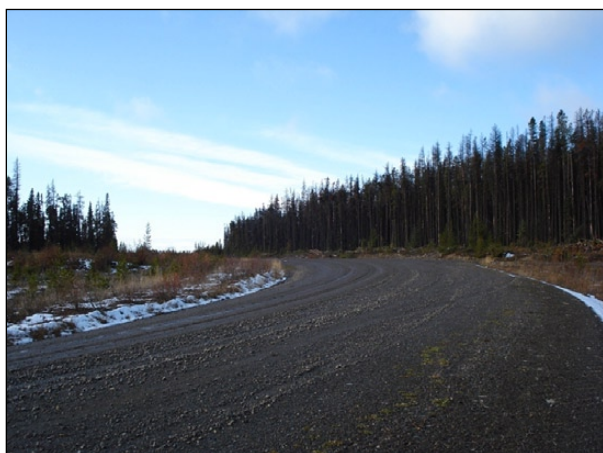
FIGURE 1. Photo of a mainline road (junction of the Augier and Grizzly Forest Service roads).
