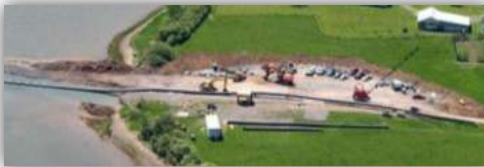
Figure 2: Open Cut Trench Shore Approach
