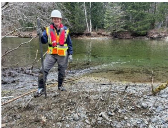
Figure 1. Live willow stakes shown in the foreground, planted in river right bar at the confluence of Green Creek and the Nanaimo River (photo taken March 7, 2025).
