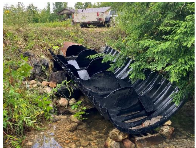
Figure 1. Example polymer-coated steel Fishculvert fishway with baffles installed at a perched culvert to restore fish passage.
