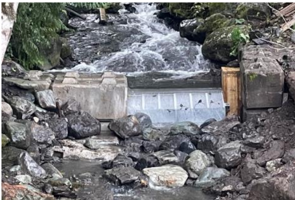
Figure 2. Final intake configuration, looking upstream.
