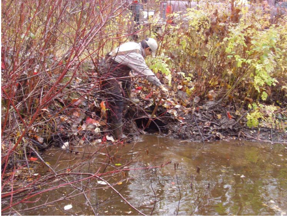
Photo 11: GFA technician clearing culvert intake that was plugged by beavers at Site 22 (Canoe Creek FSR – Km 2.4).
