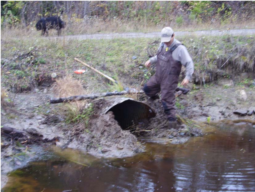
Photo 10: GFA technician cleaning culvert intake that was plugged by beavers at Site 20 (Canoe Creek FSR – Km 2.4).
