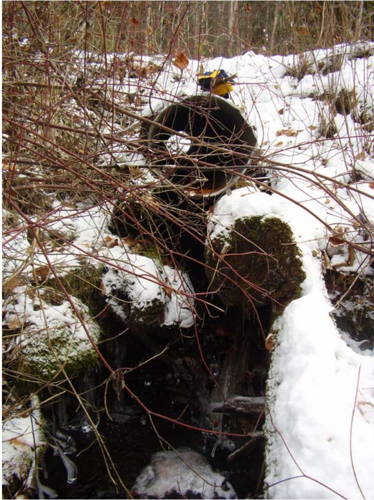
Photo 3: Site 14 looking at dry suspended culvert and water flow through log corduroy below – barrier to all fish.
