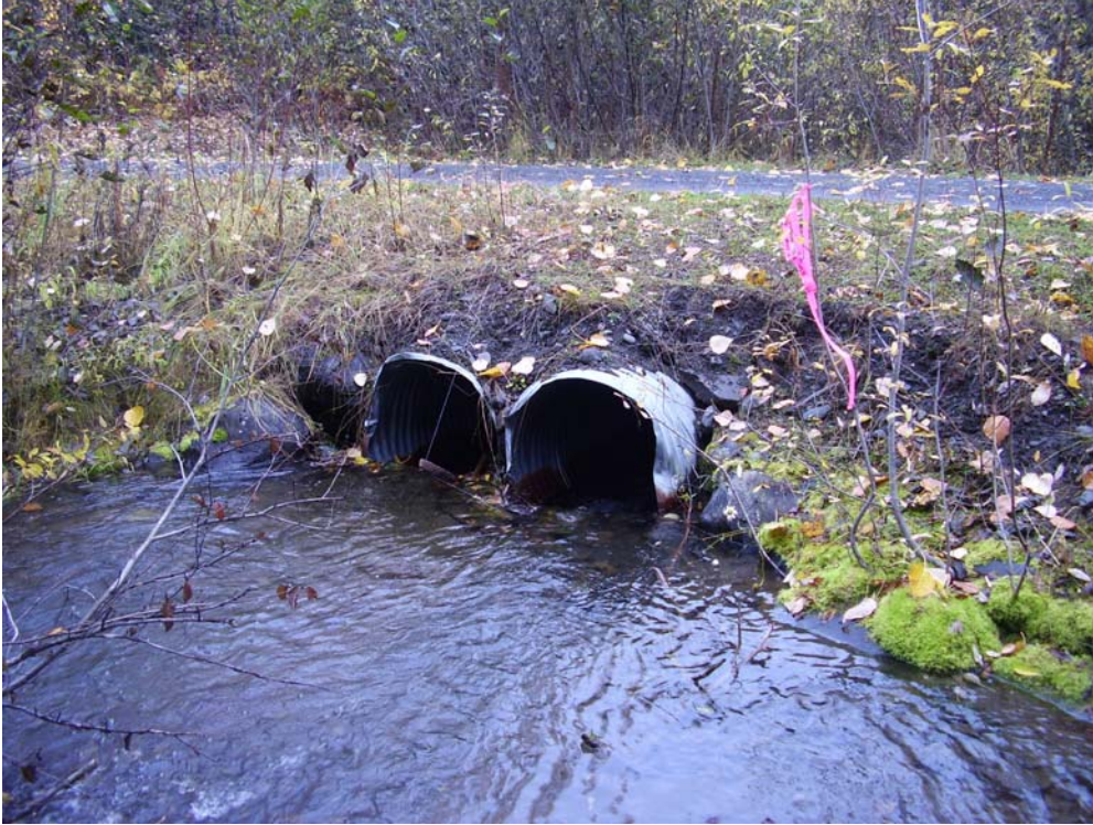
Photo 1: Site 3 looking downstream at culvert inlet – velocity barrier to juvenile salmonids.
