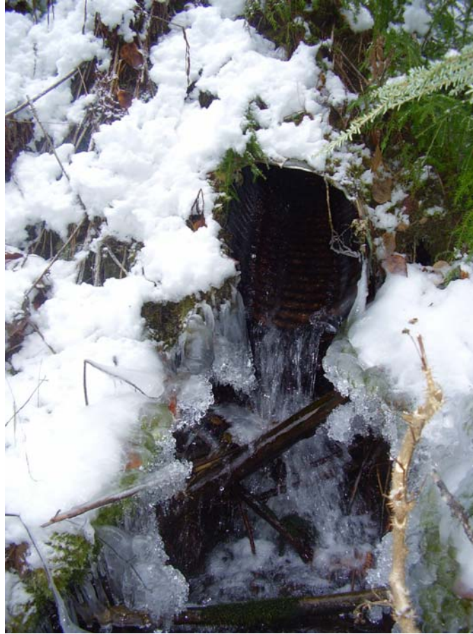
Photo 5: Site 15 looking at suspended outlet – barrier to all fish (24-Mile FSR Km 0.4).
