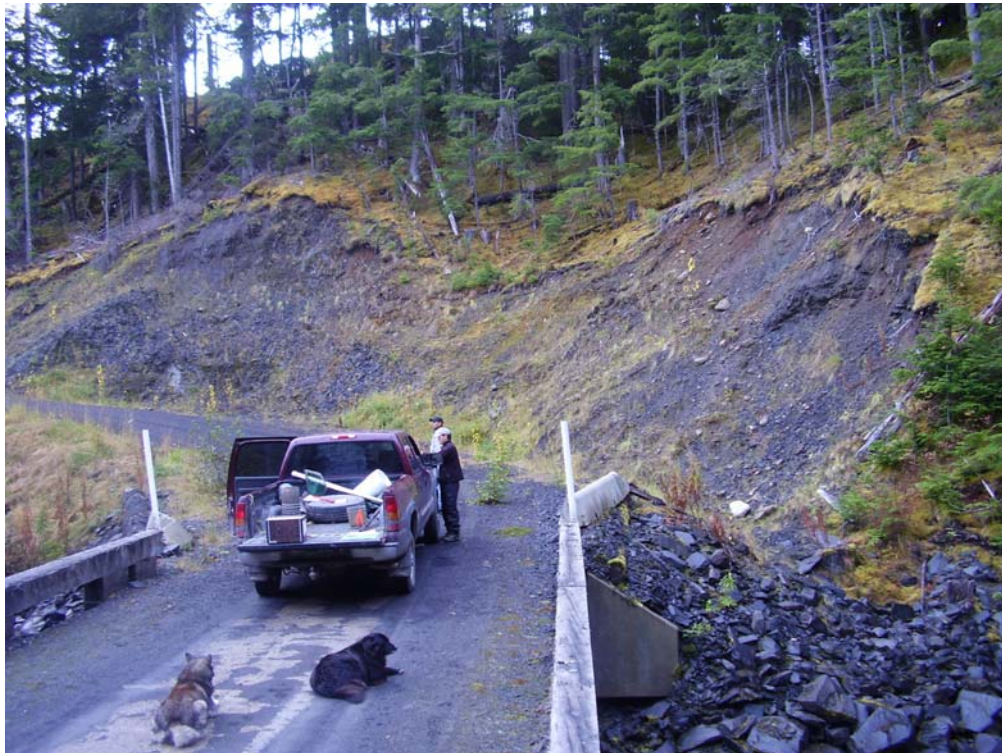
Photo 7: Site 1 looking at large exposed cut bank on right back ditch. SCQI = 1.8 (very high ranking).
