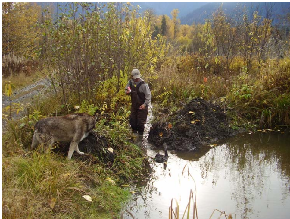
Photo 12: GFA technician clearing back-ditch that was dammed by beavers at Site 9 (Kitwancool FSR – Km 1.8)
