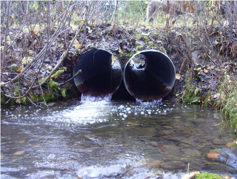
Photo 2: Site 3 looking upstream at culvert outlet – velocity barrier to juvenile salmonids.
