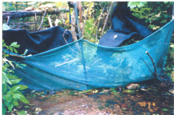
Fig.2 Isolation net at downstream end of work site.
