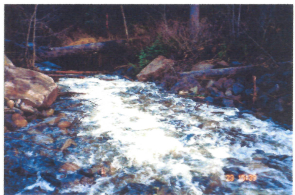
Fig.6 Closer view of face of weir/riffle structure approx. 1.5mo after construction. (Some large boulders in this riffle would provide resting and holding areas for fish).
