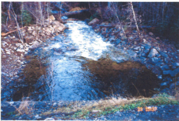
Fig.2 Weir/riffle structure approx. 1.5mo after construction.
