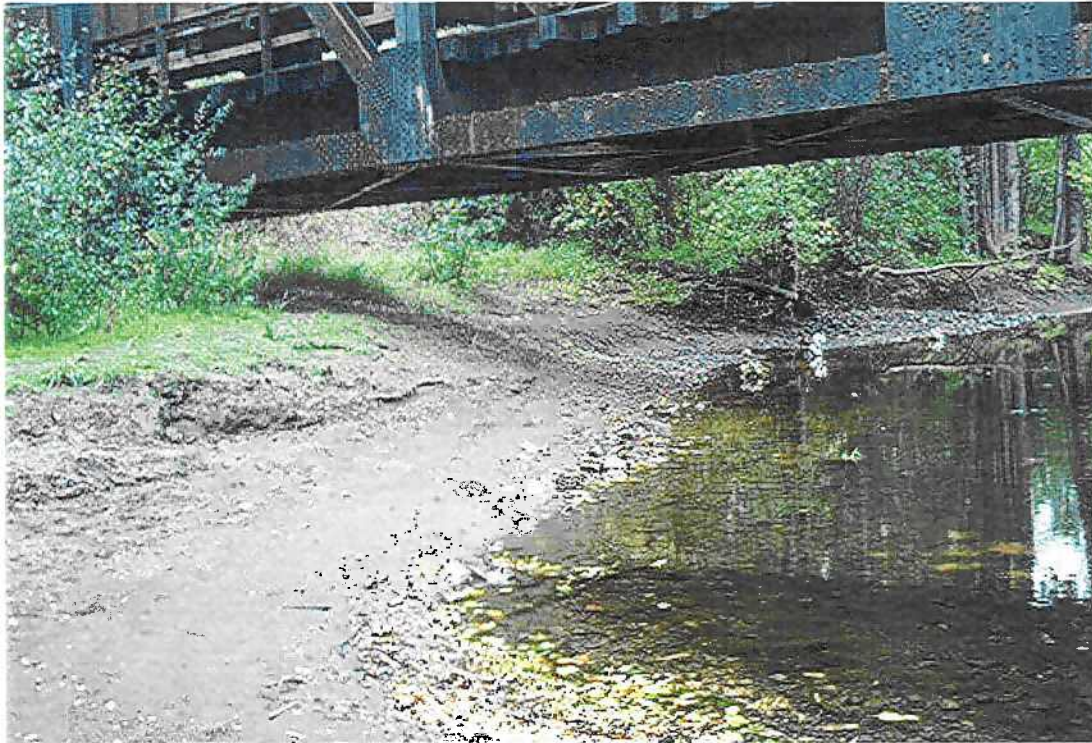
Photograph 3. Left downstream bank under CNR bridge looking southeast (downstream).
