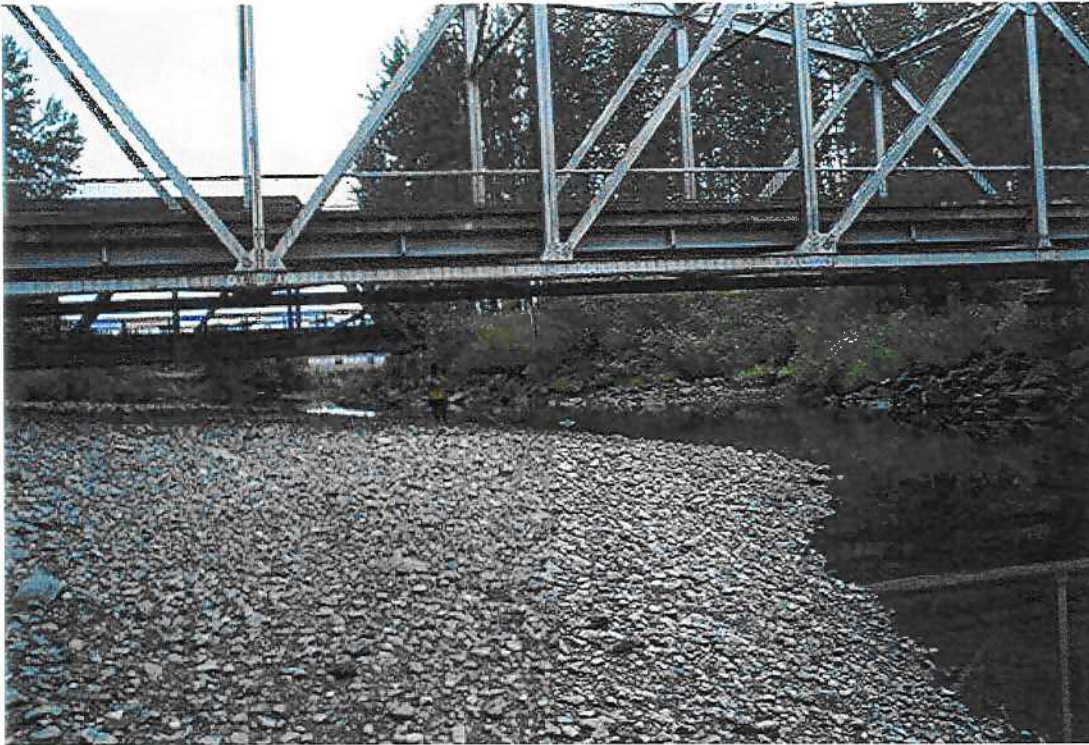
Photograph 9. Taken along left downstream bank (looking south or downstream) showing current water level and exposed side bar that exists under the CNR and highway bridges.
