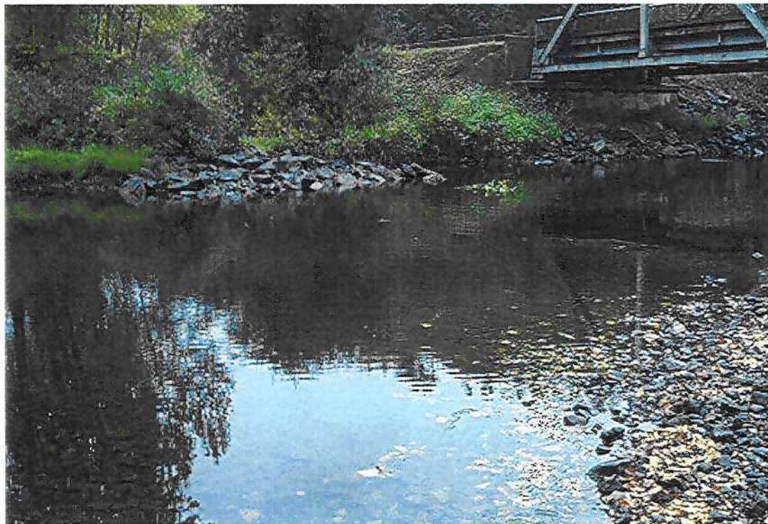
Photograph 4. Run section looking north (upstream) between CNR bridge and Highway 16 bridge.
