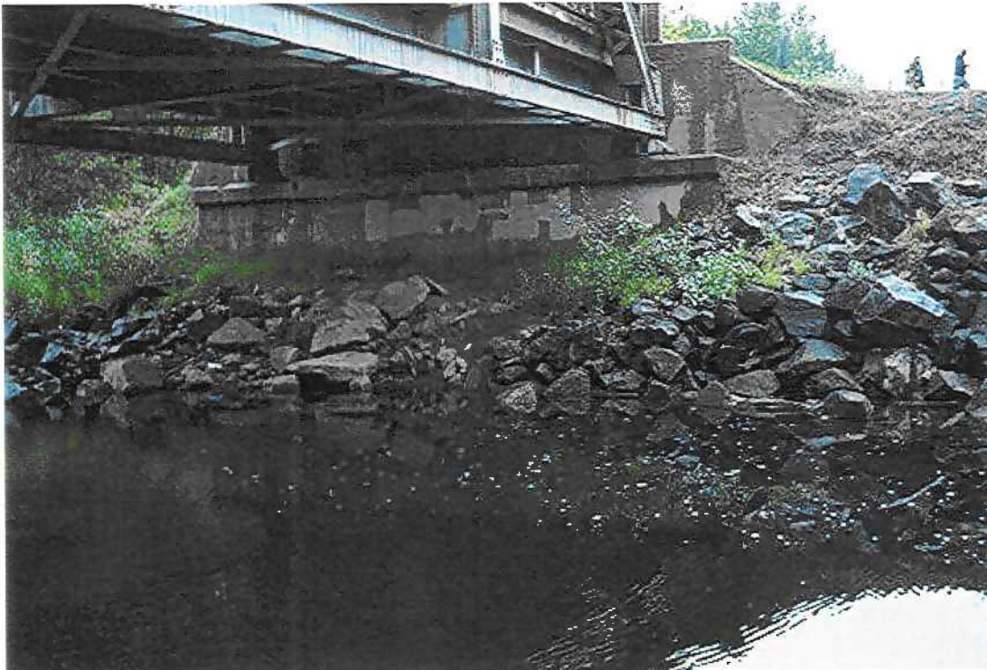
Photograph 7. Right downstream bank highway bridge abutment (west side).
