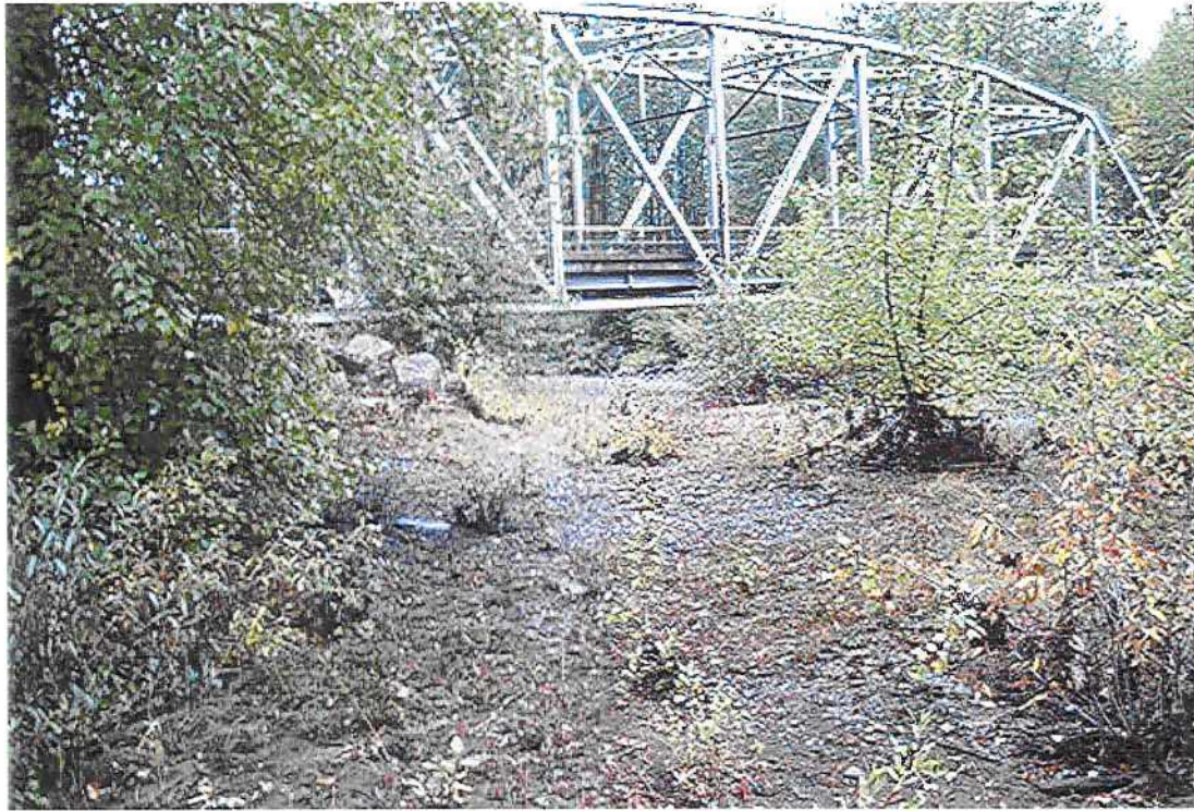
Photograph 11. Top of left upstream bank, upstream of highway bridge, looking southwest.
