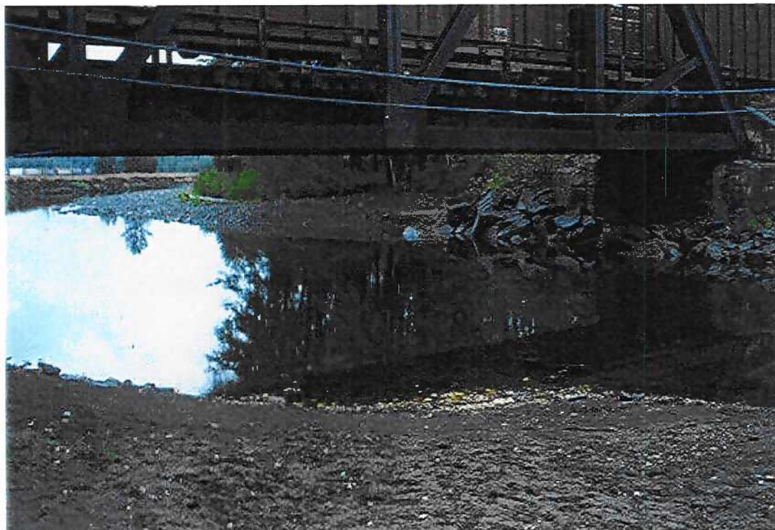
Photograph 2. Right downstream bank under CNR bridge looking west (downstream). Note: resolution is 72 dpi.
