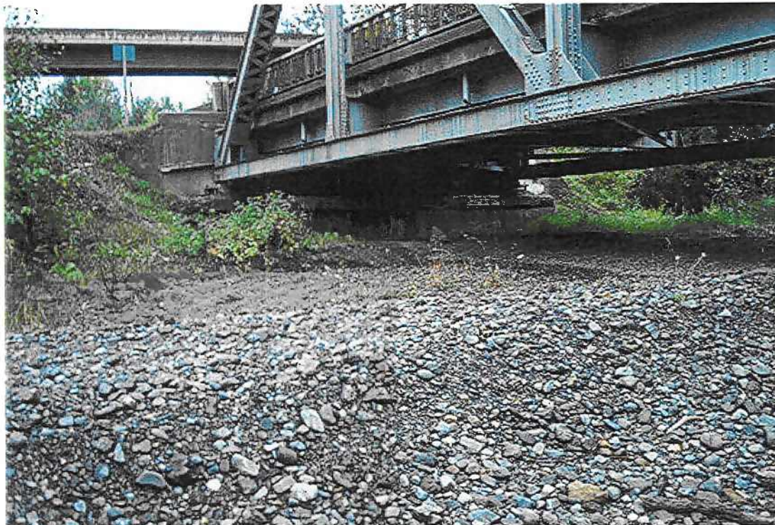
Photograph 8. Left downstream bank highway bridge abutment (east side).
