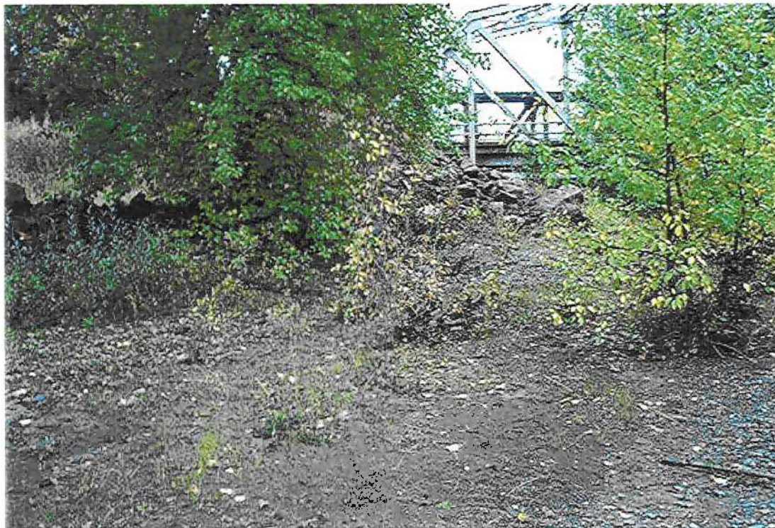
Photograph 12. Top of left upstream bank, upstream of highway bridge, looking southwest.
