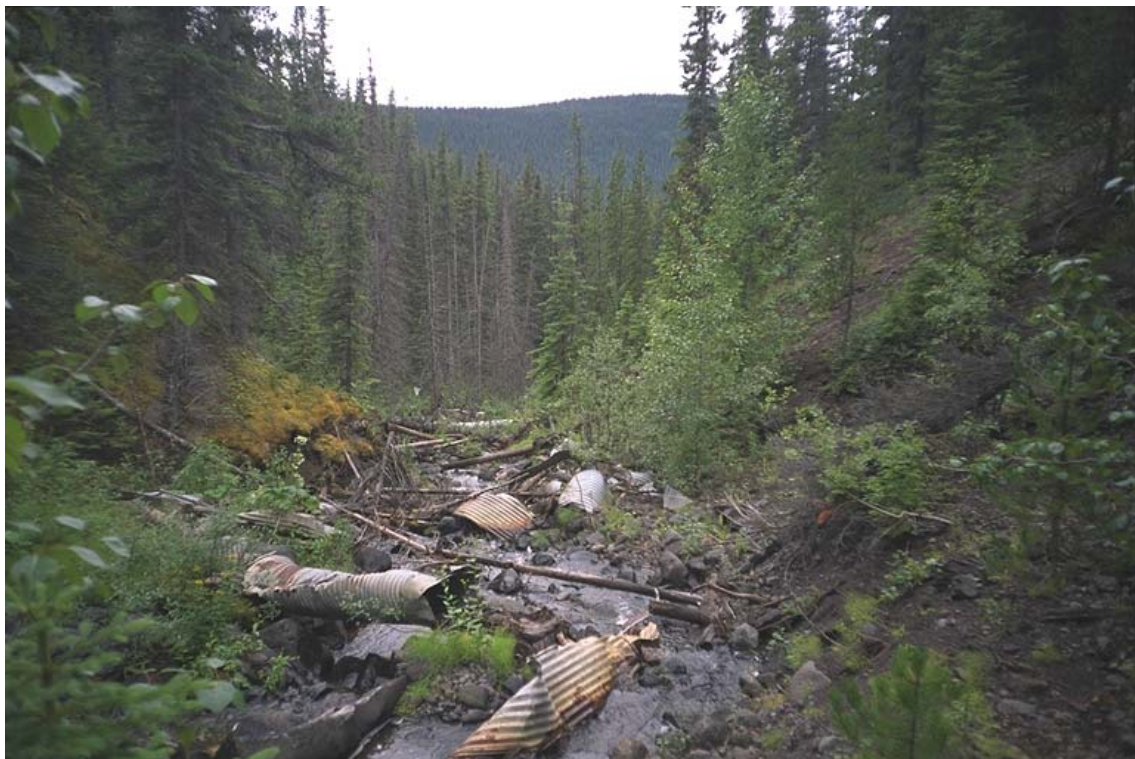
Figure 9. Downstream view of several unraveled and washed out culverts in Dungate Creek (ILP 80004), just downstream of tributary ILP 80017.
