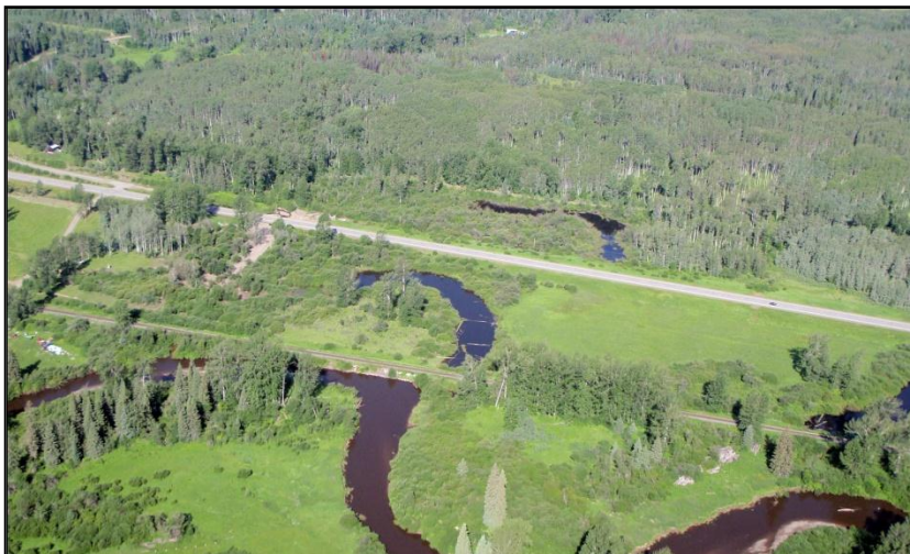
Figure 45. Upper Bulkley River floodplain bisected by CN Rail, Highway 16, and diminished riparian zones.
