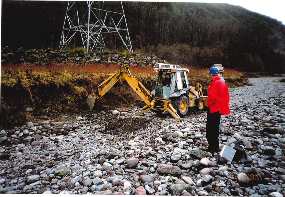
Photo 6: Digging test hole one in the upper channel.
