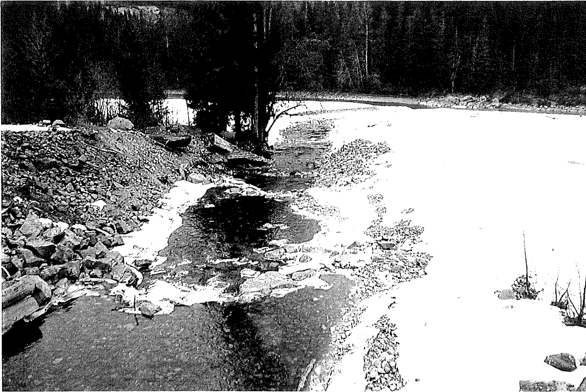
Photo 60: After the construction of two upstream rock vees (March 1998).
