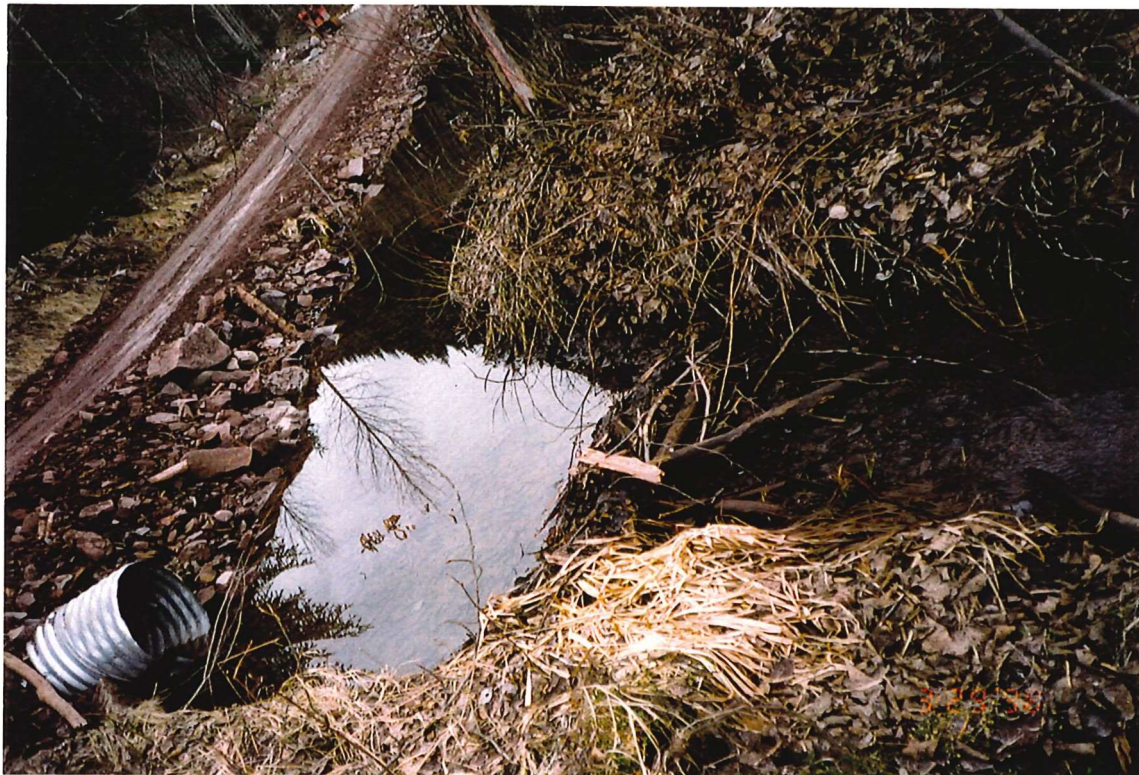
Photo 46: All of Swan Creek flowing into ditch.
