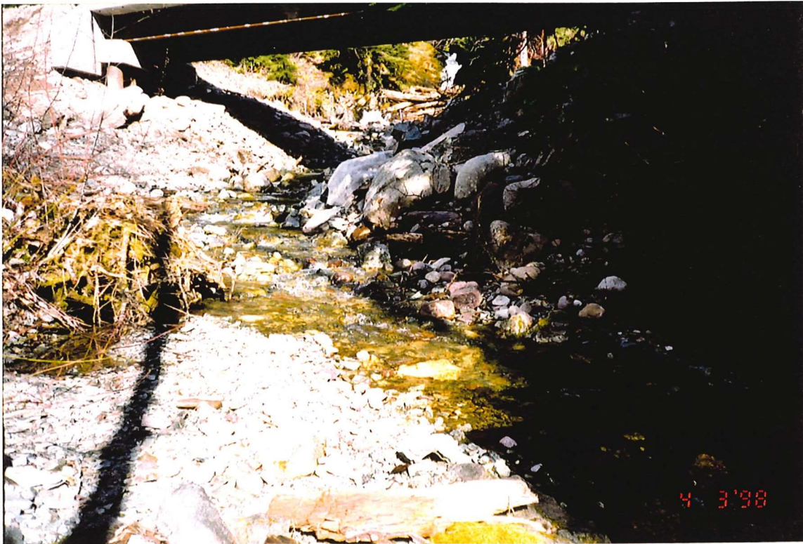
Photo 10: Looking upstream to the bridge.
