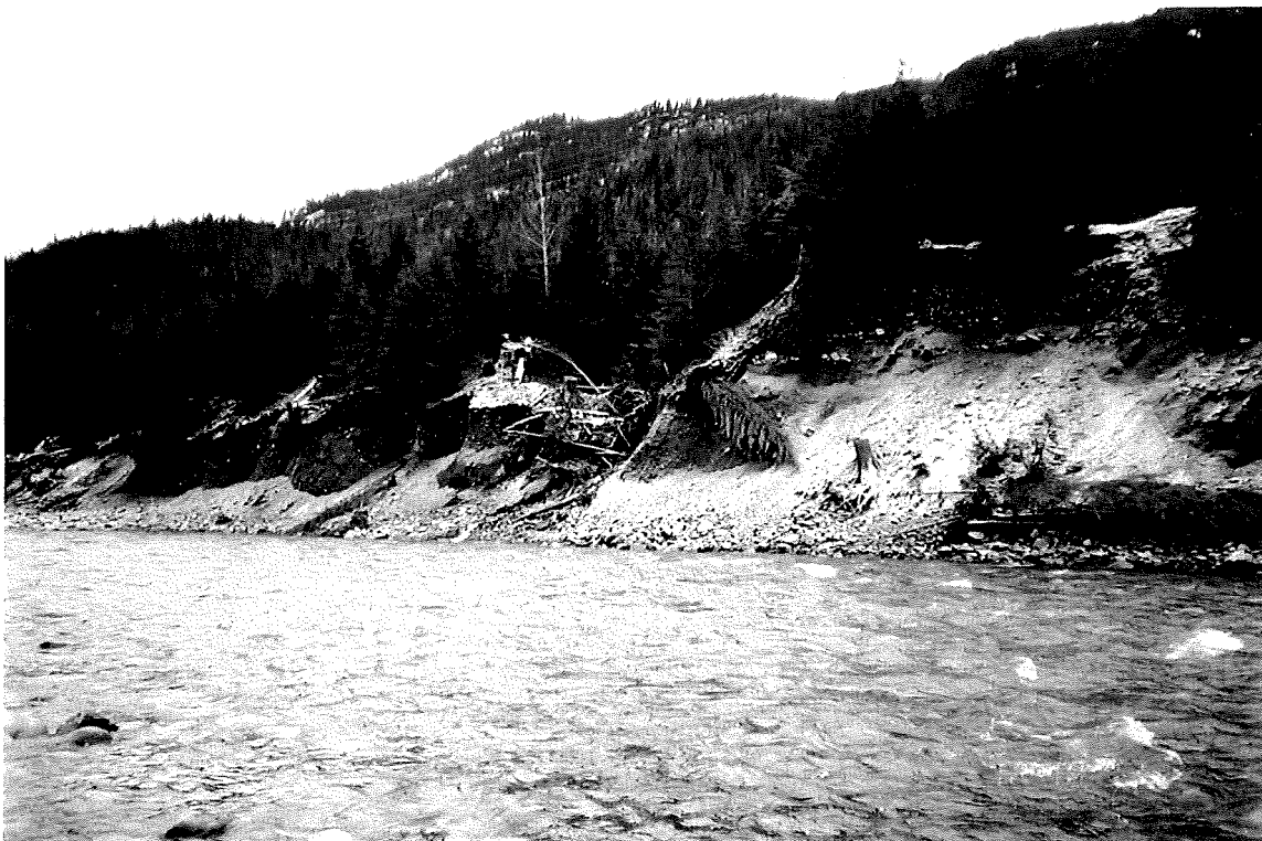
Photo 25: This eroding bank is causing sediment into the Zymoetz River.
