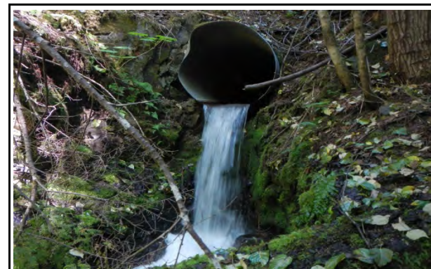
Plate 5 Photograph taken at 100m upstream looking upstream at a hanging culvert.
