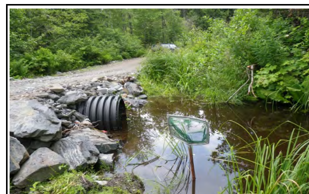
Plate 5 Photograph taken at 20m downstream looking west at a road crossing.
