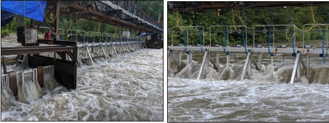
Photo on left shows upstream view from right bank and photo on right is upstream view of KSEF after panels had been opened.
