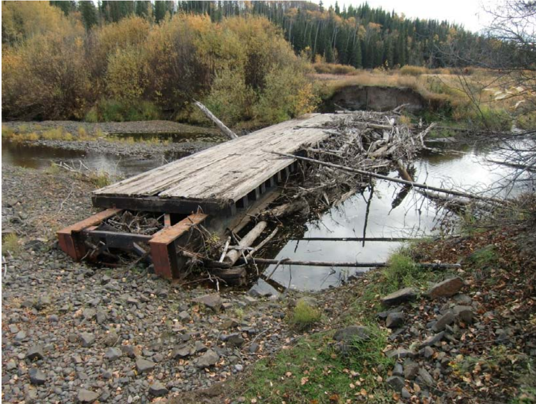
Photo 1. Strimbold Bridge, September 29, 2015.
