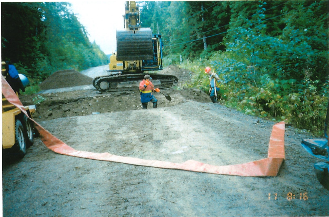
Photo 10-1 Excavating around natural gas line.
