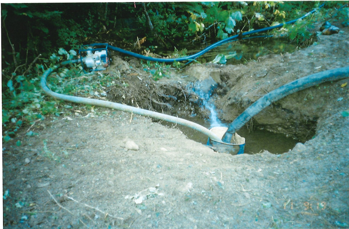
Photo 10-4 Filling upstream sump prior to diversion. Note 3" pump for removing dirty water
