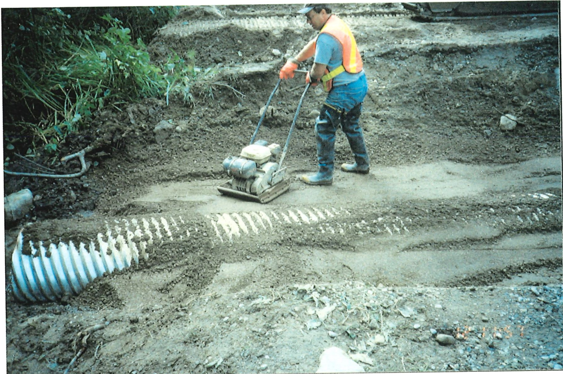
Photo 12-5 Compacting gravel around culvert.
