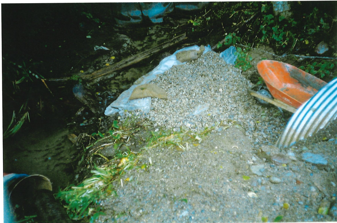
Photo 9-6 Upstream sandbag / poly weir with fisheries gravel for culvert infill.
