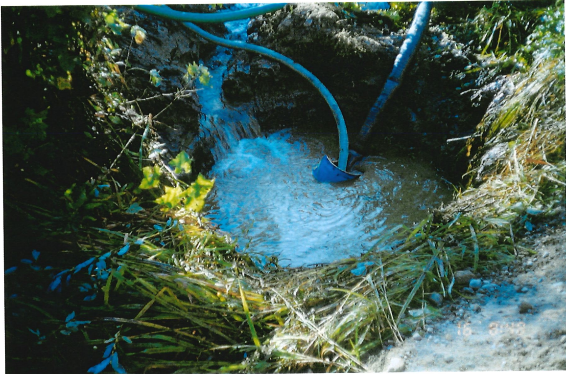
Photo 16-1 Filling upstream sump prior to diversion.
