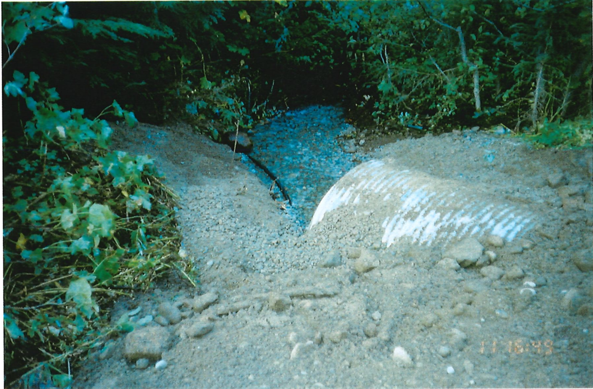
Photo 10-7 Inlet of culvert showing distribution of gravel substrates. Note local water intake adjacent to right bank.
