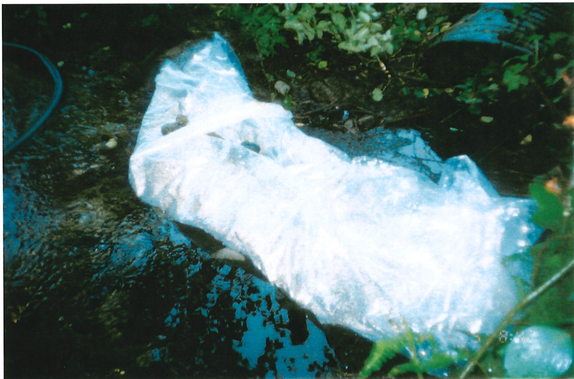
Photo 6B-2 Sandbag / poly weir at upstream end of culvert.
