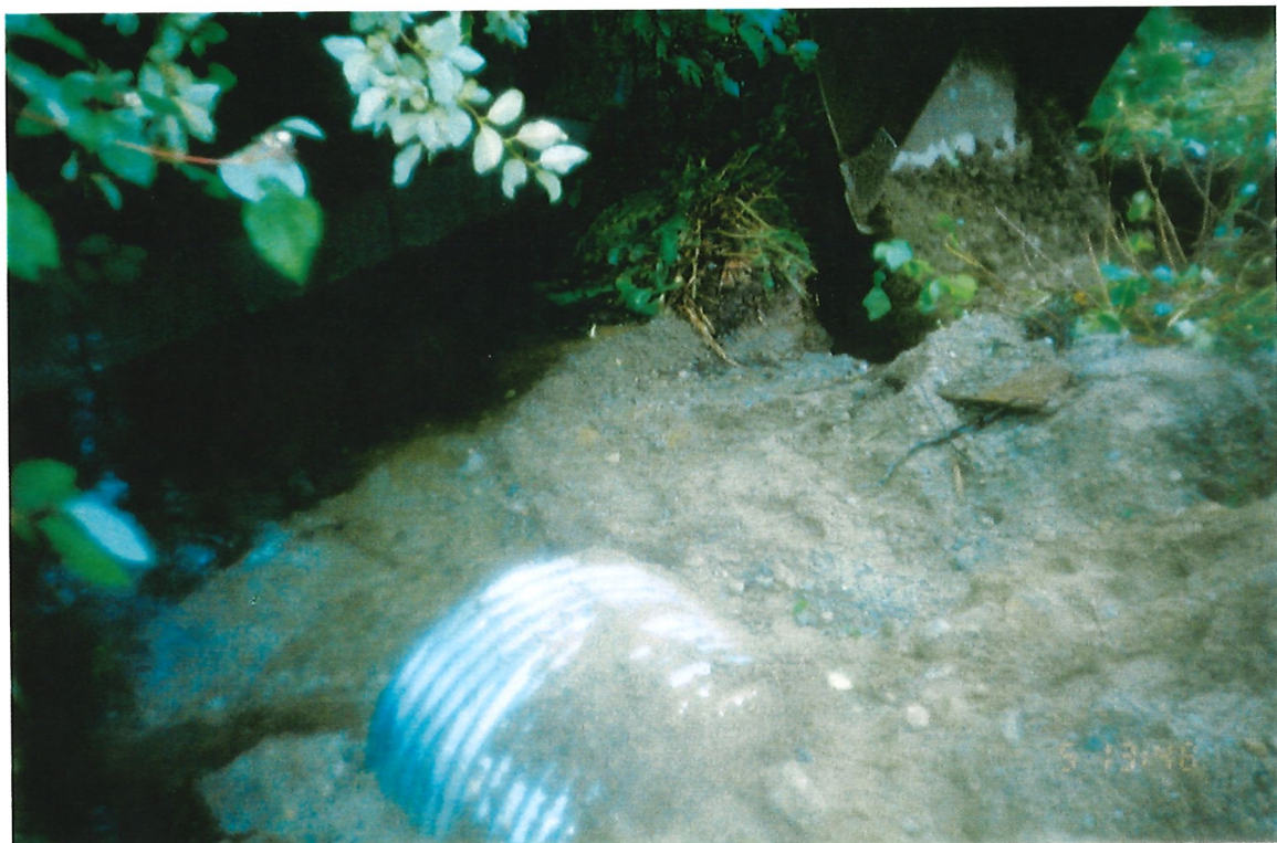
Photo 6B-10 Backfilling upstream sump.
