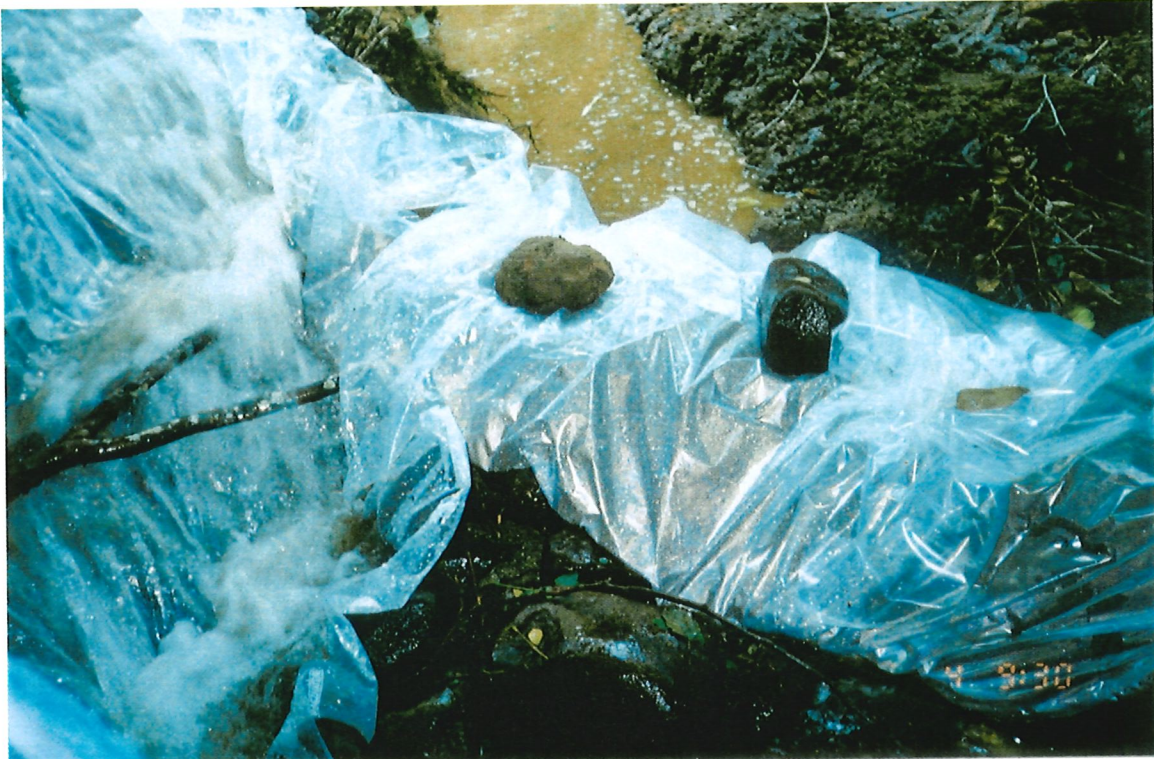
Photo 6-5 Photo of downstream sandbag / poly plastic weir and isolated dirty water within trench after culvert removal. Poly / boulder diffuser at left of picture.
