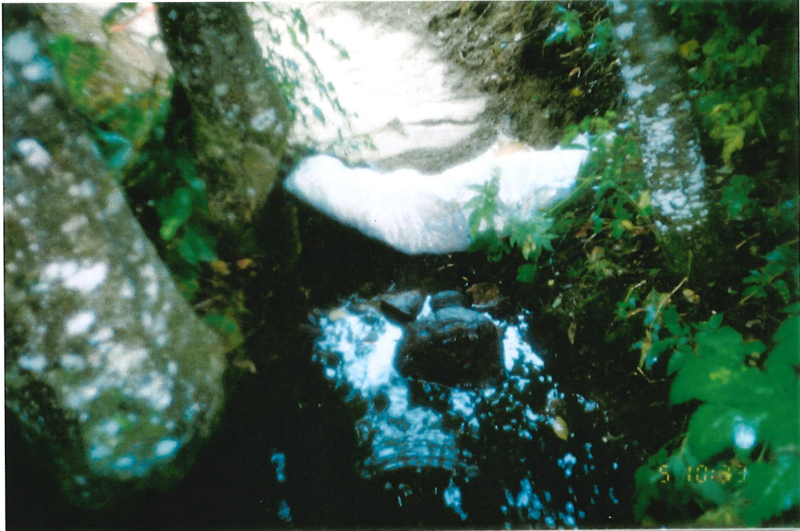
Photo 6B-3 Sandbag / poly weir at downstream end of site.
