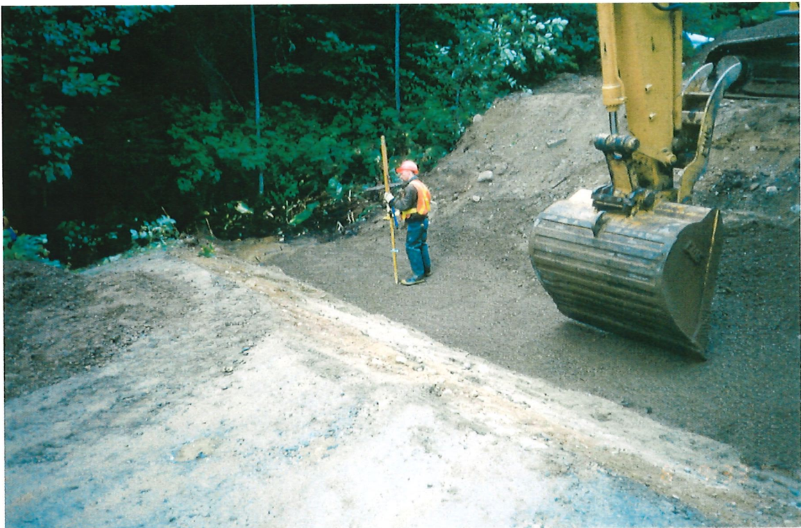
Photo 5-4 Leveling culvert bed to grade.
