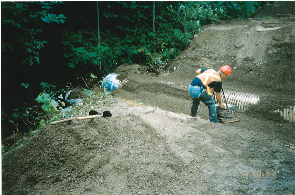
Photo 5-6 Compacting fill around culvert.
