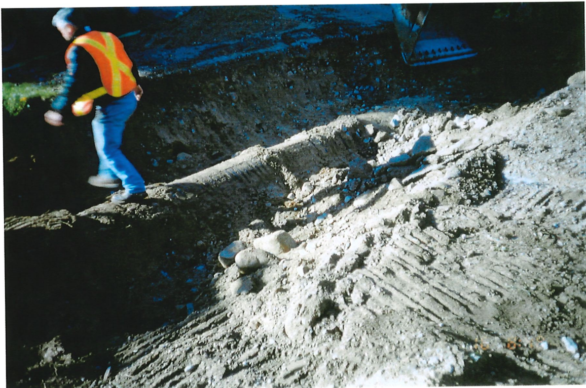
Photo 16-2 Excavating down to existing culvert.
