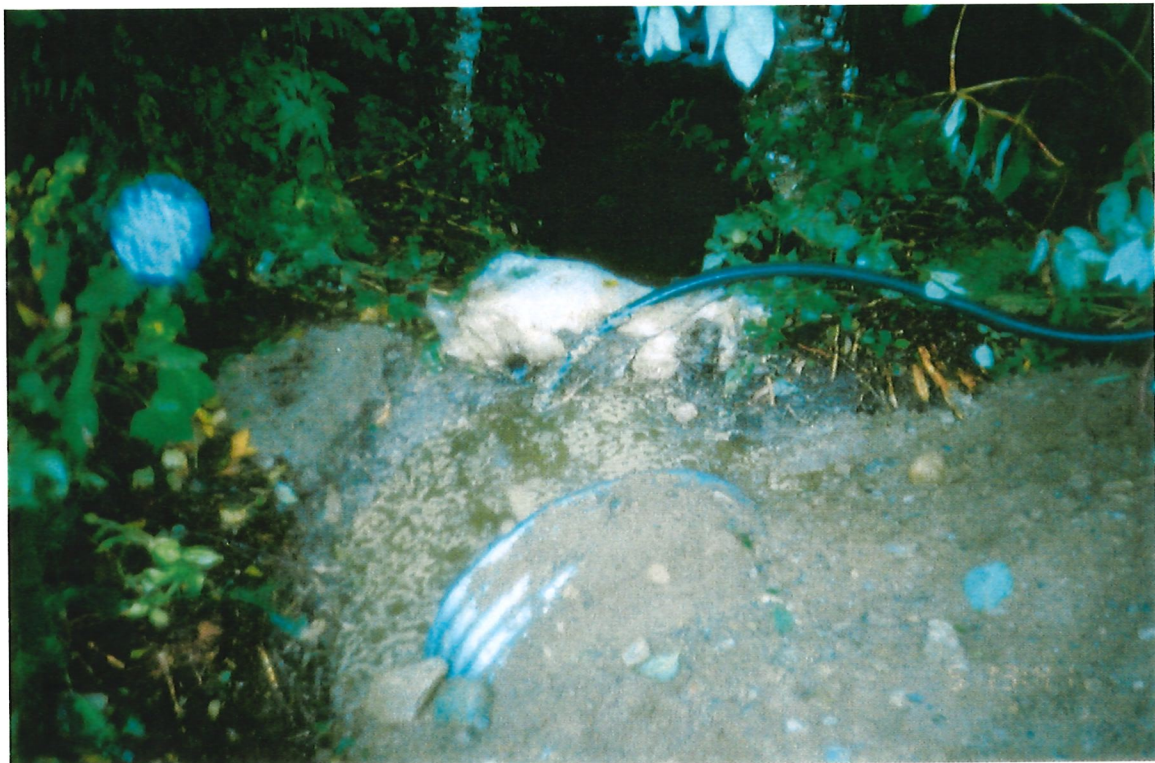
Photo 6B-8 Flushing of culvert to remove fines from fill materials. Dirty water was pumped into adjacent vegetation.
