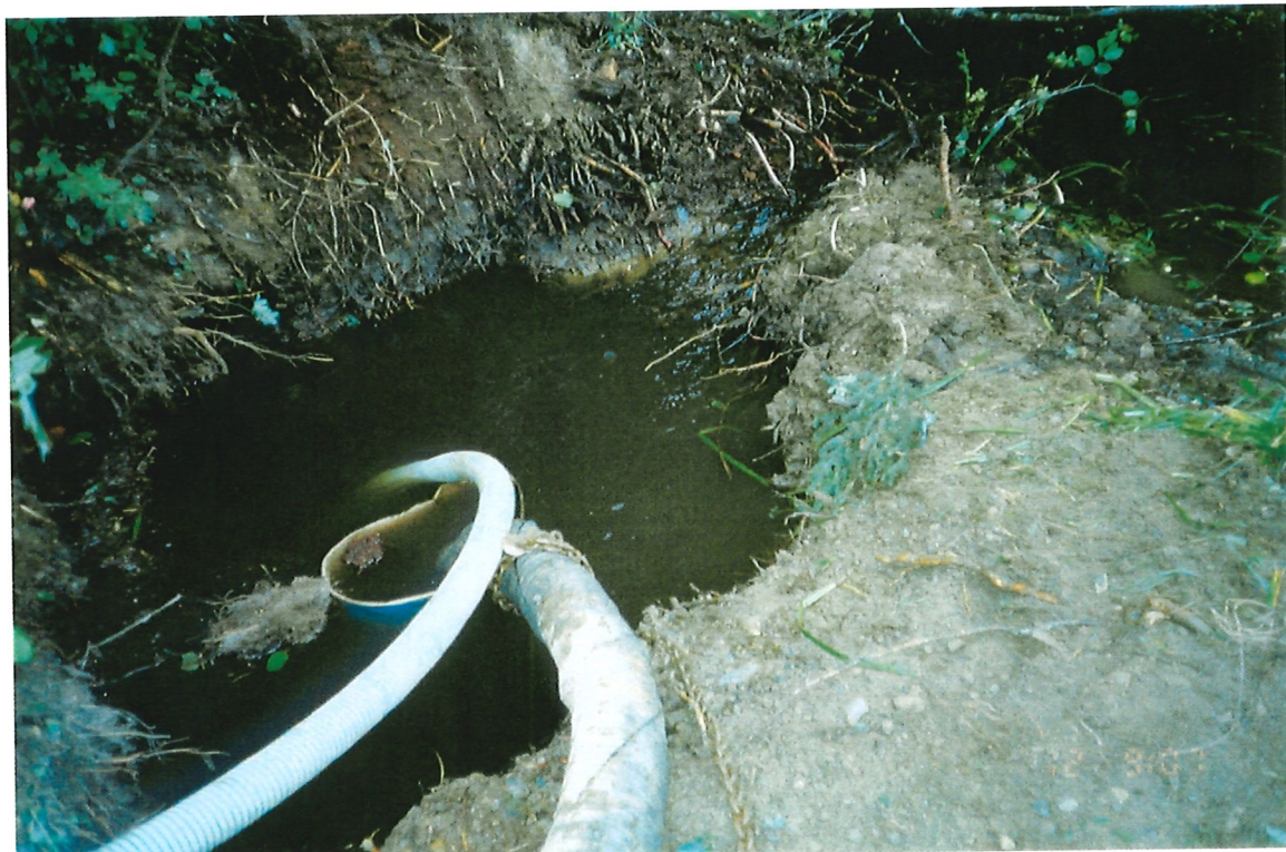
Photo 12-2 Filling upstream sump prior to diversion. Note 3" pump for removing dirty water
