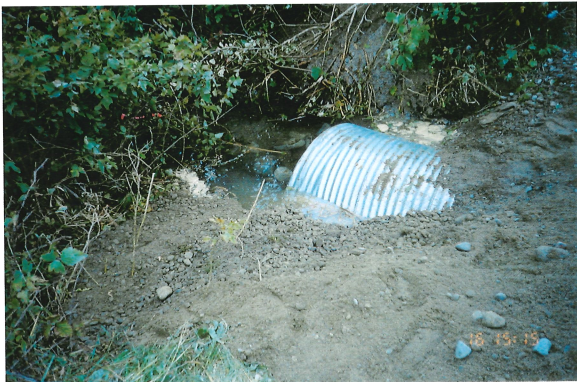
Photo 16-8 Photo of outlet immediately after breach of upstream weir.
