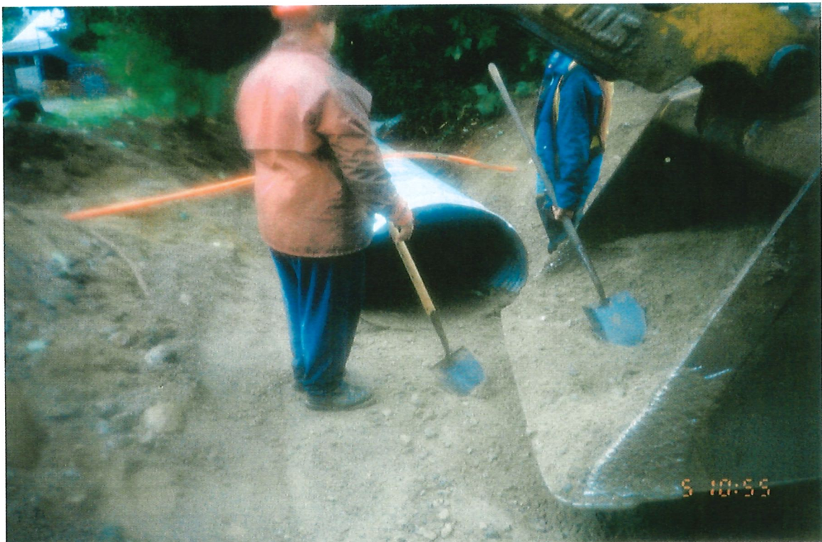
Photo 6B-6 Crew filling culvert with approved fisheries gravel.
