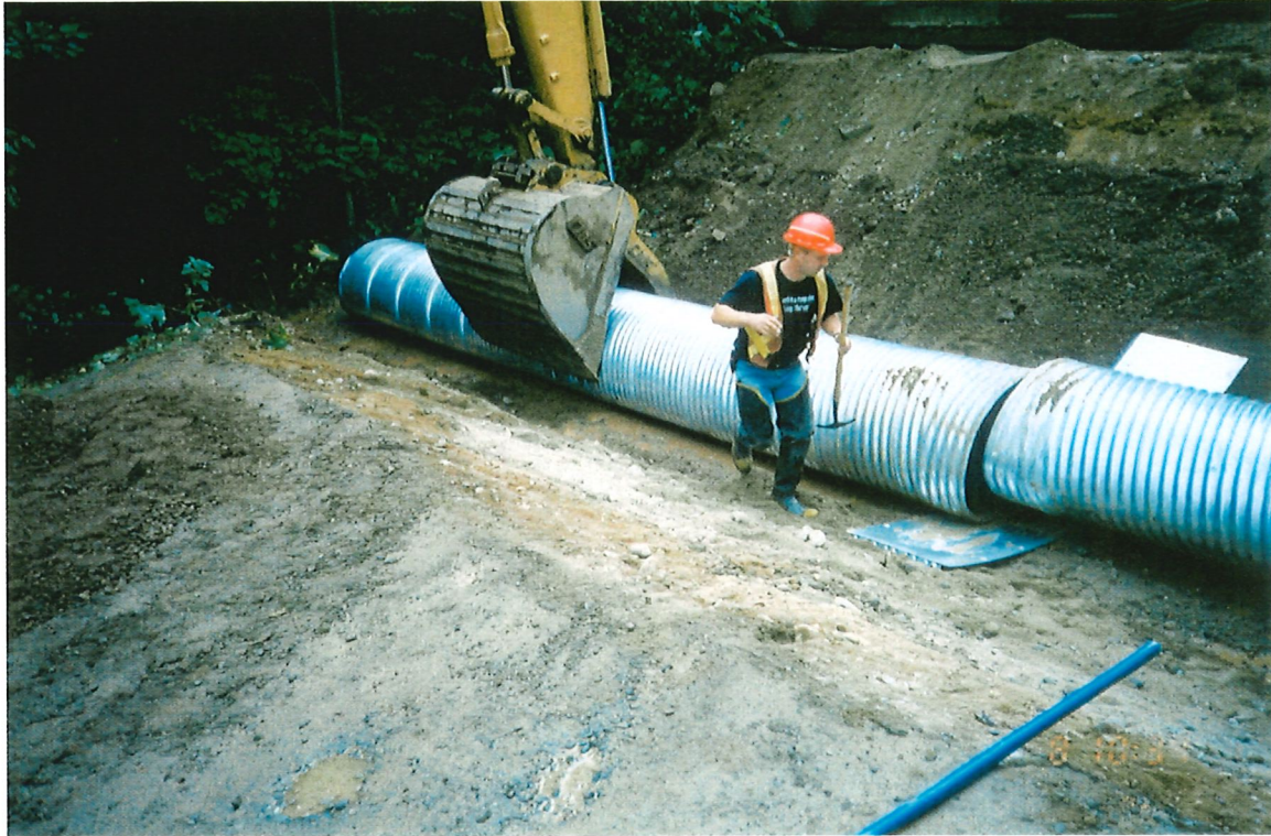
Photo 5-5 Aligning upper and lower sections of culvert prior to collaring.
