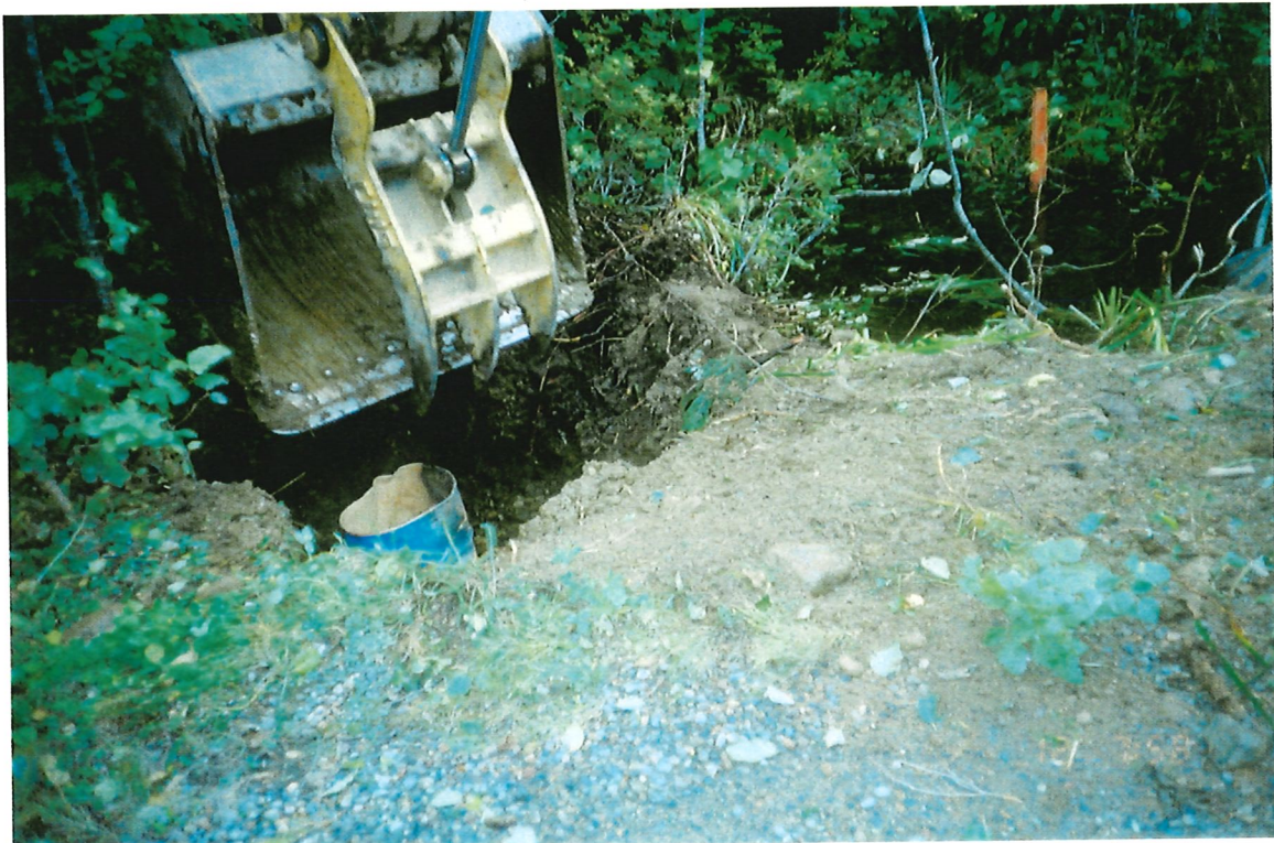
Photo 12-1 Placing sump adjacent to stream.
