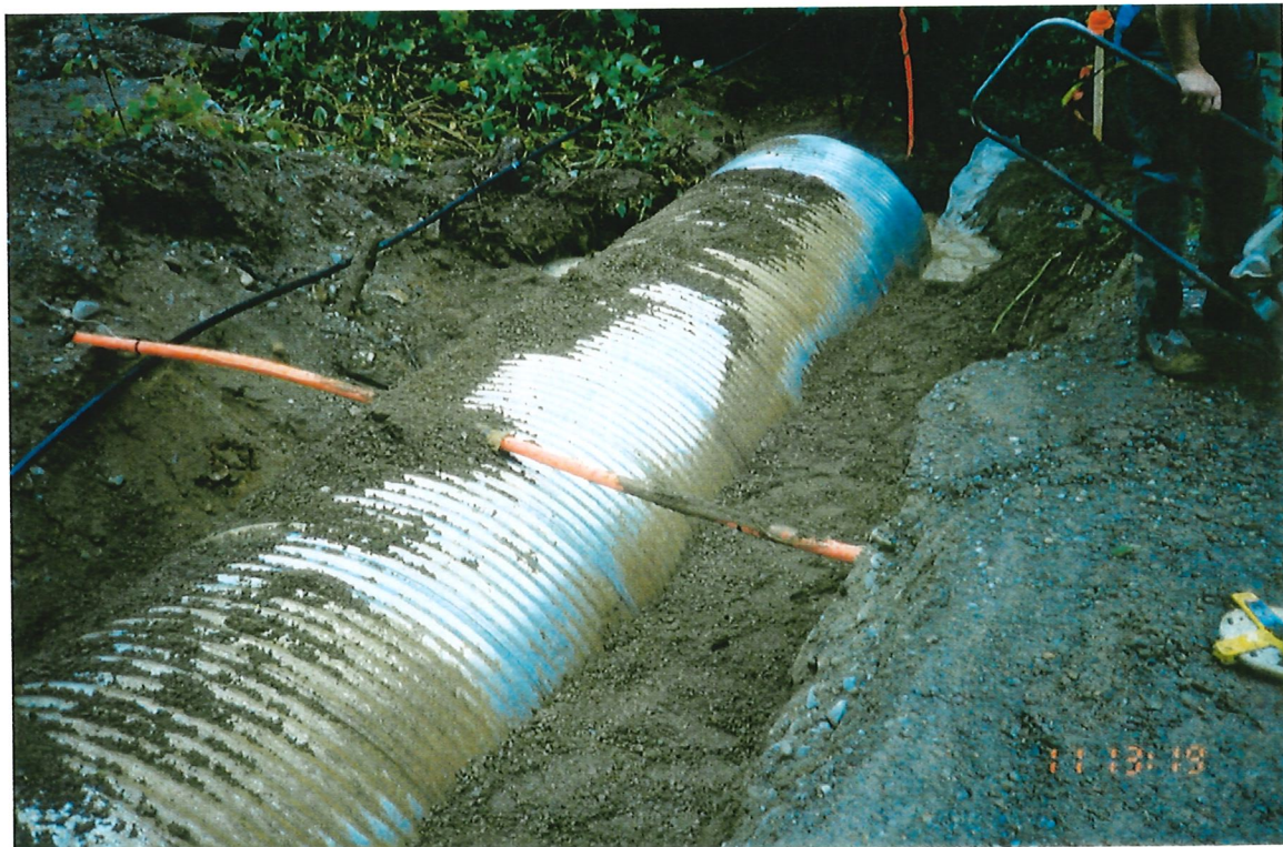
Photo 10-6 Backfilling and compacting around culvert.
