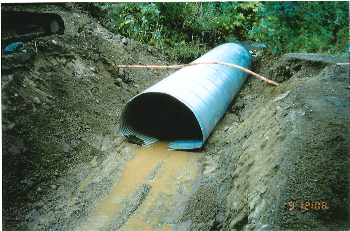
Photo 9-2 Downstream section of culvert being installed under natural gas line.
