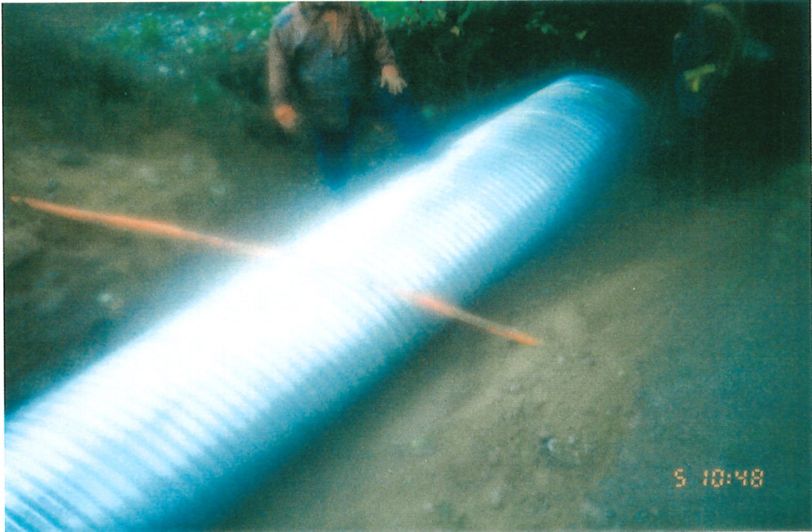
Photo 6B-5 Placing culvert under natural gas line.
