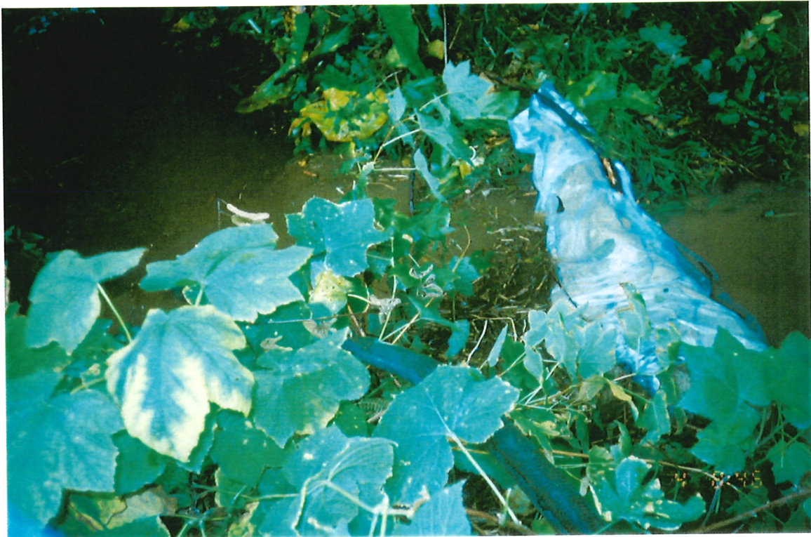
Photo 6-3 Upstream sandbag / poly plastic dam.
