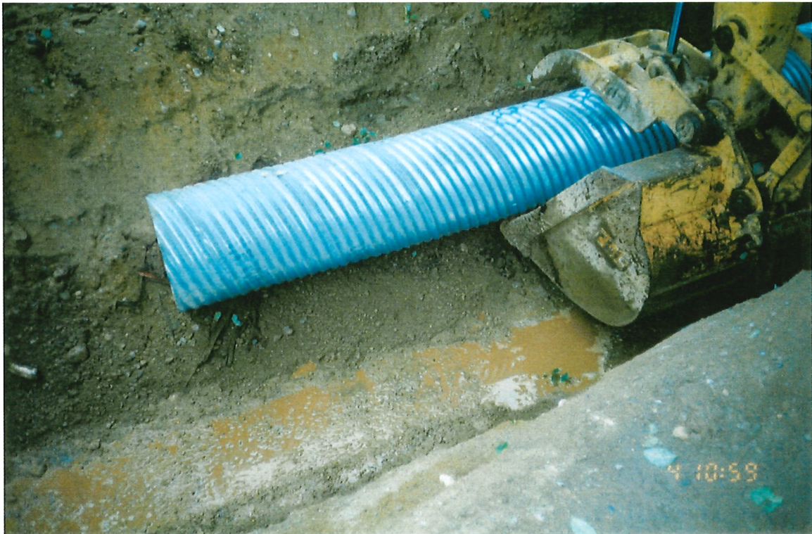
Photo 6-7 Laying new section of culvert in trench.
