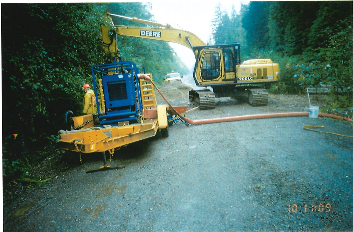
Photo 9-7 Flight pump and excavator used for 1 st Avenue installations.
