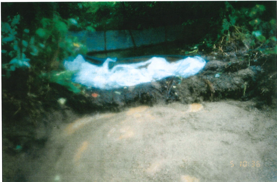
Photo 6B-4 Sandbag / poly weir at upstream end of site and fish exclusion fence in background.
