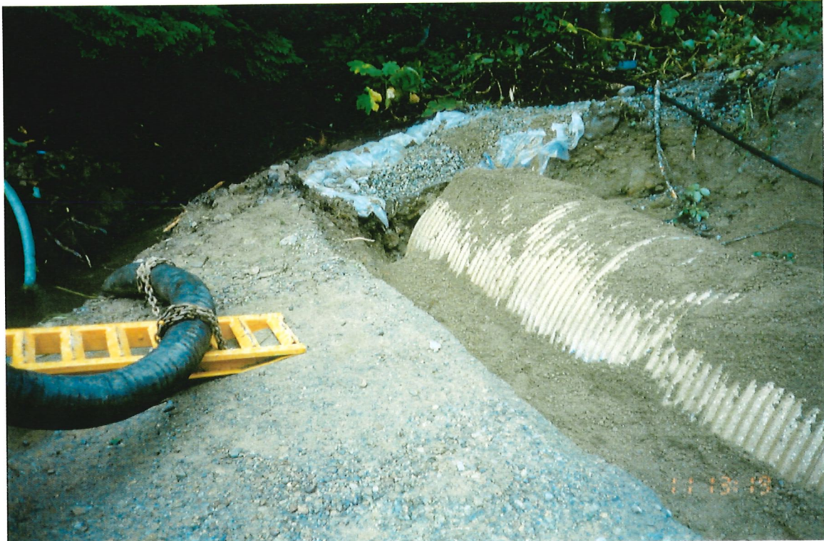
Photo 10-5 Backfilling around culvert.
