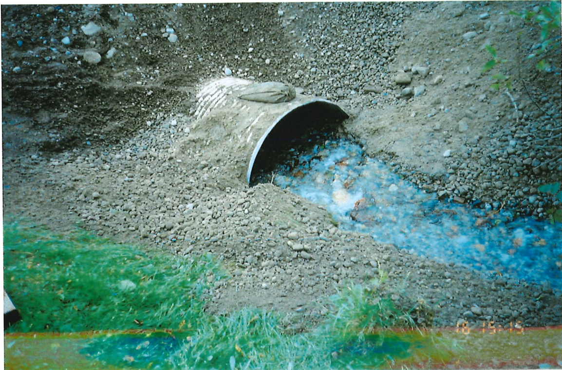
Photo 16-7 Photo of inlet immediately after breach of upstream weir.
