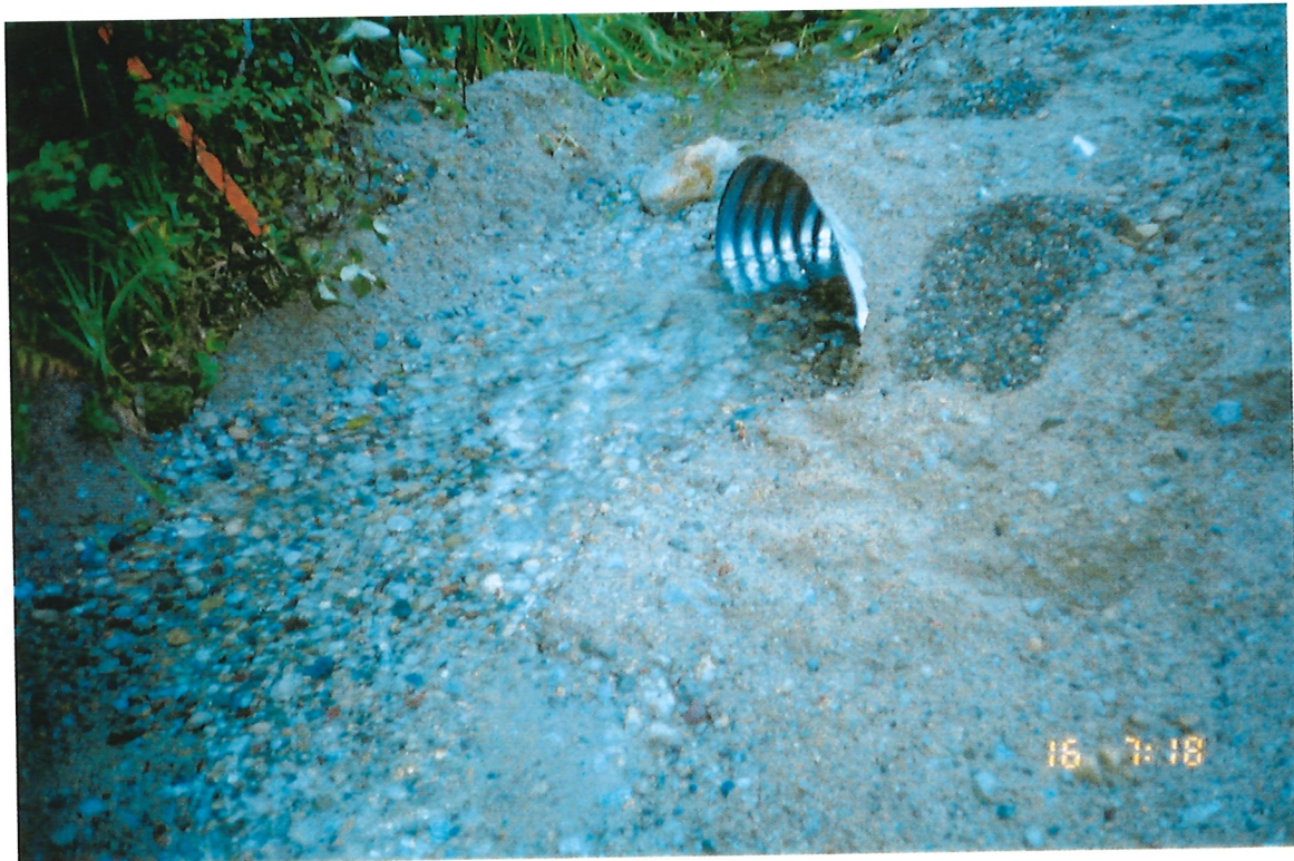
Photo 14-2 Culvert inlet.
