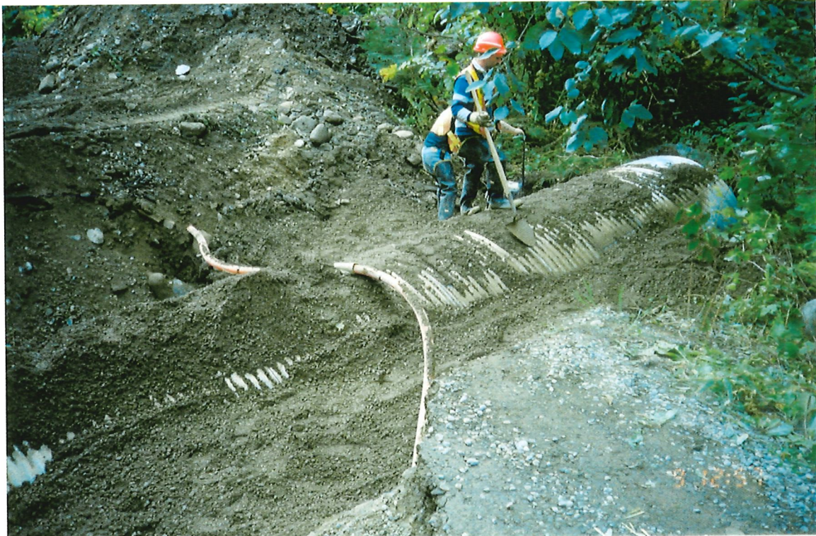
Photo 9-5 Compacting gravel around culvert.
