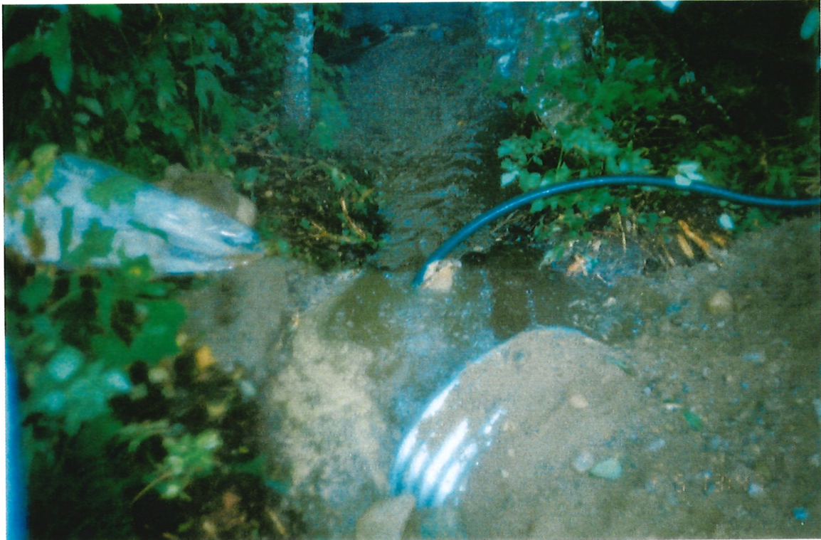
Photo 6B-9 Full breach of upstream weir and removal of downstream weir.
