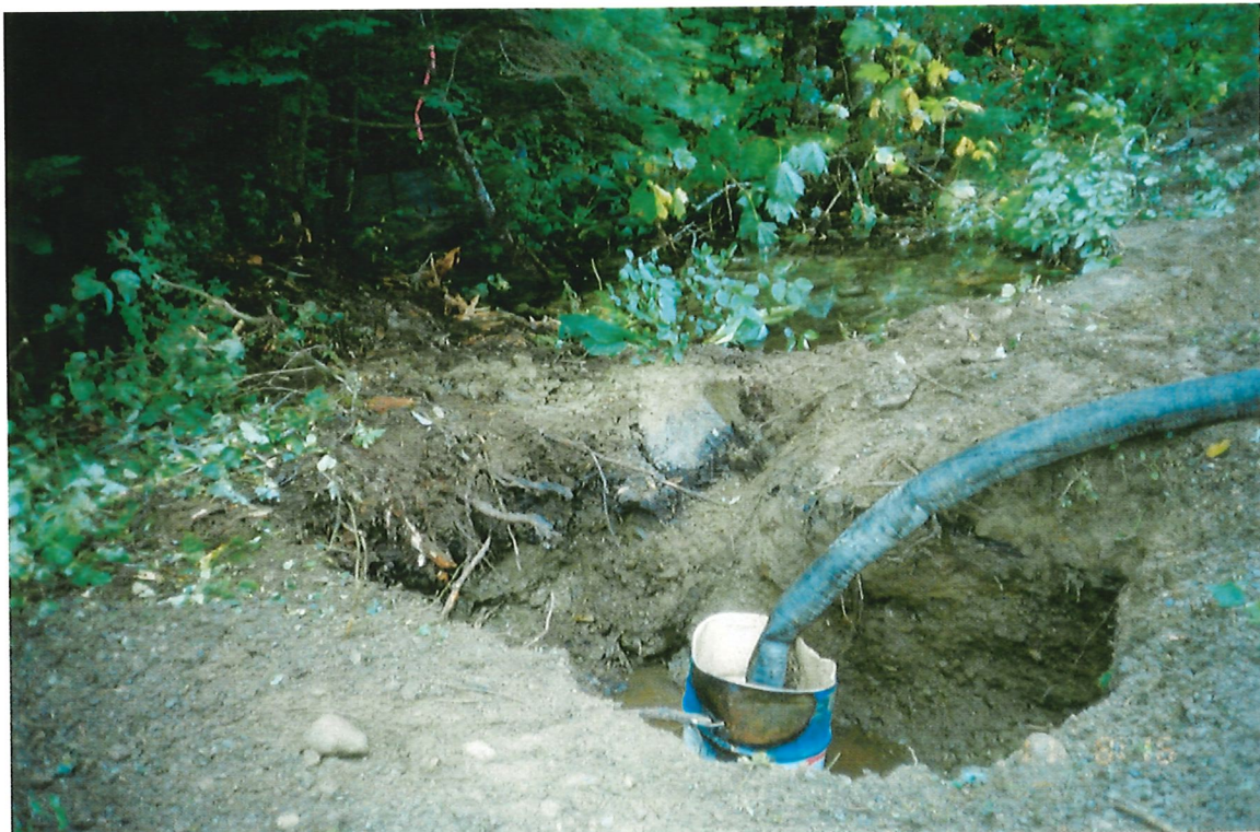
Photo 10-2 Sump at upstream end of culvert prior to filling.
