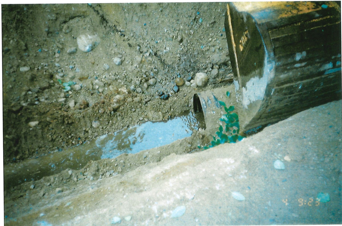
Photo 6-4 Excavating existing culvert.
