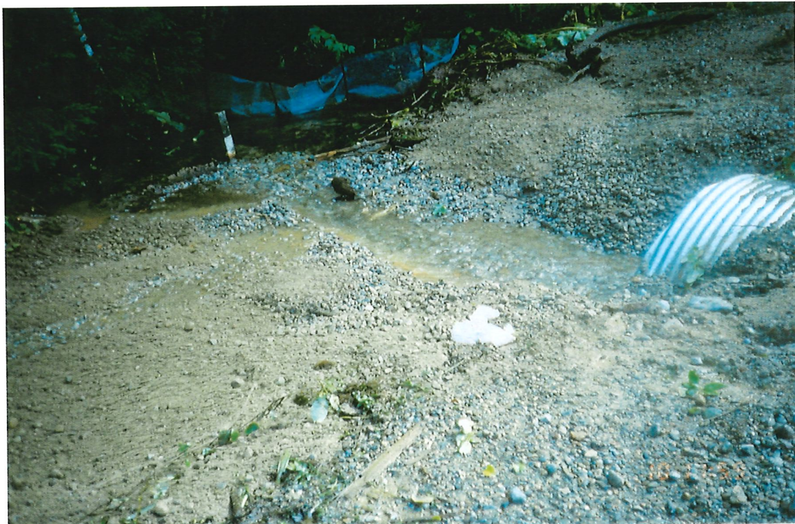
Photo 9-10 Photo of culvert inlet after full breach and sump infill.
