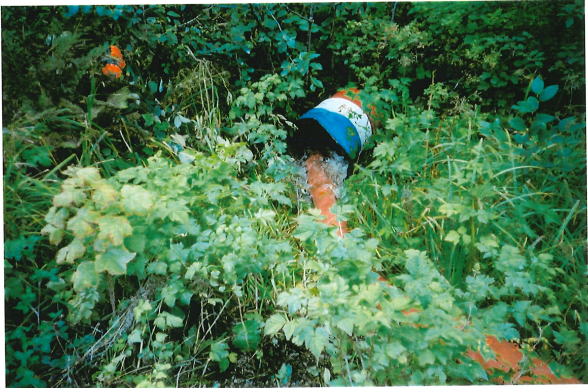
Photo 12-3 Diffuser at end of diversion hose.
