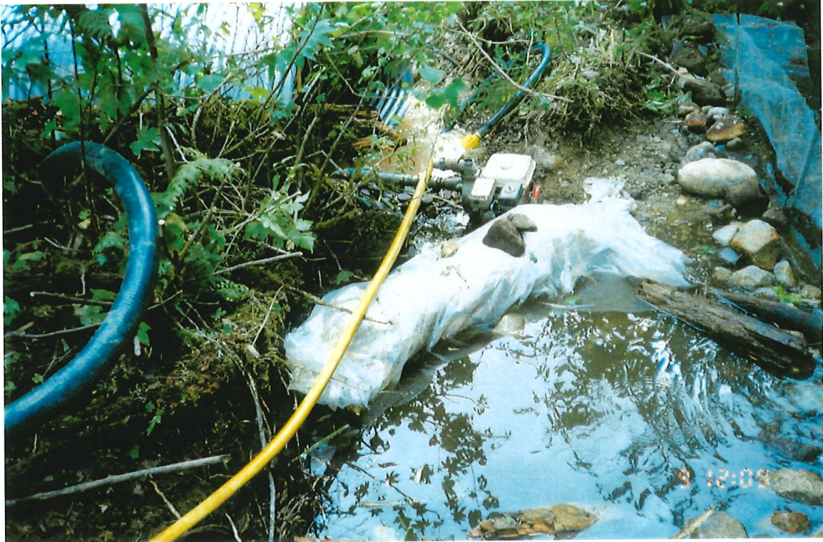
Photo 9-3 Sump with pump and sandbag / poly weir at outlet of culvert.
