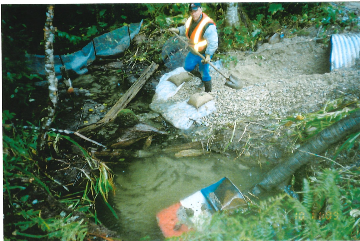
Photo 9-8 Partial breach of upstream weir for culvert cleanse.
