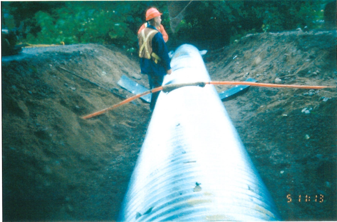
Photo 6B-7 Crew collaring culvert and wrapping natural gas line prior to backfilling.
