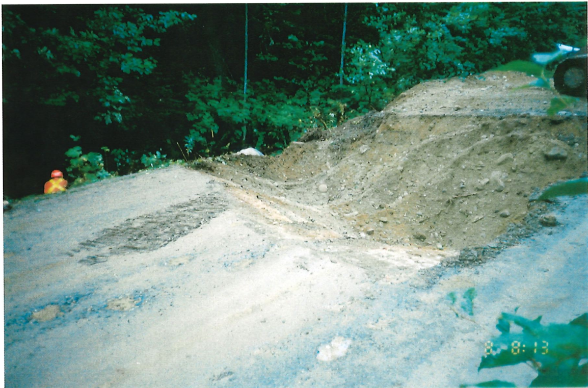
Photo 5-2 Excavating roadbed.
