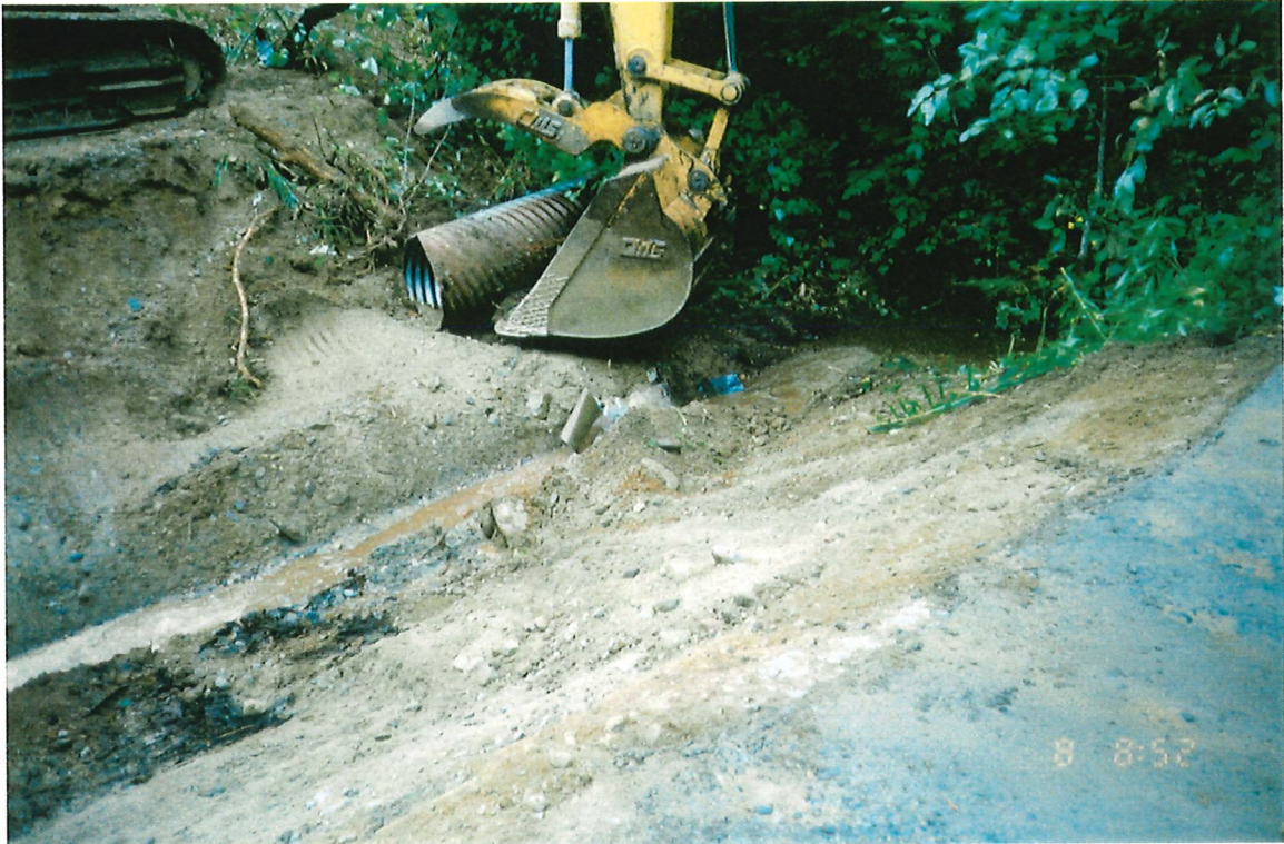
Photo 5-3 Removing existing culvert from trench.
