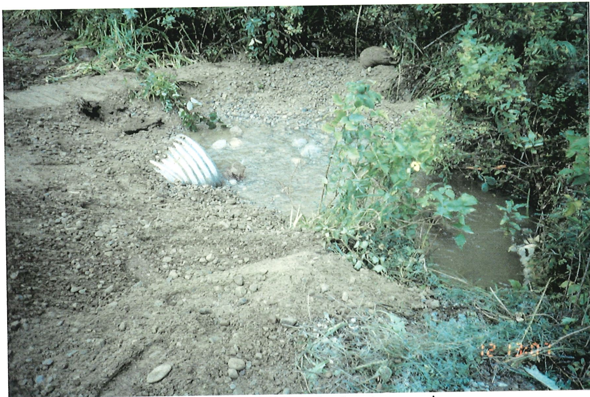
Photo 12-6 Water out of culvert after full breach of upstream weir.
