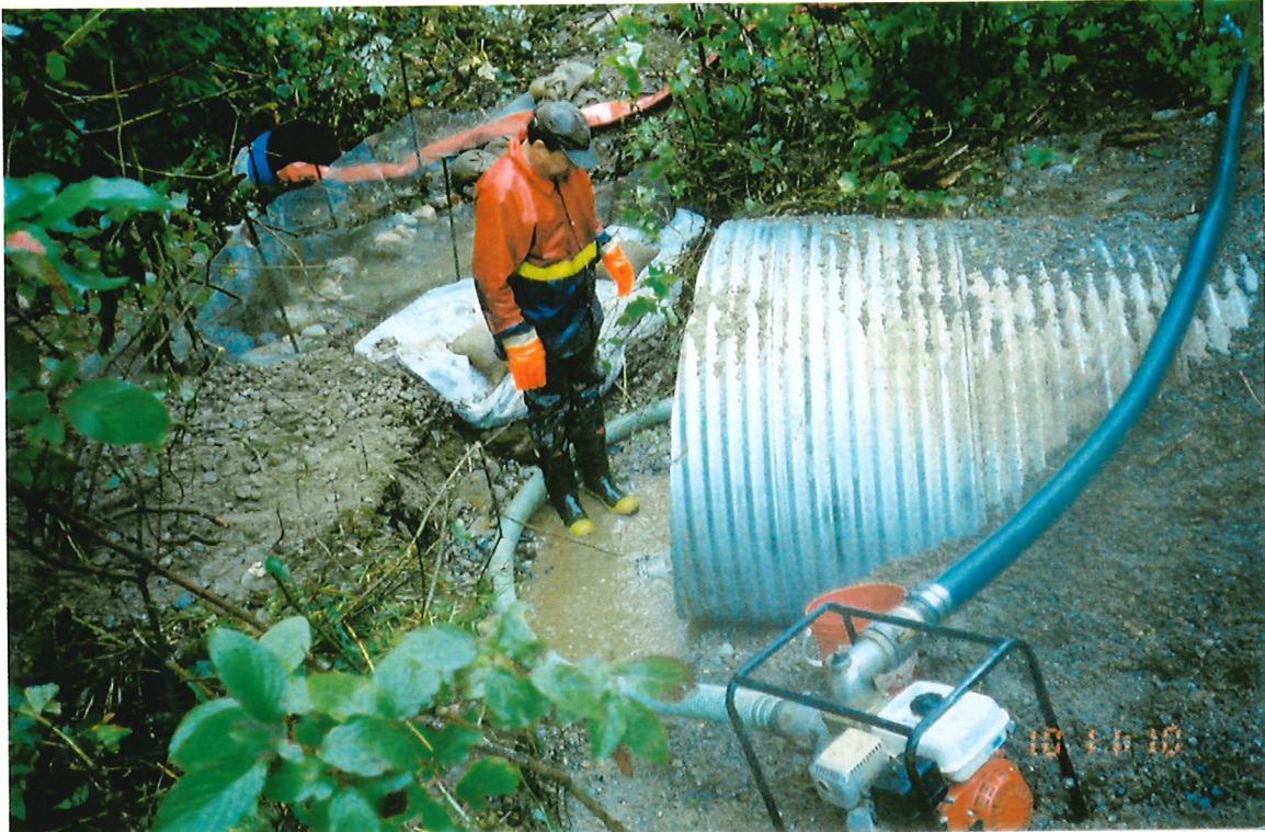
Photo 9-9 Removing dirty water from lower sump during culvert cleanse.
