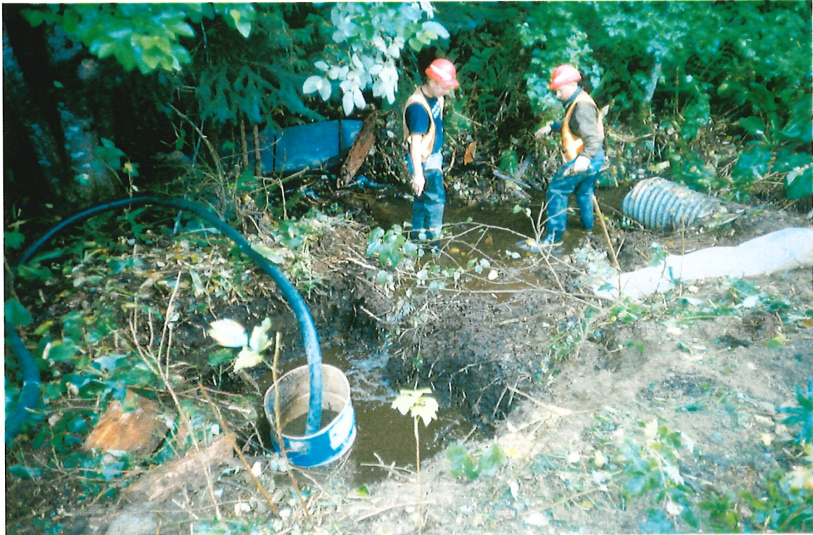
Photo 5-1 Crew filling sump at upstream end of culvert.
