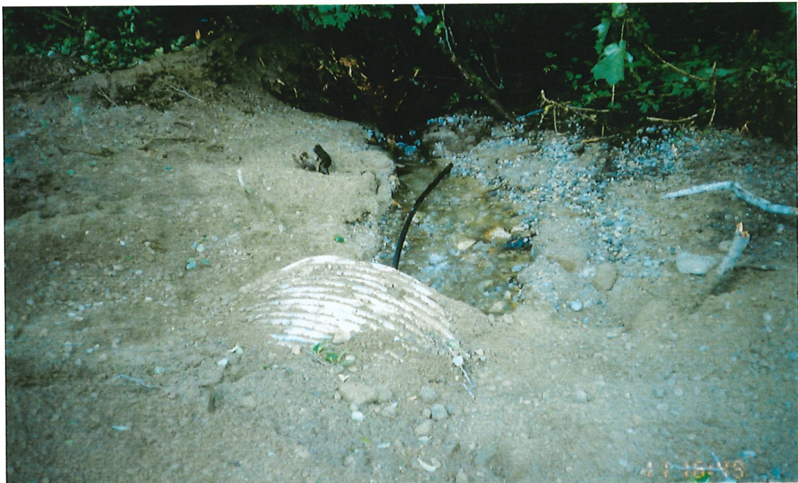
Photo 10-7 Outlet of culvert showing local water intake hose running up and through culvert.
