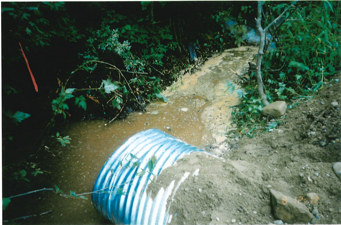
Photo 5-7 Flushing of culvert to remove fines from culvert infill materials. Dirty water pumped into adjacent vegetation.
