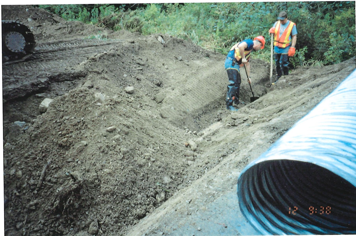
Photo 12-4 Crew searching for gas line in culvert trench.
