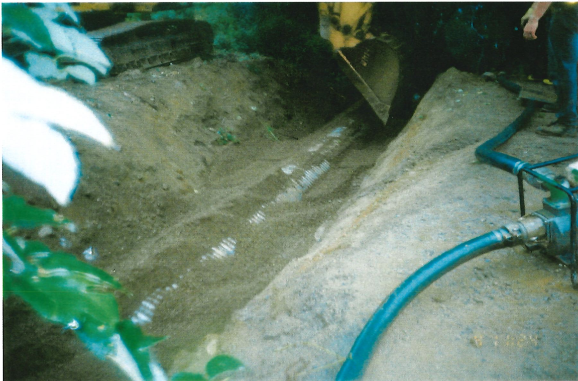
Photo 6-8 Back-filling new culvert.
