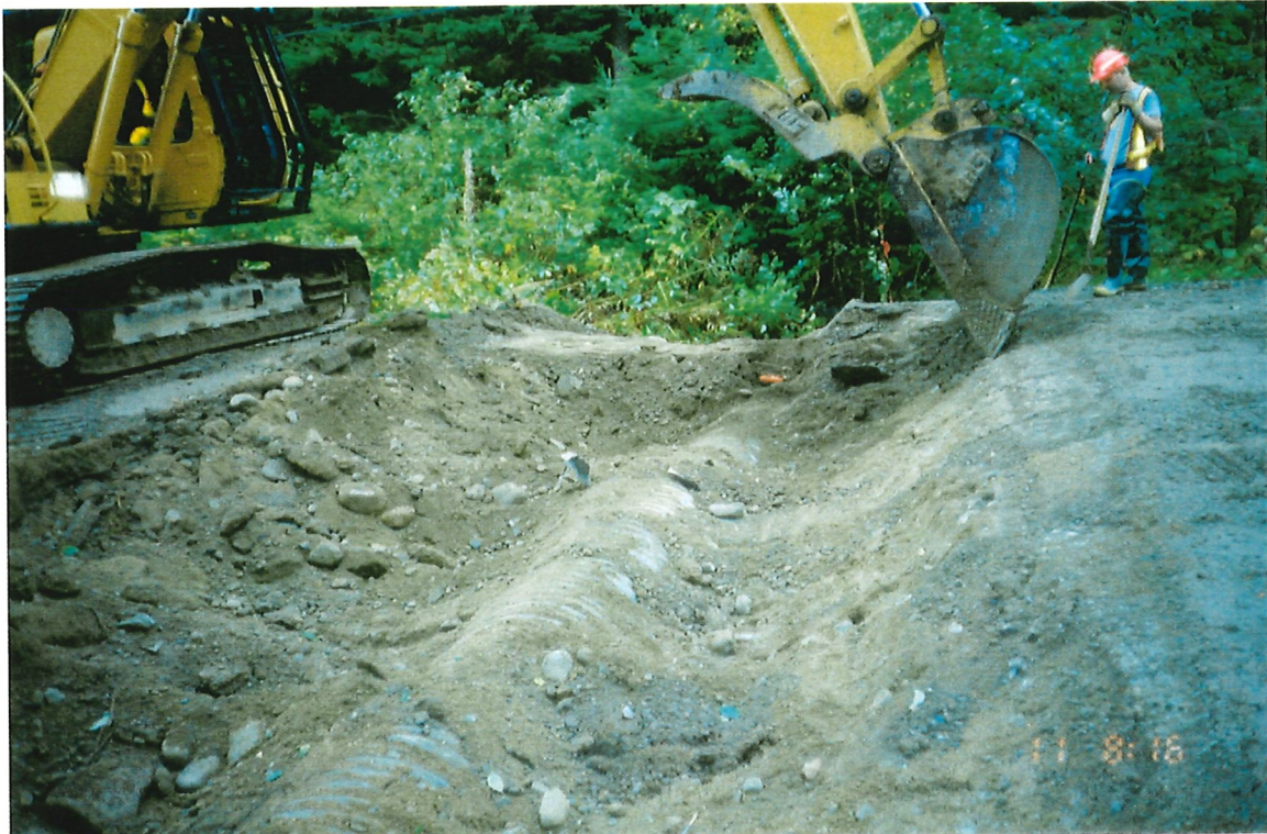
Photo 10-3 Excavating around natural gas line.
