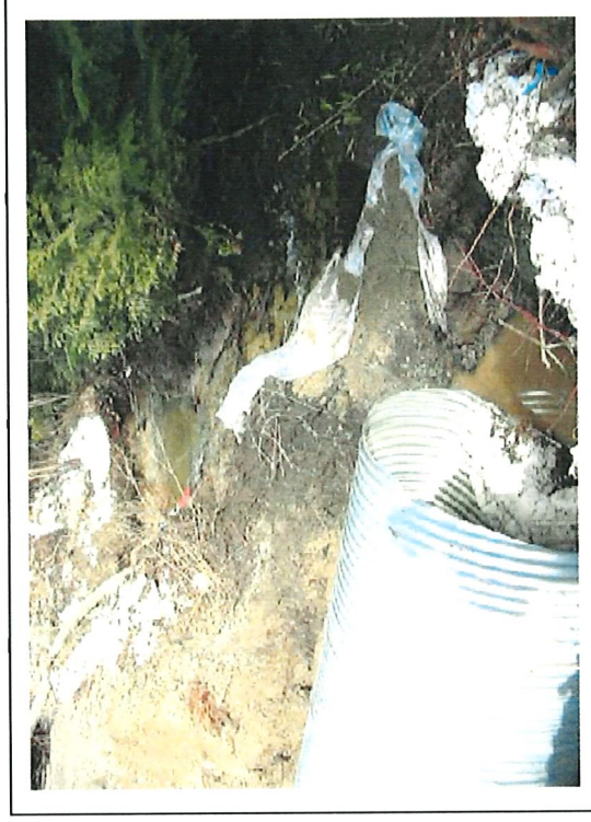
Culvert inlet prior to backfilling.
