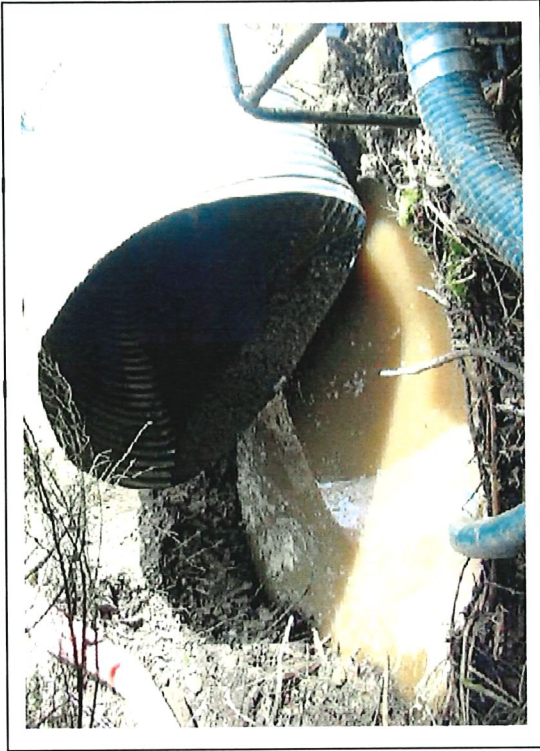
Infill substrates were flushed with water prior to re directing stream flow through the new culvert.
