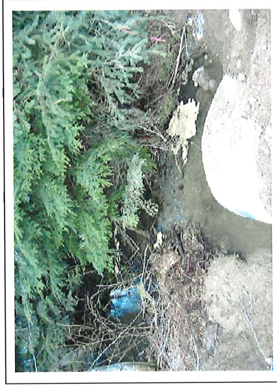
Infill substrates were flushed with water prior to re directing stream flow through the new culvert.
