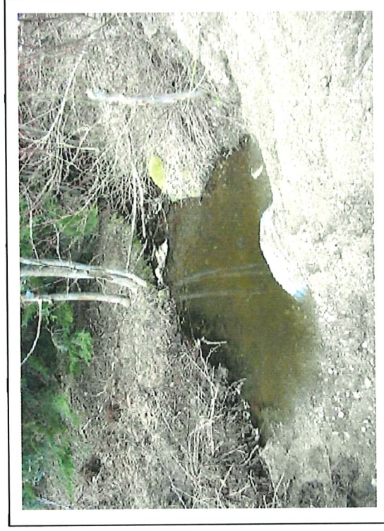
Culvert outlet post construction.
