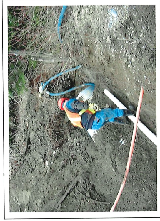
Culvert was backfilled with gravel material.
