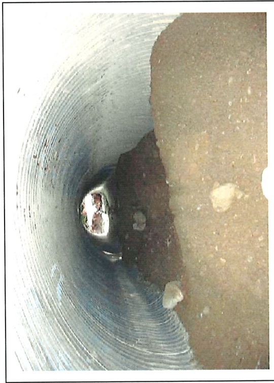
Culvert was filled with gravel and cobble substrates.
