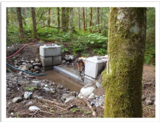
Photo 13: Installing lock block weir sill
