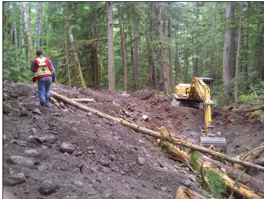
Photo 3 – June 22, 2012 – Channel construction near the log jam.
