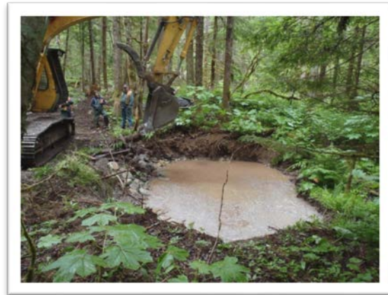
Photo 9: Excavation for placement of lock block weir
