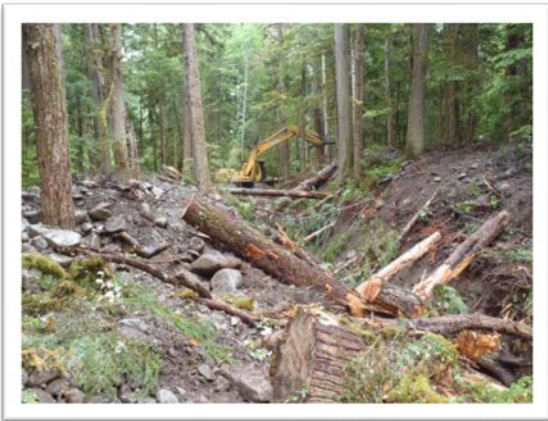
Photo 5: Continued channel excavation
