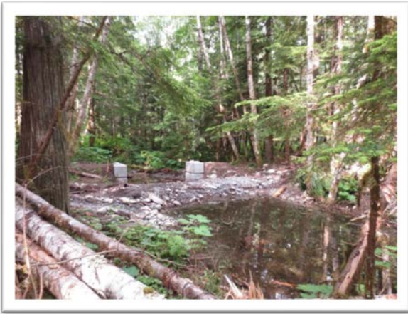
Photo 12: Looking downstream from 2011 channel towards lock block weir
