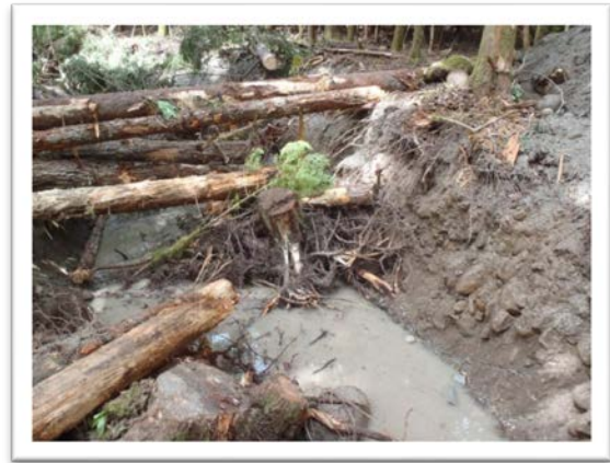
Photo 2: Newly excavated channel
