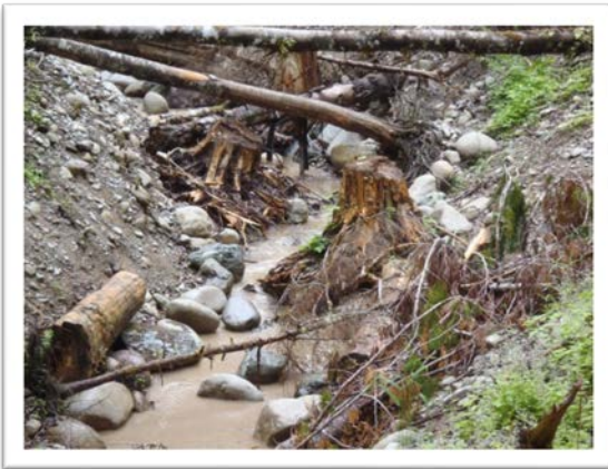
Photo 8: Typical excavated channel
