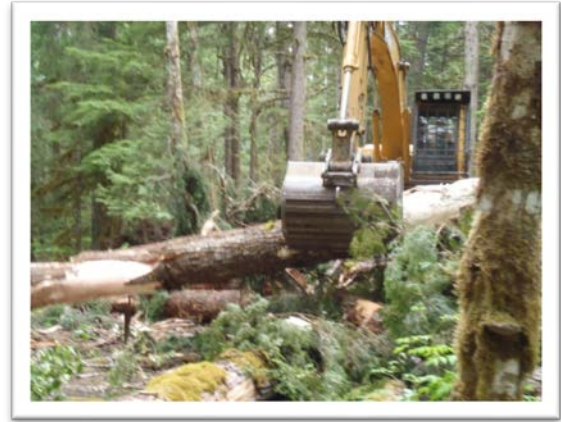
Photo 4: Removing logs from natural channel
