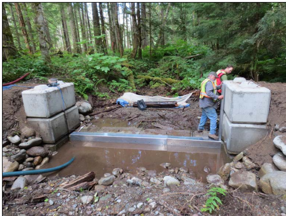
Photo 5 – August 2, 2012 – Installing the metal edge on the sill.
