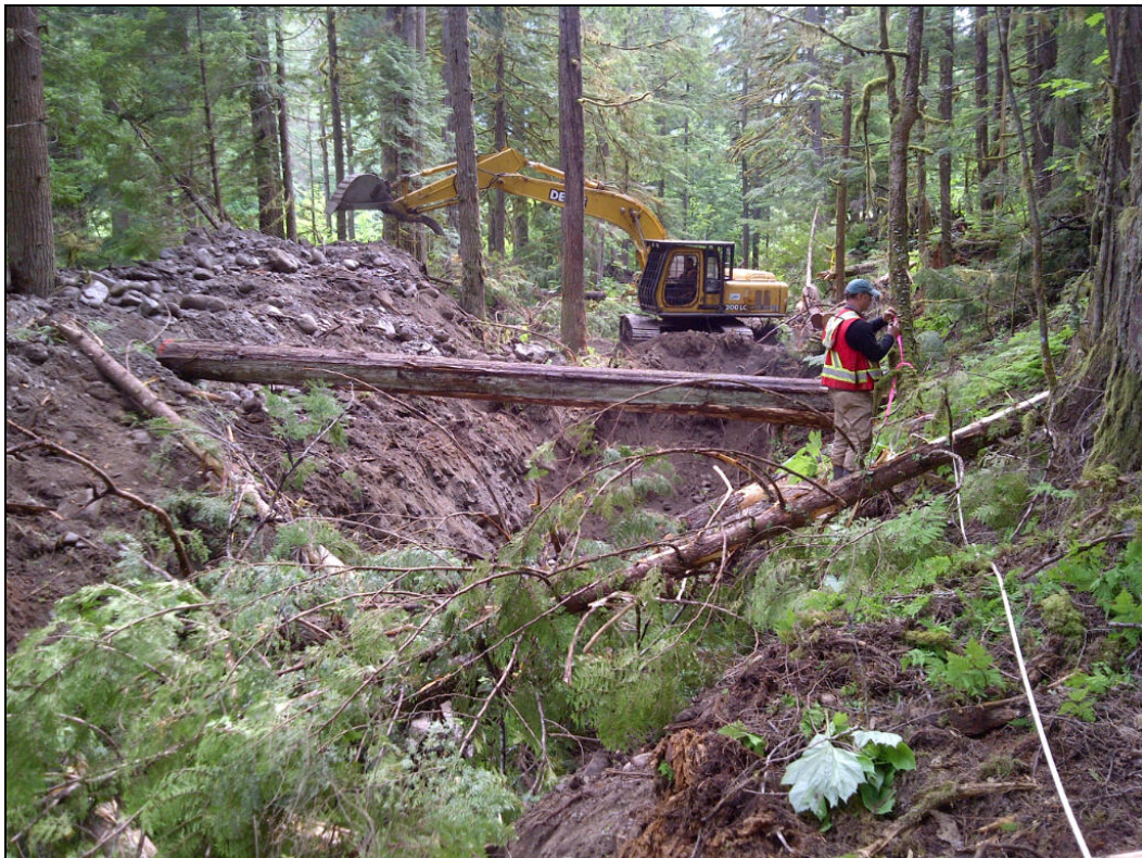
Photo 2 – June 25, 2012 – Typical channel construction
