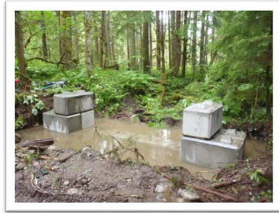
Photo 11: Completed lock block weir
