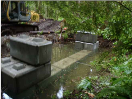
LOCK BLOCK WEIR
