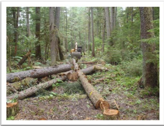
Photo 1: Clearing the channel route
