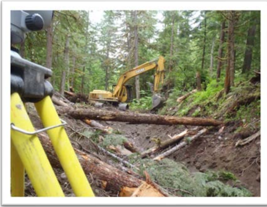
Photo 6: Continued channel excavation
