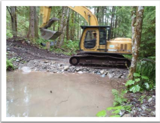
Photo 10: Lock block weir excavation continued
