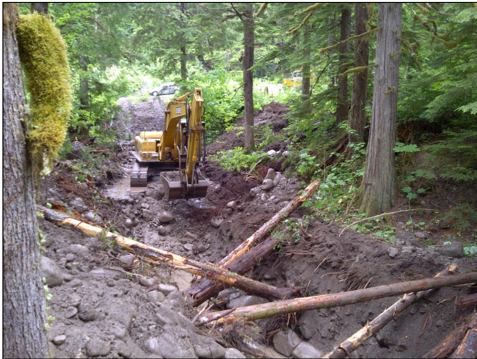
Photo 4 – June 27, 2012 - Approaching the end of the open channel.
