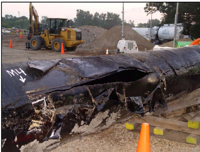
Figure 53. Enbridge pipeline rupture , Kalamazoo River, 2010. Courtesy of the US National Transportation Safety Board.
