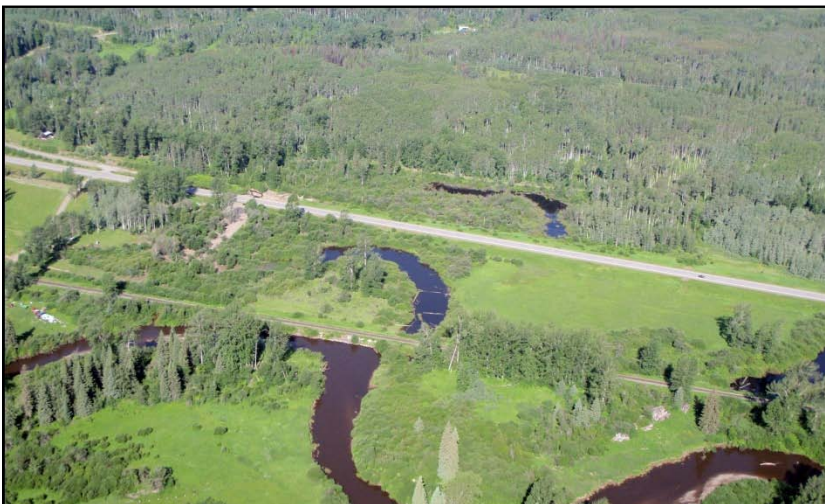
Figure 42. Upper Bulkley River floodplain bisected by CN Rail, Highway 16, and diminished riparian zones.
