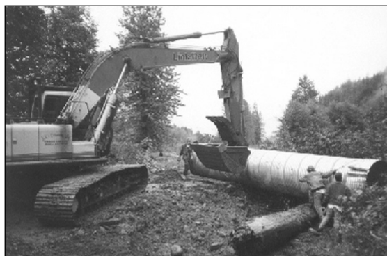
Figure 6-38. Installation of new 1500 mm culvert.
