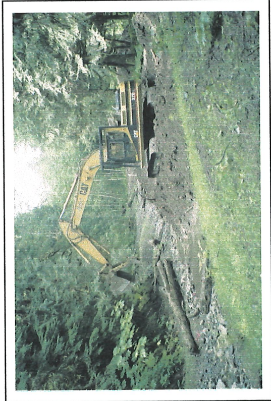
Photo 17. August 2001. 320 Caterpillar Excavator digging the head pond (Pond 1).
