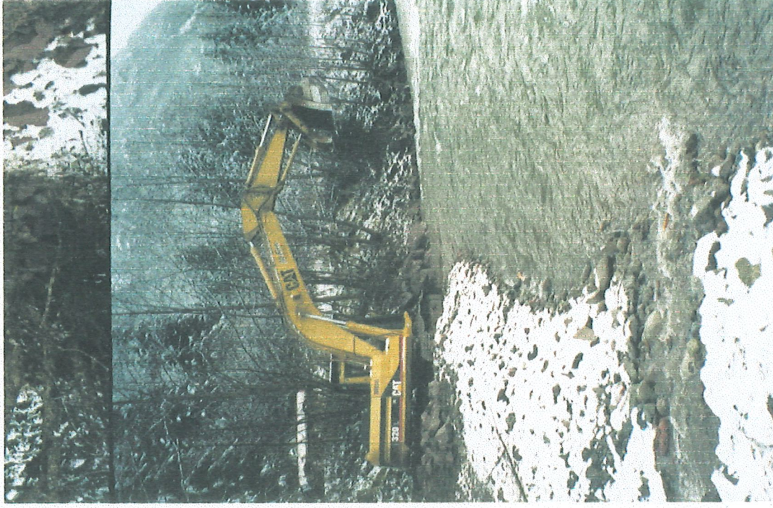
Photo 7. November 2001. Looking downstream along the Copper River at the excavator placing rip rap along the toe of the road. The old outlet channel is in the foreground.
