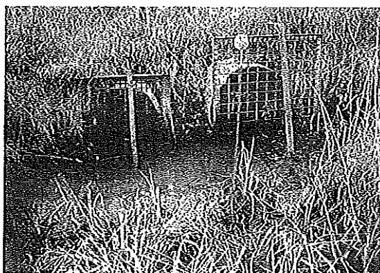
C: Upstream view of culverts under Highway 16. Note the screens that would prevent adult salmon migration.
