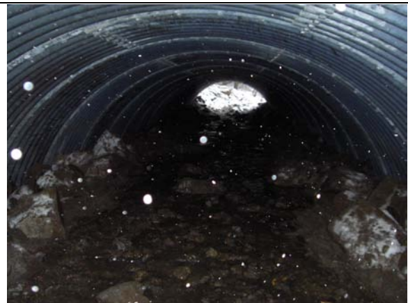
Sutherland 43km Photo 5. Finished cascade-pool morphology streambed, November 17, 2009.
