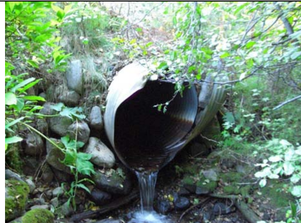
Dipper 0.7km Photo 1. Pre-existing 900mm CMP outlet, September 2009.
