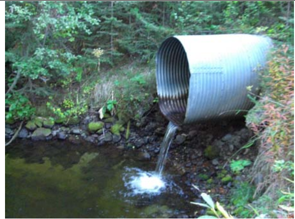
Sutherland 43km Photo 1. Pre-existing 1400mm CMP outlet, September 2009.
