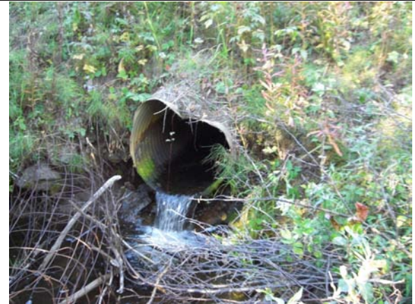
Sutherland 26.5km Photo 1. Pre-existing 800mm CMP outlet, September 2009.
