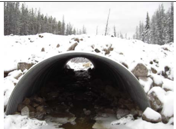
Sutherland 26.5km Photo 2. Finished riffle-pool morphology streambed, November 28, 2009.
