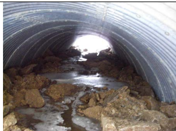
Dipper 0.7km Photo 3. Finished step-pool morphology streambed inside new arch.
