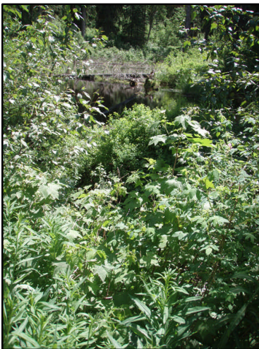
Figure 42. Site 240 culvert inlet. View upstream from inlet.
