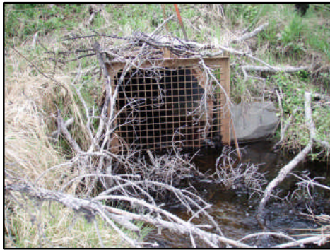
Figure 40. Site 74 culvert inlet. View downstream to inlet.
