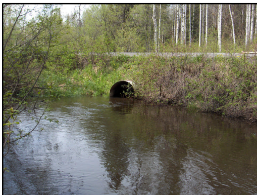
Figure 31. Kline Creek culvert outlet. View upstream to outlet.
