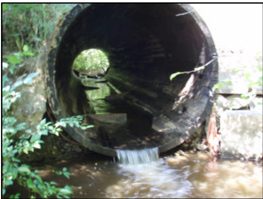
Figure 24. Murder Creek outlet. View upstream to outlet. Note the few remaining baffles.
