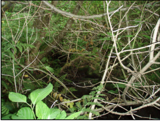
Figure 53. Site 390 culvert outlet. View downstream from outlet.
