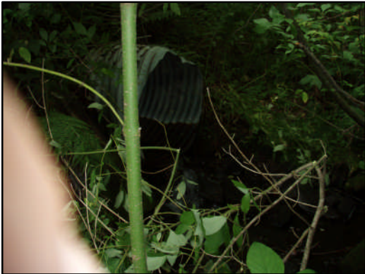
Figure 54. Site 390 culvert outlet. View upstream to outlet.
