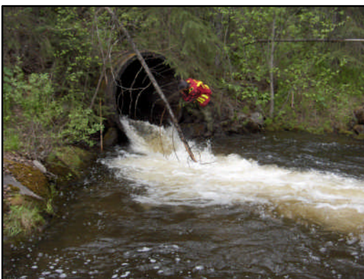
Figure 17. Skunsnat Creek culvert outlet. View of outlet from downstream.
