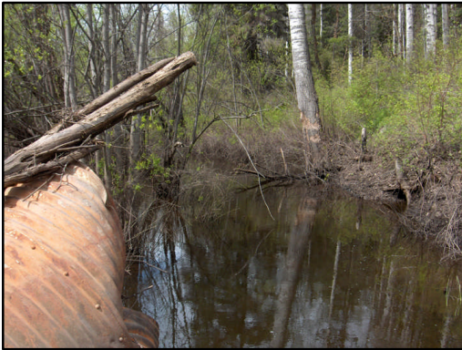
Figure 32. Kline Creek culvert inlet. View downstream of inlet.
