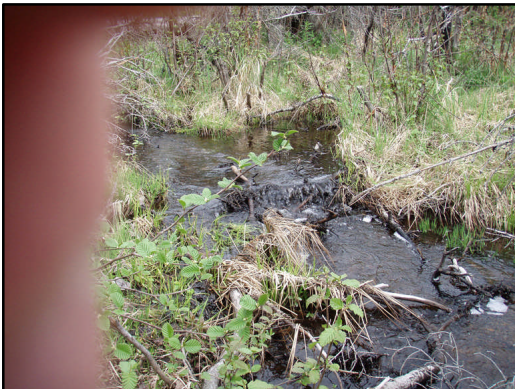
Figure 39. Site 74 culvert inlet. View upstream from inlet.
