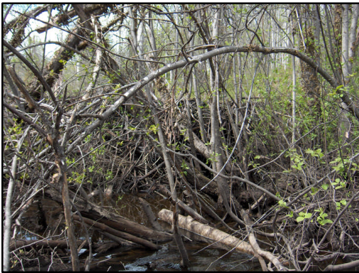
Figure 34. Kline Creek culvert inlet. View to beaver dam 29 m upstream.
