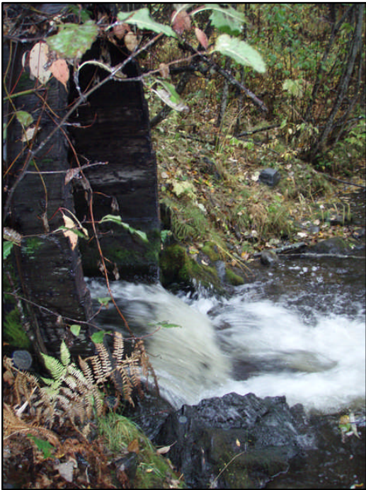
Figure 15. Clifford Creek outlet. Side view shows culvert discharge onto boulders.
