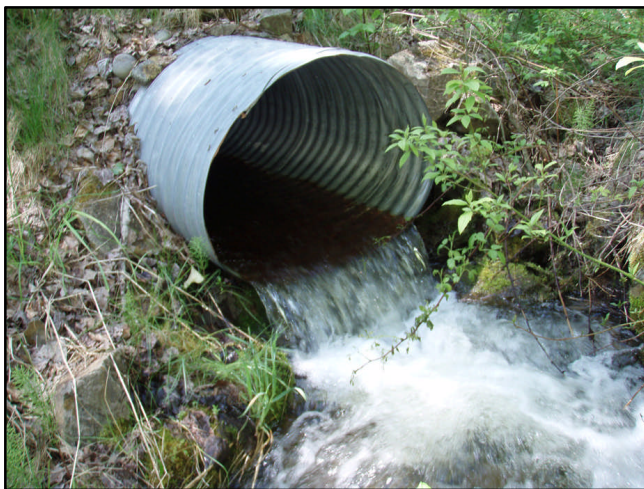
Figure 2. View upstream of Site No. 145 culvert outlet. This outfall drop is a barrier to most fish.
