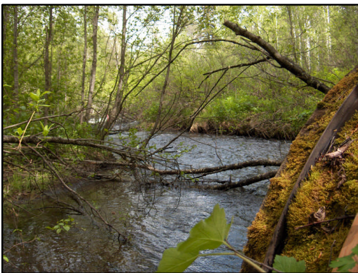
Figure 12. Clifford Creek culvert inlet View upstream from inlet.
