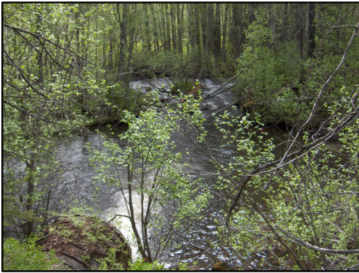
Figure 14. Clifford Creek culvert outlet. View downstream from outlet. Original channel is to the right of photo.
