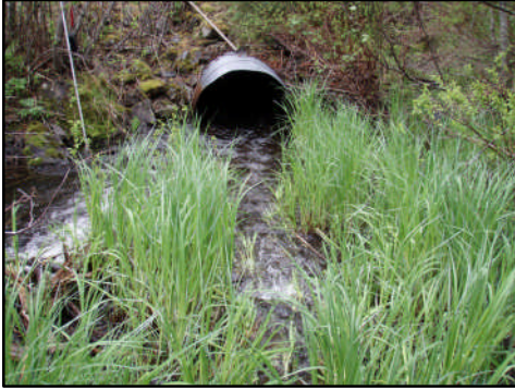
Figure 26. Hodder Creek culvert inlet. View downstream to inlet.
