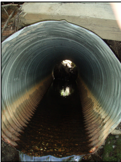
Figure 50. Site 239 culvert. View upstream through culvert.
