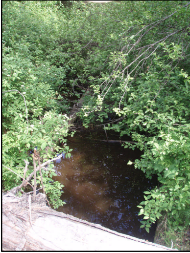
Figure 48. Site 239 culvert outlet. View downstream from outlet.
