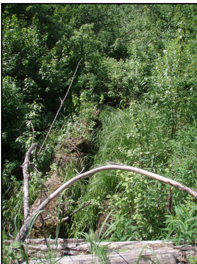
Figure 47. Site 239 culvert inlet. View upstream from inlet.
