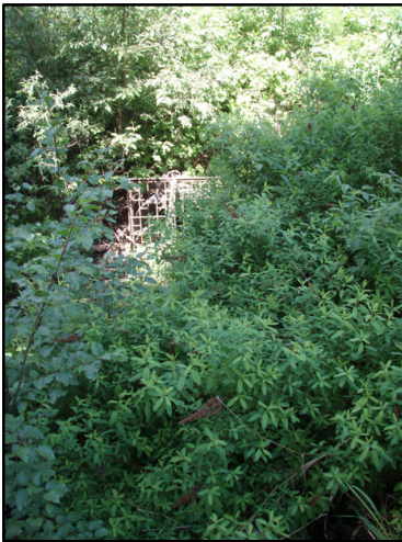
Figure 41. Site 240 culvert inlet. View downstream to inlet
