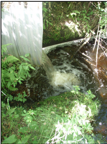
Figure 44. Site 240 outfall drop
