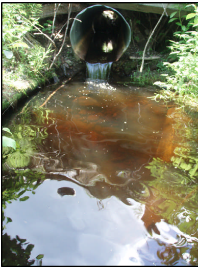
Figure 49. Site 239 culvert outlet. View upstream to outlet.
