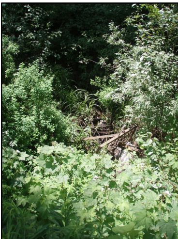
Figure 45. Site 240 inlet side view
