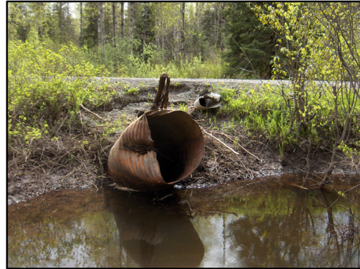
Figure 33. Kline Creek culvert inlet. View upstream from inlet.
