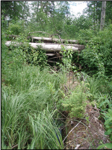
Figure 46. Site 239 culvert inlet. View downstream to inlet.
