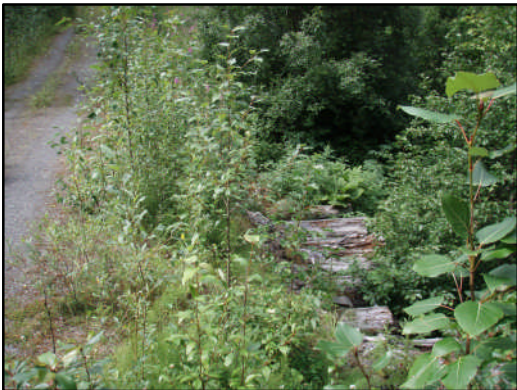
Figure 55. Site 390 Corduroy and road bed.
