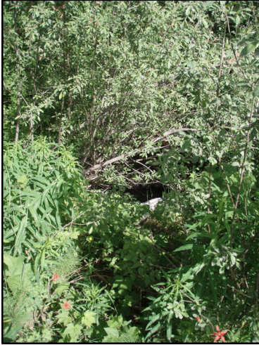
Figure 43. Site 240 culvert outlet. View downstream to outlet.
