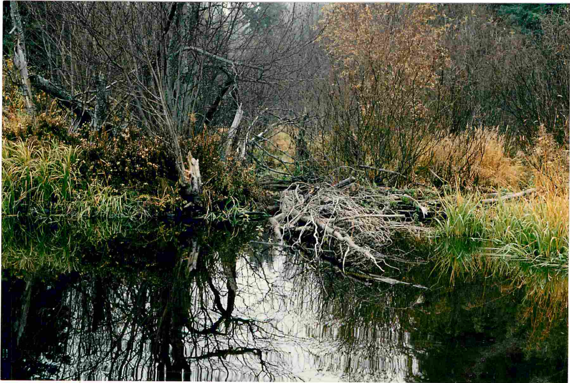
Figure 12. Looking downstream at second partial block of the McBrierie Lake outlet stream.
