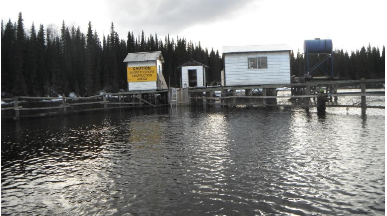
Figure 5. Front view of the Babine smolt enumeration facility, with the wire mesh leads, and the entrance to the smolt trap in the middle of the two leads.
