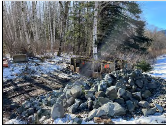
Photo 20 – fishway boxes ready to be loaded out
