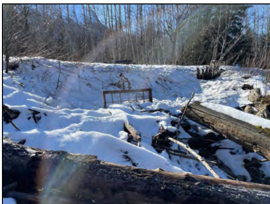
Photo 3 – looking towards the culvert inlet
