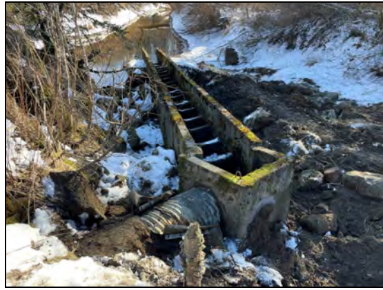
Photo 12 – site overview before boxes were moved
