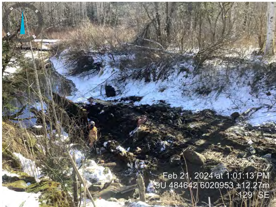
6 Partial removal of fishway
