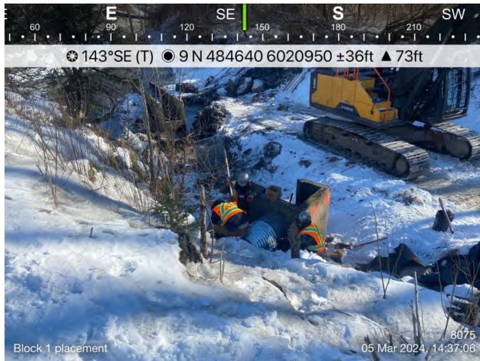
3 Installing culvert junction
