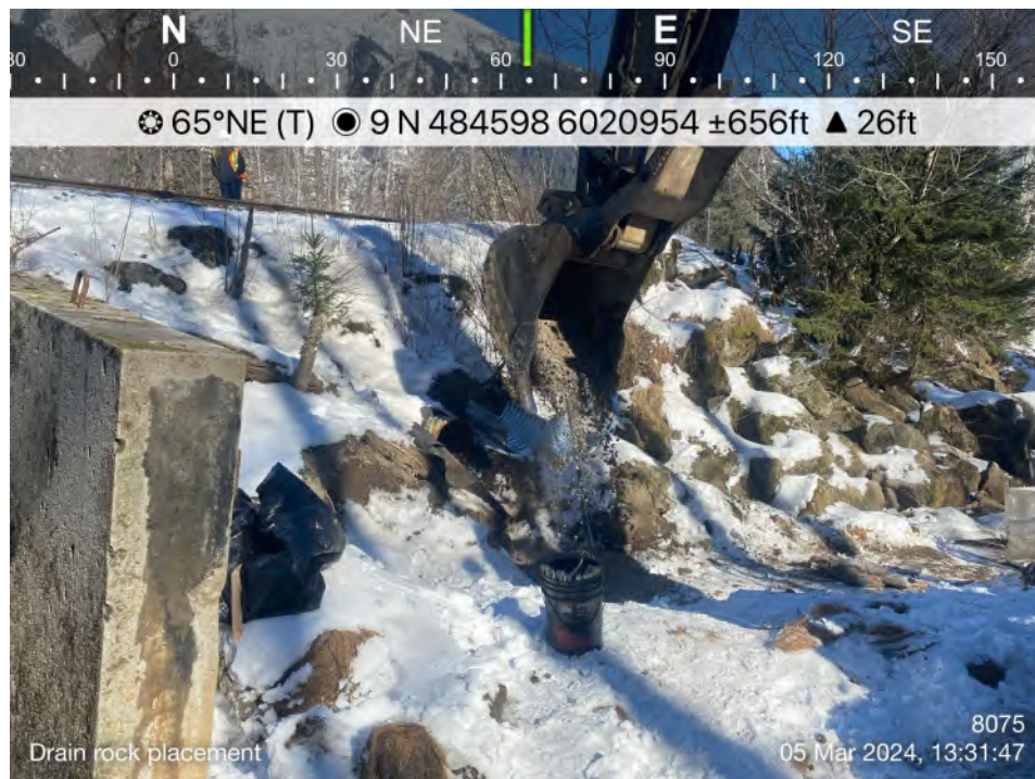
4 Drain rock application
