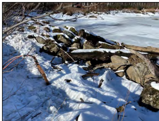
Photo 4 – the culvert inlet is set on the grade seal. Fish were observed at the toe, in the open water.
