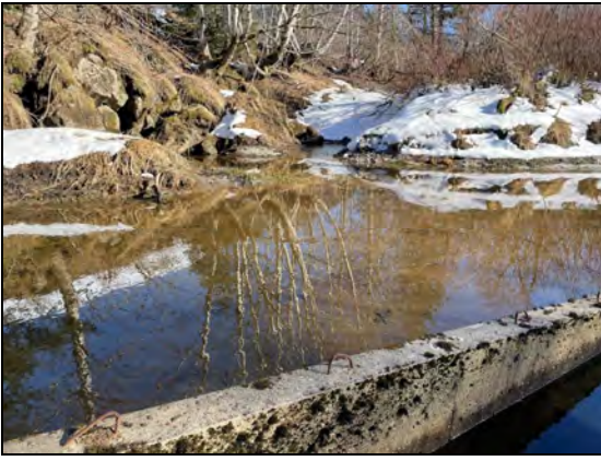
Photo 5 – toe of the downstream embankment
