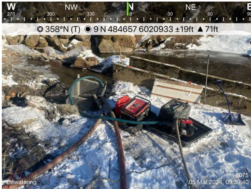
10 Pumps, gen set in spill tray, fish screens in use
