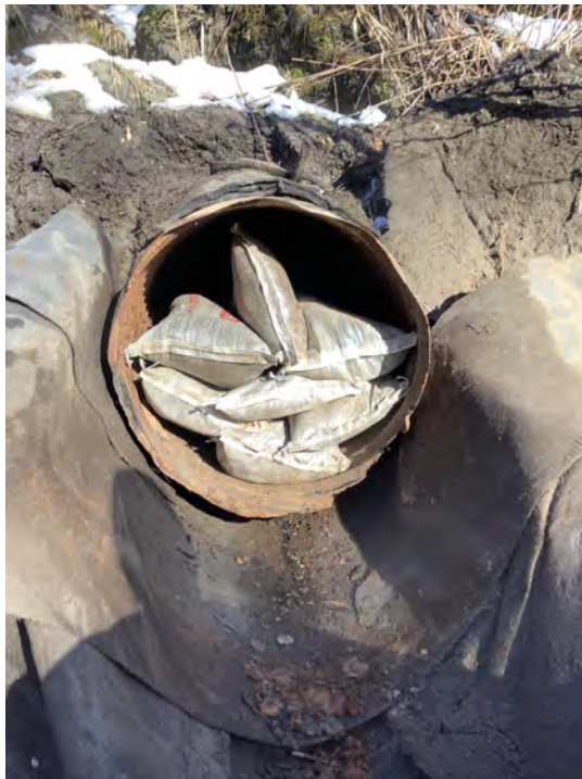
6 Sandbags in culvert to block potential flow
