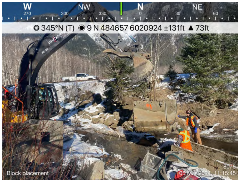
7 Block 9 placement including view of con sealant
