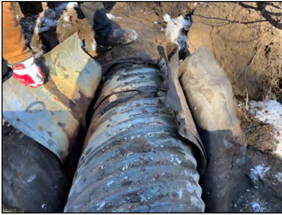
Photo 11 – collar at the culvert stub incorporated a sealer product as well as filter cloth
