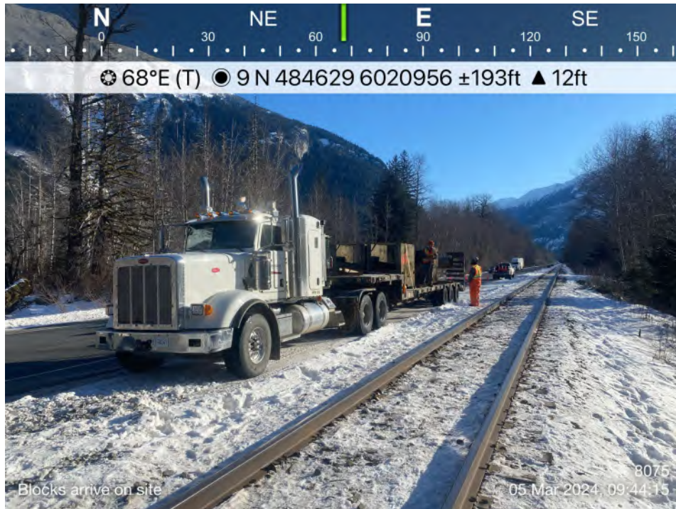
9 Remainder of blocks arrive on site
