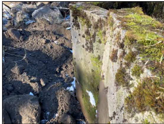
Photo 10 – ground conditions outside the top box of the fishway, gravels with riprap.
