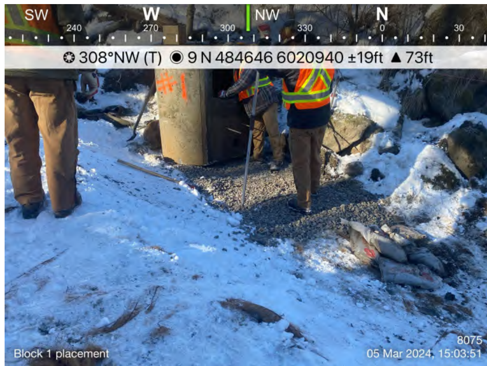
2 Adding drain rock under block 1
