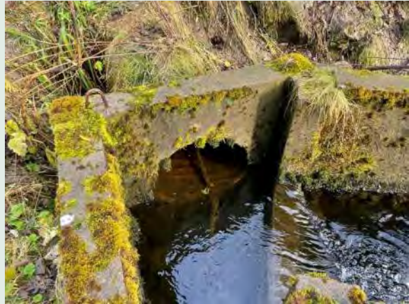
Photo 2 - Culvert Outlet View
