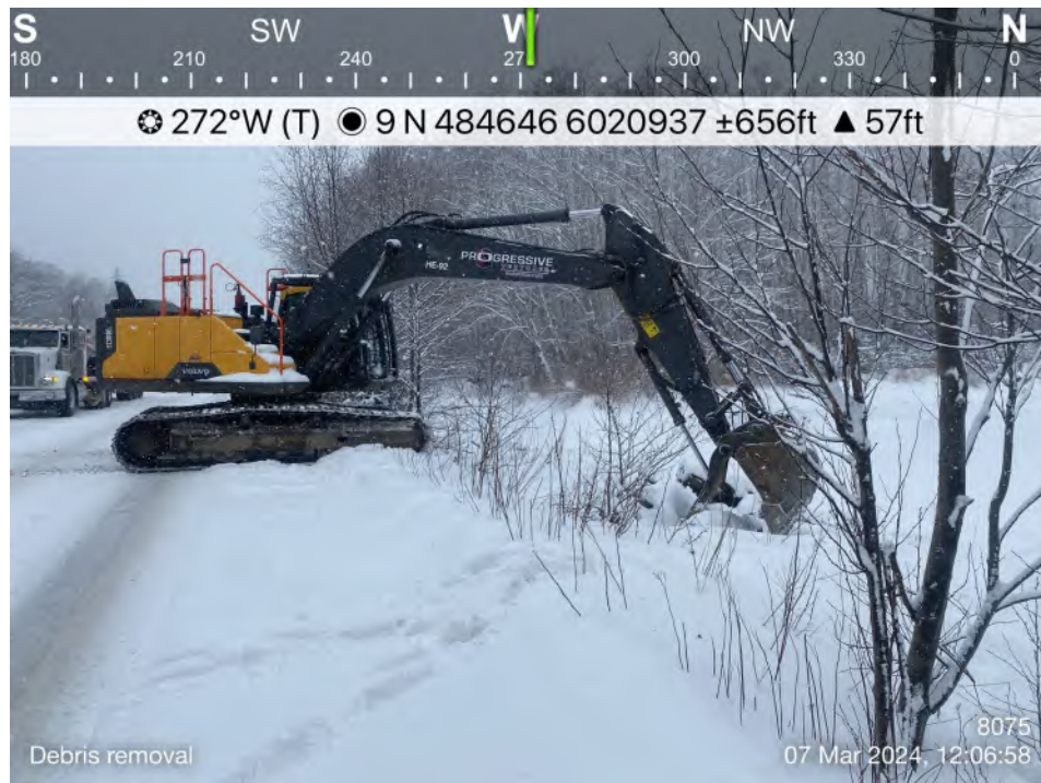
3 Excavator clearing woody debris from upstream side of culvert.
