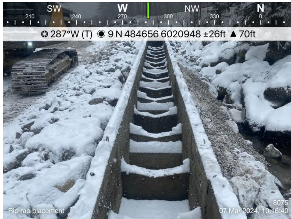
7 Fishway after completion of installation.
