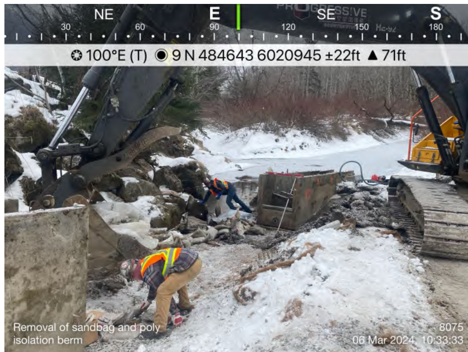
6 Removal of isolation berm.
