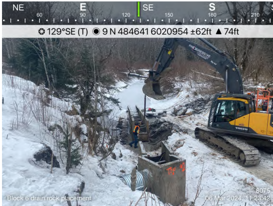
7 Placing drain rock for block 6.
