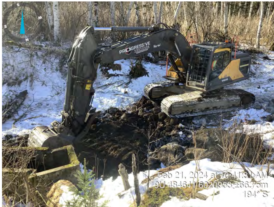
5 Excavator removing rip rap from west side of fishway
