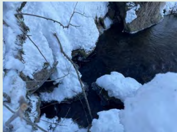
Photo 10 - Flow through the Riprap in Low Water
