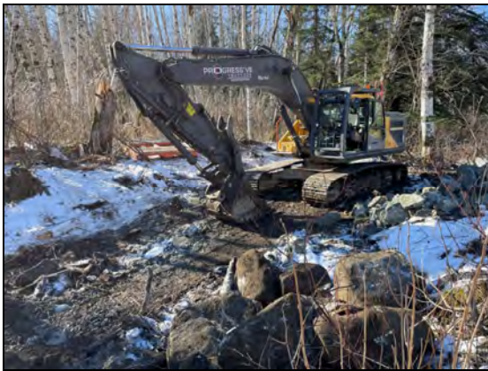
Photo 13 – the parked excavator, for proximity to the creek
