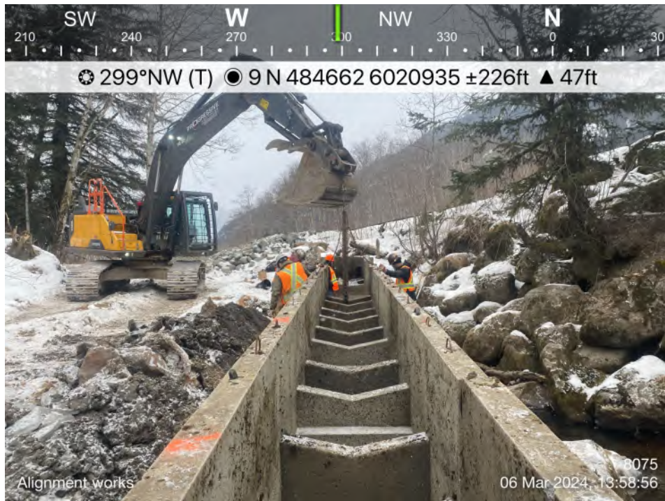
8 Alignment works in progress. All blocks placed.
