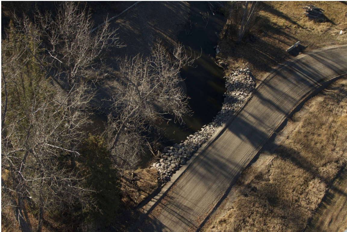
Figures 1 and 2. Confinement of the Upper Bulkley River due to railway infrastructure (top), and use of rip-rap to stabilize “Forestdale” road on the Upper Bulkley River 2km downstream of Bulkley Lake (bottom), October 2013. Photos: Brian Huntington.
