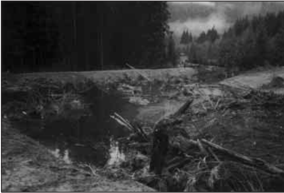
Figure 2-13. Newly excavated pond prior to replanting. Pond depth ranges from >3 m along the berm to the left to 0.3 m to the right. Overflow is located where the person is standing on the berm.
