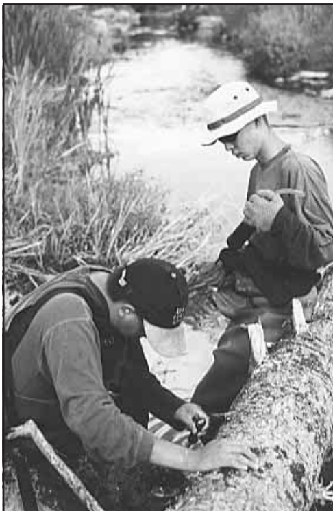
Figure 7-24a. Anchoring LWD structures.
