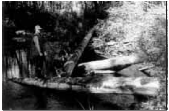
Figure 1-38. Site 6, lower Spirit Creek after LWD placement.
