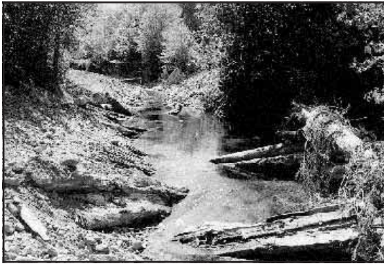
Figure 1-14. LWD structures, pool and riffle structure in the first 100 m of the upper Kennedy side channel.
