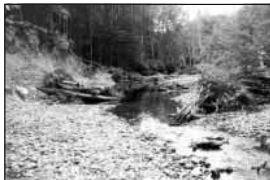
Figure 1-31. Downstream view showing four small LWD structures positioned to protect a steep eroding gravel cutbank. The left structure is 2 m high at the bank.
