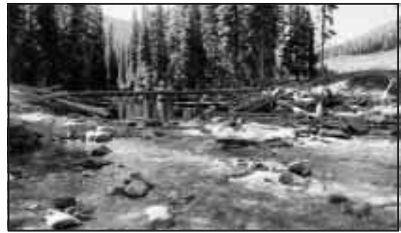
Figure 4-48. Newbury type riffle and natural material bank revetment at a deactivated bridge crossing.
