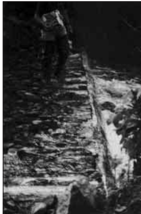
Figure 7-6. Site 13. A Hewitt ramp structure was constructed in a long riffle section. Cedar logs were manually sawn to create 8 foot cedar planks on the ramp. The restored site now provides deep backwater pools and an overall increase in wetted habitat and cover under the structure.
