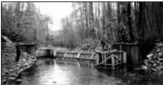
Figure 5-4. Fish counting fence constructed on lower Hagensborg Slough.
