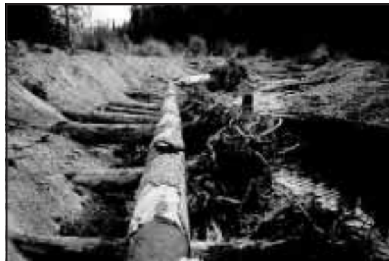
Figure 3-9. Log crib wall.
