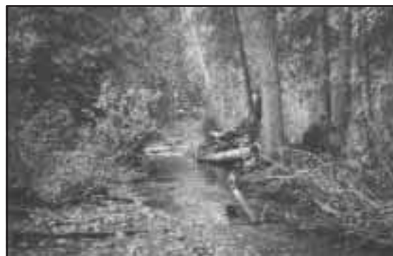
Figure 4-24. Post-work downstream view of spruce tilt log, re-oriented rootwad and re-established stream course on Pass Creek.
