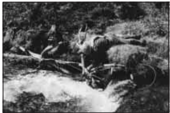
Figure 4-69. Rootwad LWD placement will provide bank stability and create habitat.
