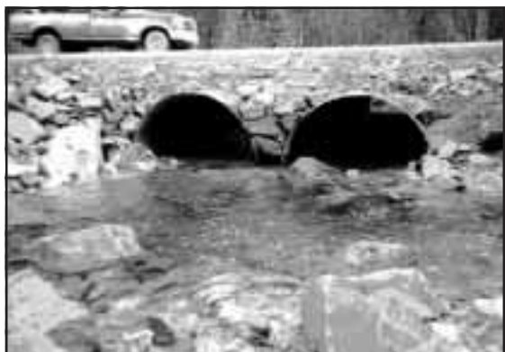
Figure 5-15. Culvert site at 19 km - 1300 Road, Cottonwood River watershed after construction of a downstream riffle.
