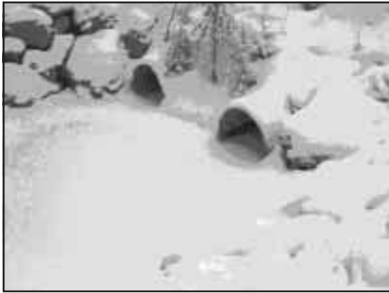
Figure 5-12. Culverts backflooded after weir installation.
