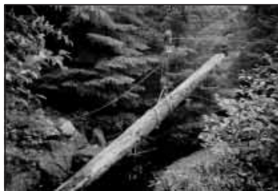
Figure 6-20. A large Western red cedar log being moved from the road to the creek using a skyline and chainsaw winch.
