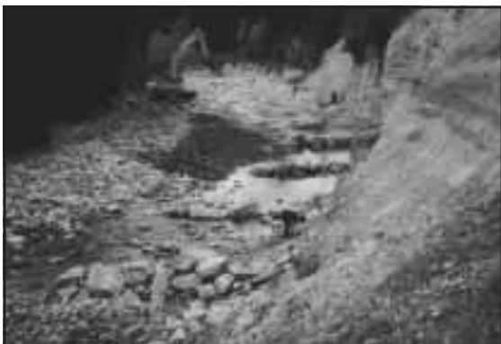
Figure 3-33. View in a northerly direction of Granite Creek facing downstream after installation of the Bendway Rock Weirs (24 September, 1998).
