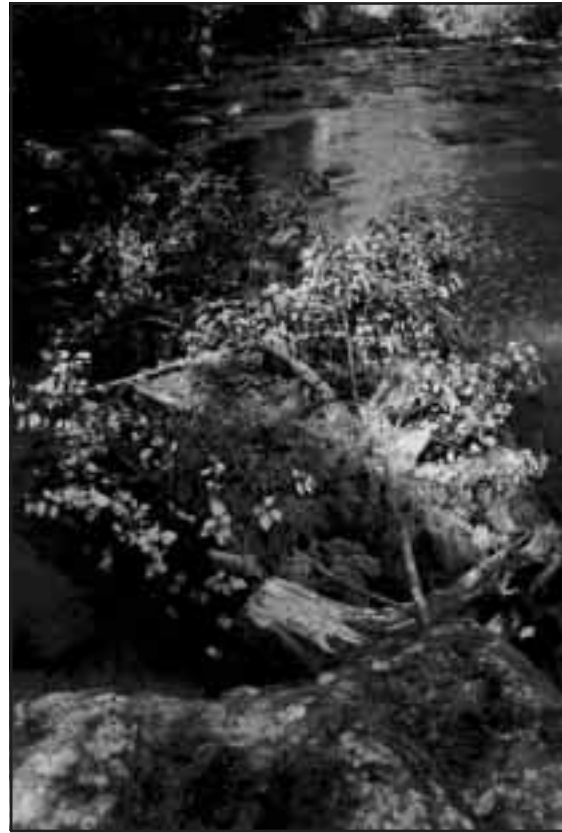
Figure 2-6. A LWD/boulder complex loaded with alder and cedar tops and branches to increase complexity.
