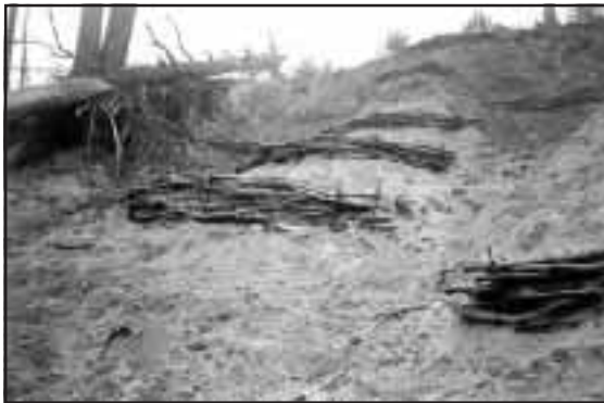
Figure 4-38. Landslide stabilization using wattle fences, live smiles and buried live pole drains (in gullies).
