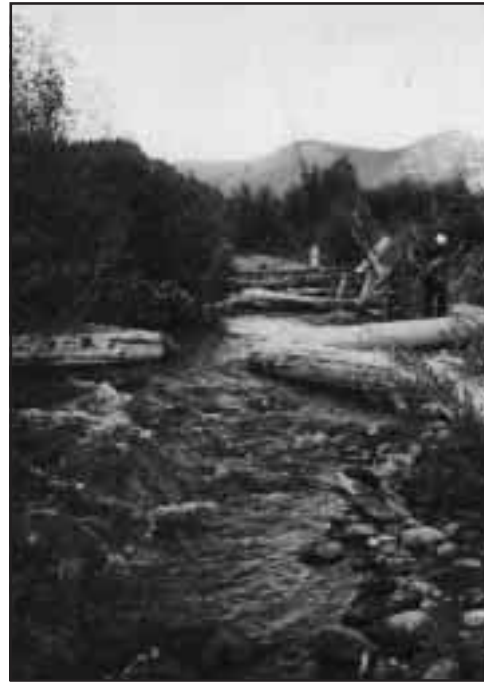
Figure 7-5. Site 9/10. Post-restoration photo of stabilized opposing V-wing deflectors, creating pool habitat, focusing scour, and reducing flow velocities throughout the habitat units.
