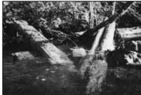
Figure 1-22. Lateral debris jam structure created by combining 2 double floating log structures, placed in 1996, with a new LWD piece and extra boulders. Structure was placed to provide protective cover element to an existing pool. (Note: structure is built around an existing natural log.)
