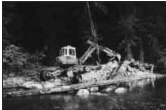
Figure 3- 44. A box groin structure, one of four installed in the West Kettle River in 1998 to provide fish habitat cover and promote pool formation. (During construction, one log to be placed.)
