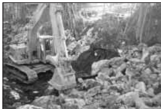
Figure 3-13. Cat 235 C placing heavy rock rip-rap to prevent down-cutting of channel, February 1998.
