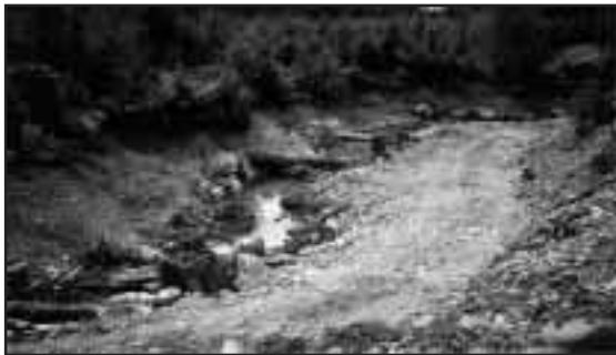
Figure 1-7. Site 18 following completion of the access road. The channel sides have been armoured with rip-rap, and complexing with wood is largely finished.
