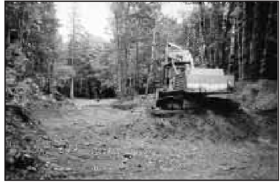
Figure 1-4. A Case 9040 excavator removed the overburden first to reduce the possible sediment load to the channel when it was excavated to grade.
