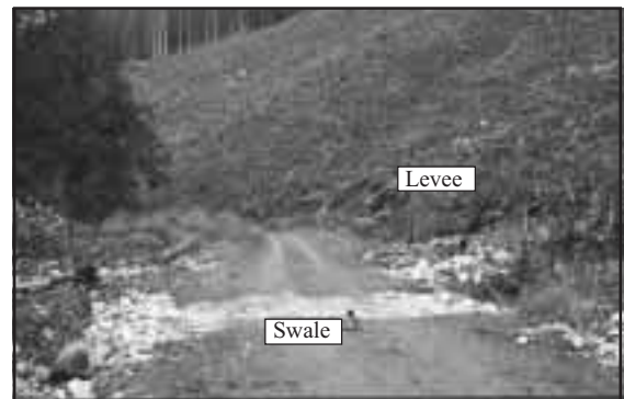
Figure 4-32. Post-work view of cobble swale and ditch block levee at the North Downie FSR crossing of “Shake Block Creek”.
