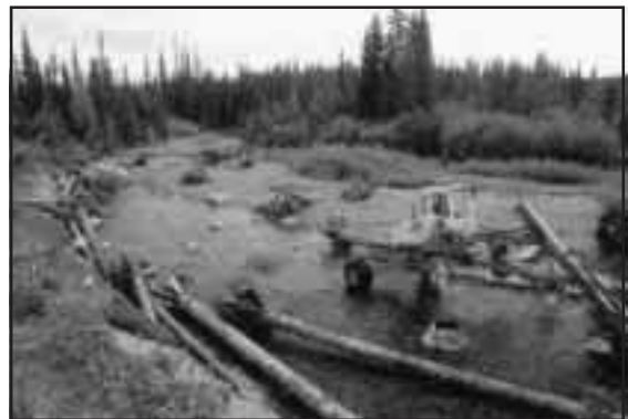
Figure 7-32. Mid-restoration upstream view of large eroding bank along Narrowlake Creek mainstem. Note LWD revetment and rock groynes under construction.
