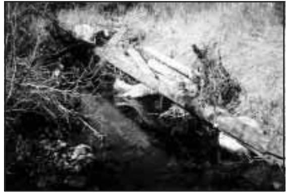
Figure 4-15. A log/rootwad structure on Buckworth Creek provides instream cover and protection to the stream bank.
