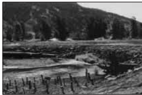
Figure 3-11. Tree revetments and live pole riparian restoration on Deadman River.
