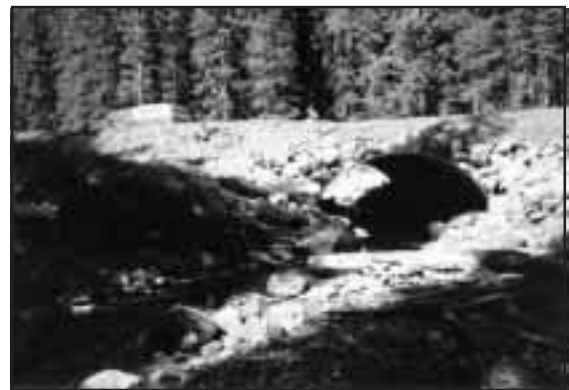
Figure 7-17. Downstream view of crossing #2 following replacement with a bottomless arched culvert.
