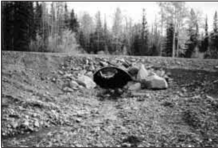
Figure 7-19. Downstream view of crossing #4 following replacement with a bottomless arched culvert and recontouring of the streambed.
