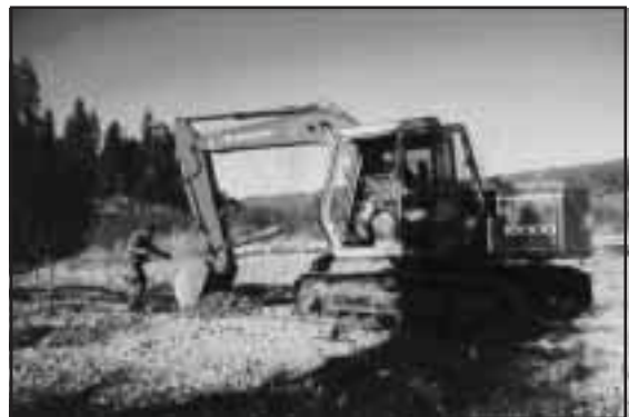
Figure 3-30. Bar planting using excavator. Willow stakes (3-4) were planted per bucket, up to 1 m deep.
