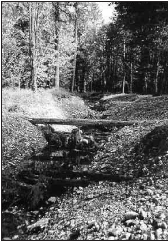
Figure 1-2. A large volume of wood was placed into the main channel to provide cover for adults and rearing salmonids.
