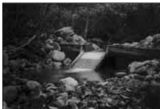
Figure 2-12. Installed and functioning intake designed by Rheal Finnigan, P. Eng. Creek water is diverted through the opening behind the ramp to the head of the new channel via a buried pipe to the right of the intake.
