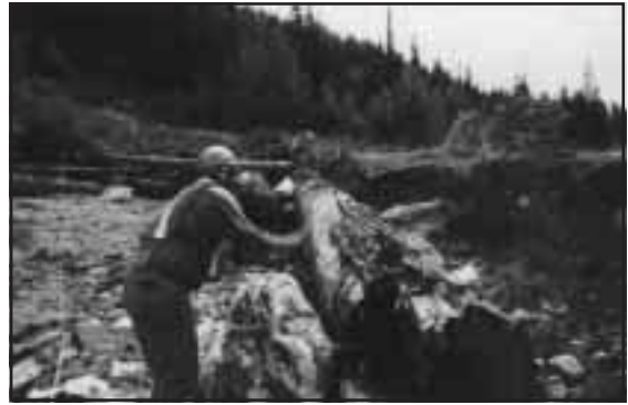
Figure 3-20. Lateral debris jam construction on Danforth Creek (Kingfisher).
