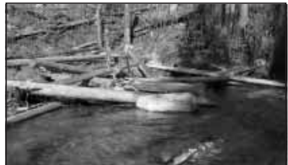
Figure 4-50. A triangular lateral log jam built in a residual pool within a minor bend of Redding Creek.
