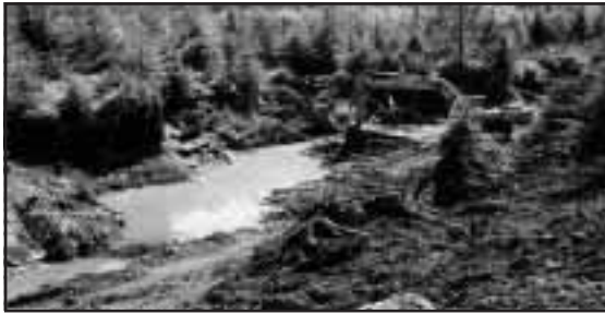
Figure 1-6. Site 18 in the upper portion of the Cypre side channel, with completion of the fourth pass to grade. As much of the southeast bankside vegetation as possible was retained during channel construction.
