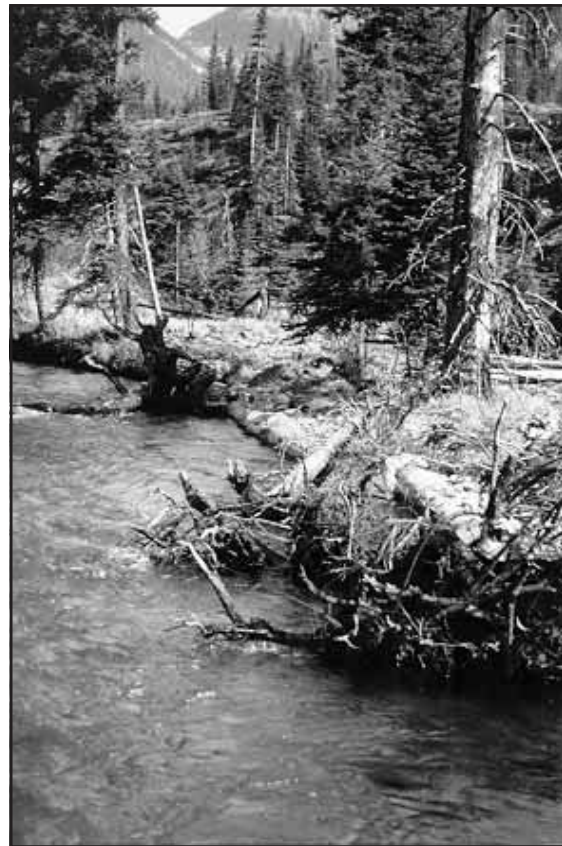
Figure 4-66. Whole tree revetment to protect eroding bank. Note energy dissipation along bank margin.
