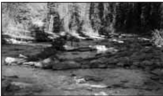
Figure 4-47. Spur log/rock weirs in the foreground with opposing natural material bank revetment in the background.
