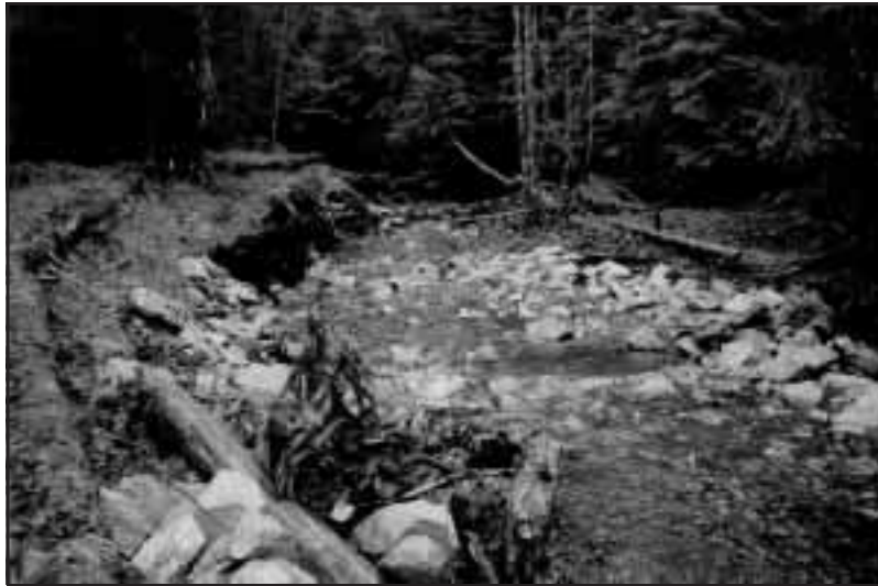
Figure 6-3. Reach 2C3 V-shaped deflector installed under a bridge to protect an eroding bank and promote channel scouring
