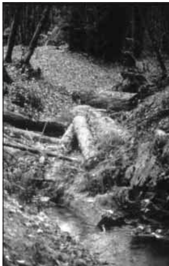
Figure 2-62. LWD placed in upper portion of channel below intake.
