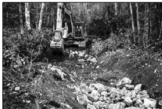
Figure 2-61. Outlet channel during restoration.
