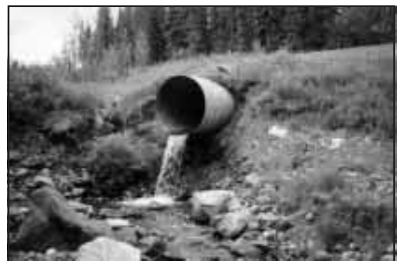
Figure 7-18. Upstream view of crossing #4 before restoration. Note the 1.5 m drop at the outfall.
