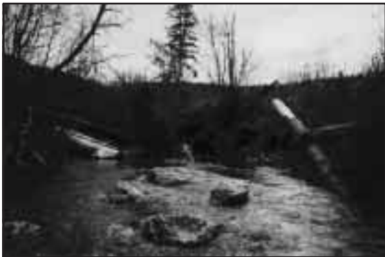
Figure 7-3. Site 7. Post-restoration showing the addition of bank deflectors, LWD in pools, and a boulder garden.
