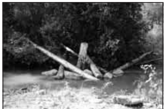
Figure 7-29. Low profile LWD structure designed to maintain pool habitat through bed scour.
