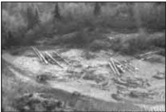
Figure 7-36. Post-restoration view of multiple lateral gravel bar stabilization structures in the lower reaches of Narrowlake Creek.
