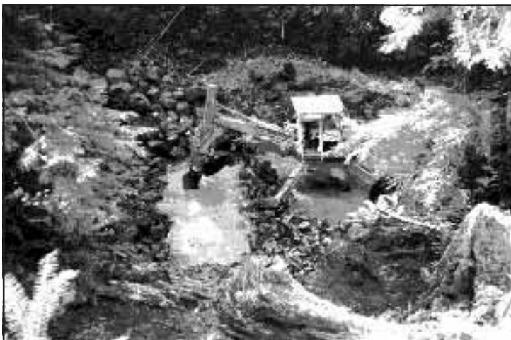
Figure 1-34. Constructing a rock riffle on the North Tributary. The “spider” is excavating a trough across the channel to key the riffle 1 m into the bed.
