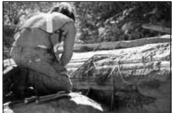
Figure 3-40. Using a rotary hammer to drill holes in a boulder.
