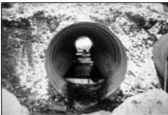
Figure 7-15. Upstream view of crossing #1 with the baffles installed in the culvert but prior to construction of the downstream riffle.
