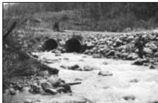
Figure 4-25. Pre-work view of partially embedded culverts posing a velocity barrier to the upstream movement of bull trout in Pass Creek.
