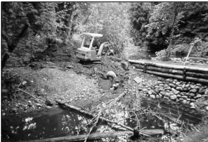
Figure 6-15. Additional culvert intake installed to increase low flow levels in the side channel.
