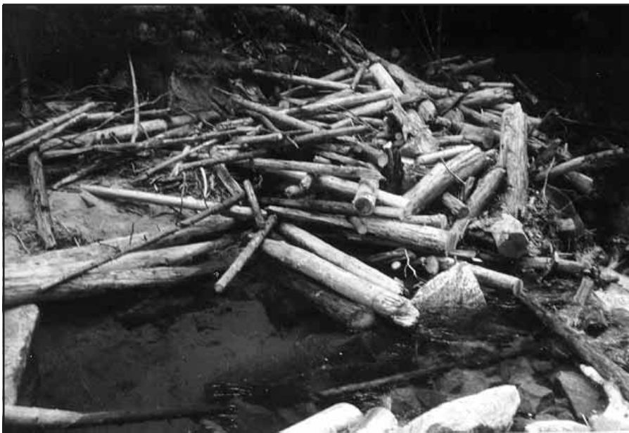
Figure 4-59. The channel of Sanca Creek is opened but logs were left in and above the pool to provide cover for trout.
