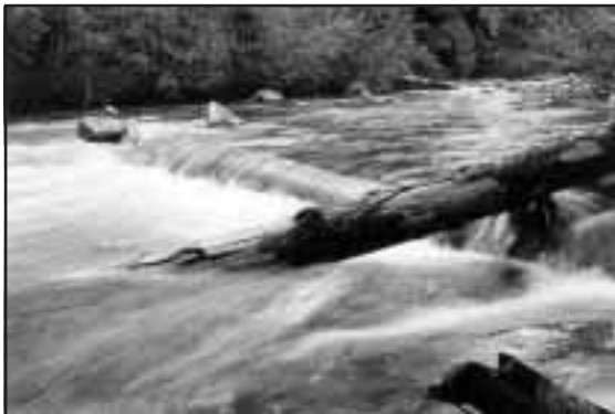
Figure 3-37. Properly functioning diagonal LWD weir, installed in 1997.
