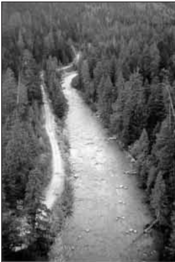
Figure 4-44. Post-project conditions. Note boulder clusters and three lateral log jams.
