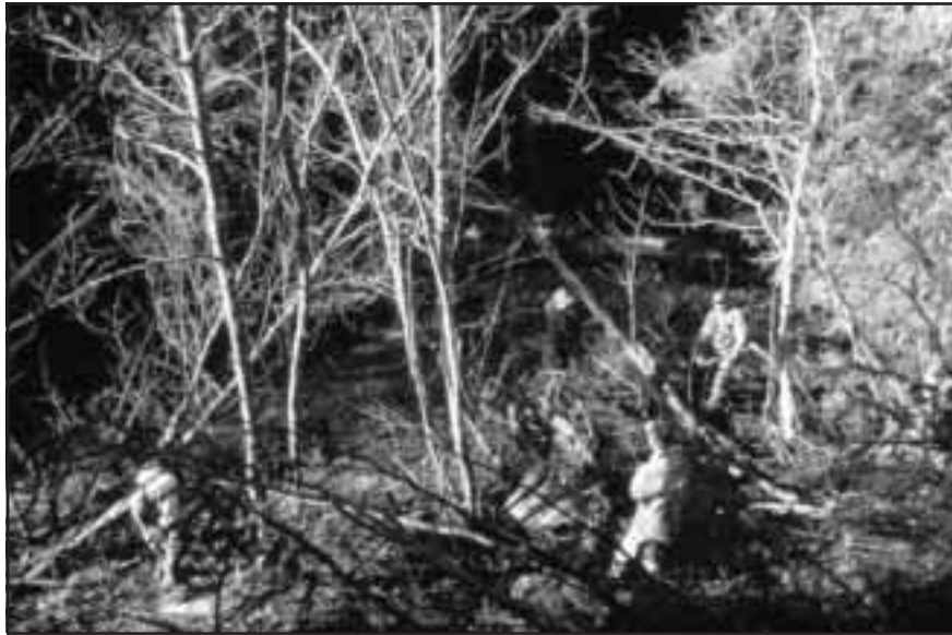
Figure 7-12. Manual labourers from Lheidli T'Enneh First Nation maneuvering large woody debris into McPhee Creek with winches and block and tackle.
