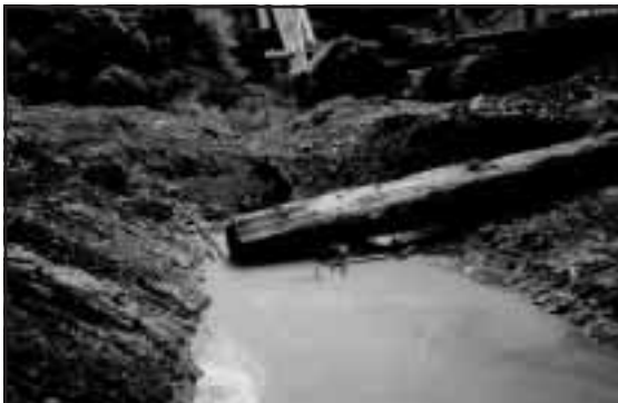
Figure 6-22. Excavation of channel in preparation for the installation of the second upstream log.
