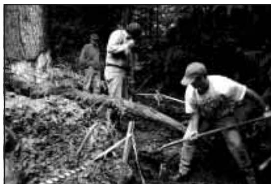
Figure 5-34. Initial hand excavation of beaver dam bypass channel, Talchako River, 77 km.
