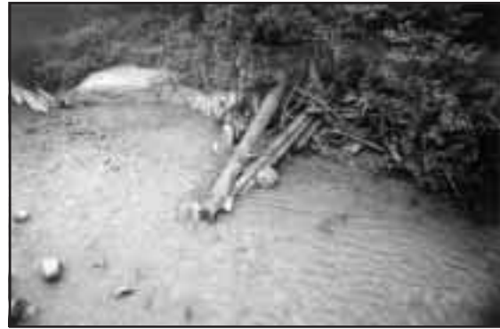
Figure 4-45. Triangular lateral log jam.
