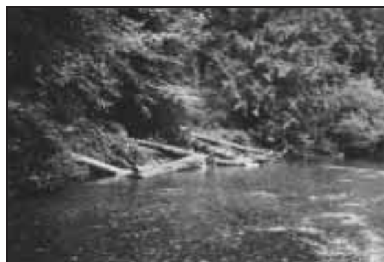
Figure 1-11 . Photograph of Site 7 where a typical lateral log spur was constructed along the right bank.
