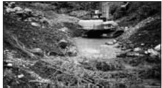
Figure 1-9a,b,c. Construction of an undercut bank using logs supported on boulders, covered with landscape fabric to minimize infilling and backfilled.
