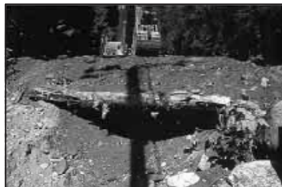
Figure 2-31. Construction of undercut bank at Young Creek.
