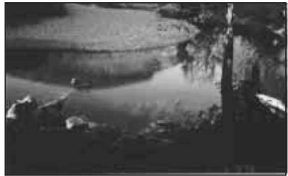
Figure 1-44 . LWD structure at Site 7, Reach 3, Sarita River. Photo shows rooted ends extending into a deep pool.
