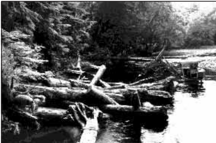
Figure 1-33. Upstream view on the Mahatta River showing two large log jams constructed to protect a gravel cutbank from erosion. A scour pool 20 m long by 12 m wide by 3.5 m deep has formed between the two log jams.
