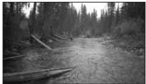
Figure 4-51. A series of three large turning logs placed at 20° upstream angle to transfer the thalweg towards the center of the channel. Note the mid-channel bar stabilization structures in the background.
