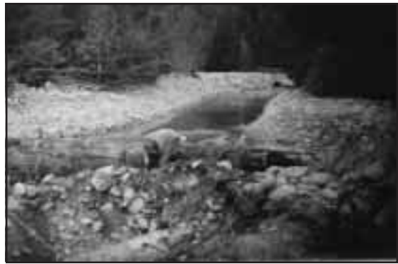
Figure 2-47. Constructed connecting channel and deadman anchoring of LWD.
