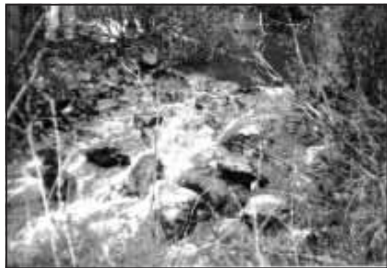
Figure 5-30. Hand constructed rock riffle completed on Rebman Creek mainstem.
