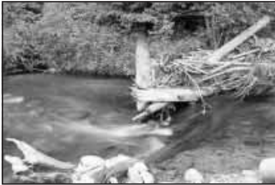
Figure 3-35. Properly functioning lateral debris jam, installed in 1997.
