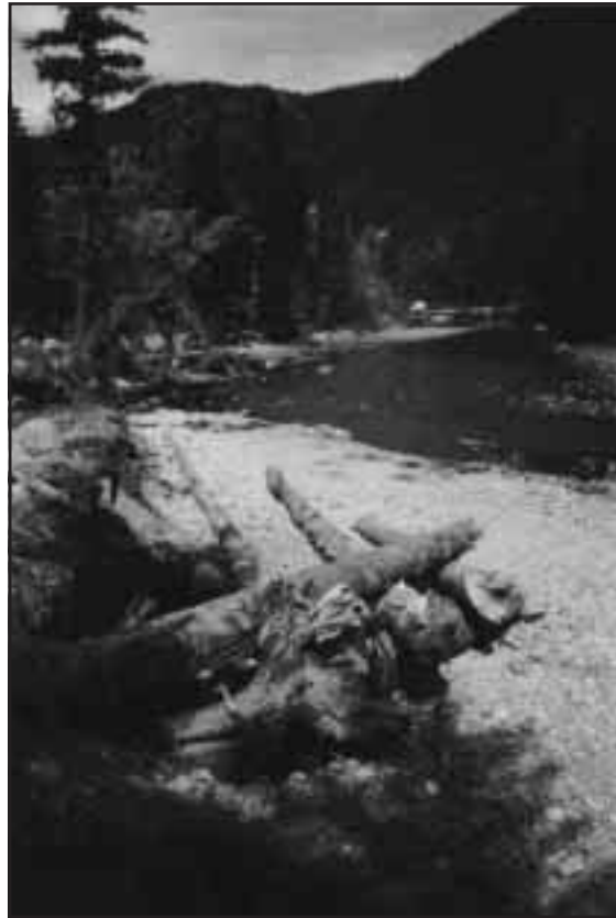
Figure 3- 43. Bank stabilization structures (before ballasting) installed in the West Kettle River as an alternative to the use of rock rip-rap for erosion control.
