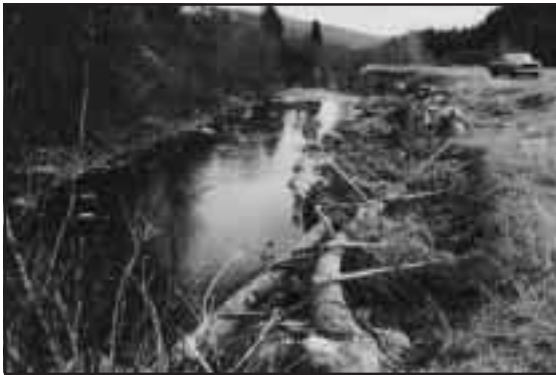
Figure 3-26. Typical river spur structure using large wood pieces, thinned trees, rootwads and boulders; supplemented by planting willow stakes.
