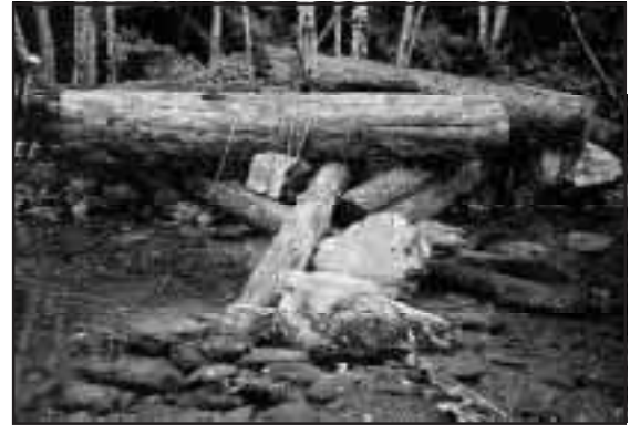
Figure 1-17. Stump Creek side channel LWD structure and excavated pool following first fall flood. Tla-o-qui-aht First Nation crew chief standing beside jam for scale.
