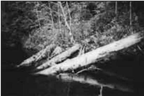
Figure 1-19. Bank protection /debris jam structure placed to protect an eroding bank, scour pool habitat and provide protective cover habitat.
