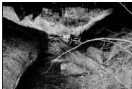
Figure 6-2. Reach 2C3 debris catcher placed on the leading edge of a gravel bar. The structure was pre-loaded with small woody debris.
