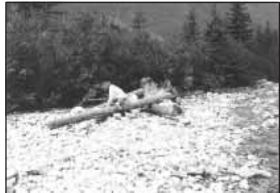
Figure 4-34. Debris catcher at the top end of a meander bend intended to promote bar stabilization and channel narrowing.
