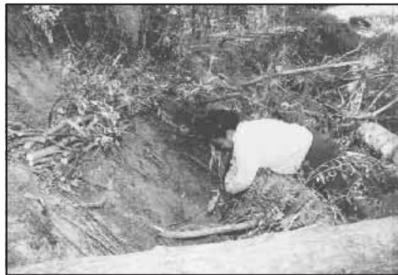
Figure 7-25. Willow wattle and brush layer placement.
