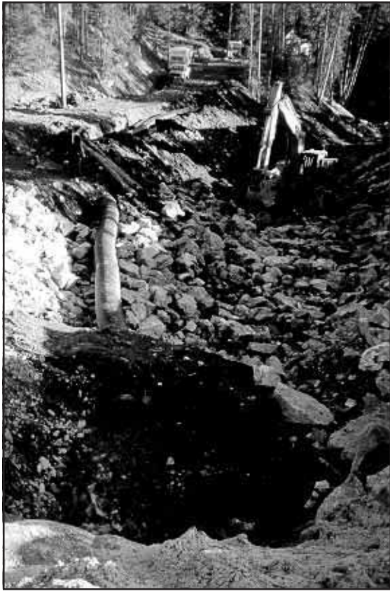
Figure 3-15. Streamflow bypass pipe in Hudson Creek, February 1998.
