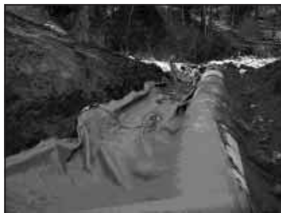
Figure 5-25. Preparing bypass channel.
