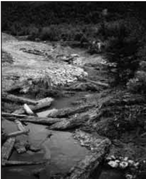
Figure 1-8. Channel complexing using rootwads, lateral revetments and LWD piles.
