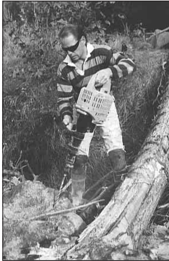
Figure 7-24b. Anchoring LWD structures.
