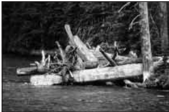
Figure 4-65. Large LWD structure. Note the use of a variety of sized LWD and rootwads for added complexity and strength.
