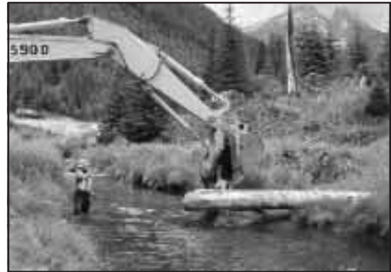
Figure 4-33. Lateral debris jam to provide additional cover in side channel.
