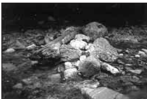
Figure 2-43. Side view of rock deflector.
