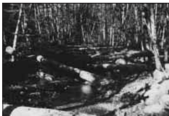
Figure 6-5. LWD added to Reach 6 in Ginlulak Creek to promote scour, improve channel definition and provide cover for coho salmon.
