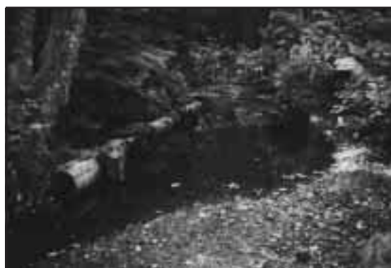
Figure 6-7. One section of Reach 7 after stream cleaning and placement of LWD for cover.
