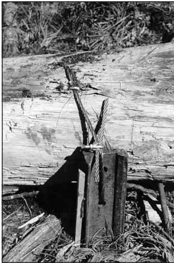
Figure 4-64. Typical placement of anchor “piers” used to supplement boulder ballasting.
