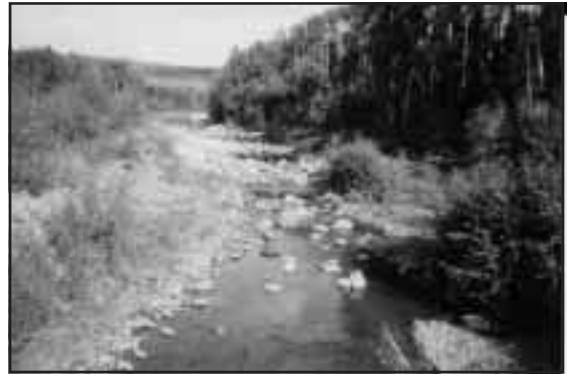
Figure 7-27. Upstream view of channel (from FSR bridge) after riffle-pool construction and LWD placement.
