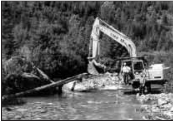
Figure 4-37. Cover log to increase cover, anchored to large boulders in existing pool.
