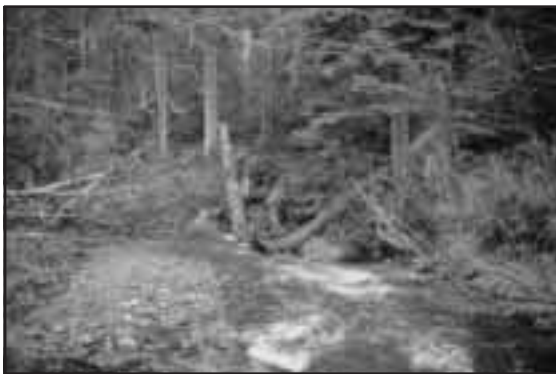
Figure 7-8. Post-restoration photograph of McPhee Creek, Reach 2 site 5. Lateral triangular large woody debris structure constructed in pool to provide overhead cover and induce additional scour.
