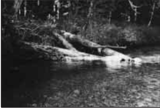
Figure 1-18. Lateral debris jam, located along the Wolfe Creek restoration section, placed to scour pool habitat and provide protective cover habitat.
