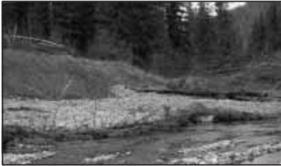
Figure 4-9. The lower groyne with a whole tree deflector incorporated into its streamward edge.
