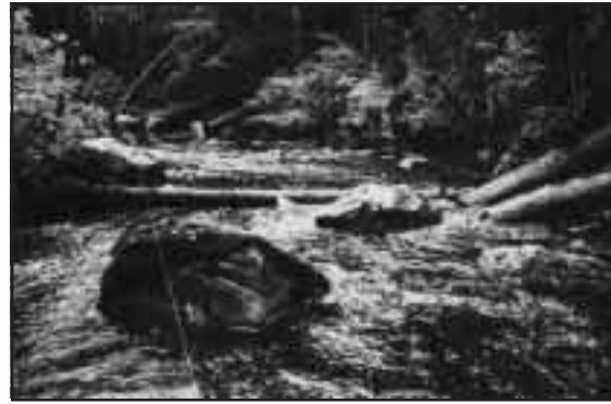
Figure 1-21. Large rootwad added to double deflector log to increase the efficiency of deflector structure. The same treatment was applied to an adjacent structure in an attempt to form a channel constriction to promote bedload scour.
