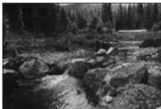
Figure 3-3. Upstream "V" structure to create pool habitat on Arrastra Creek.
