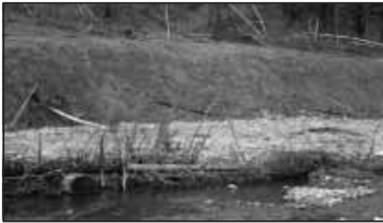
Figure 4-10. The upper groyne. Note the re-contoured hillslope in the background with grass seed starting to become established.
