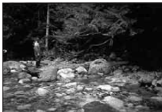
Figure 2-44. Downstream view of constructed rock deflector.
