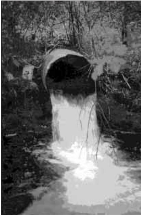
Figure 5-27. Channel is constructed to route stream prior to pulling culvert on unnamed creek.
