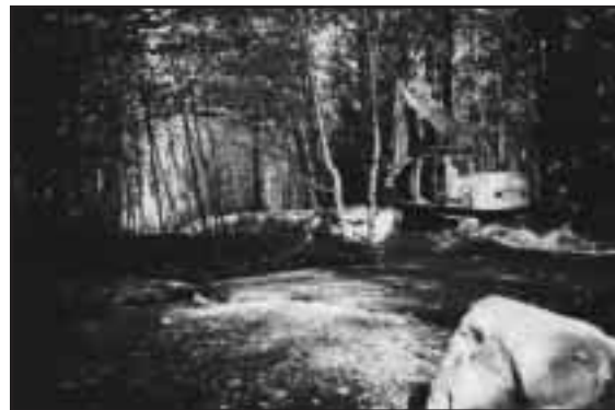
Figure 6-18. Construction of protective berm along right bank of Kwinyarh mainstem to protect newly constructed channel.
