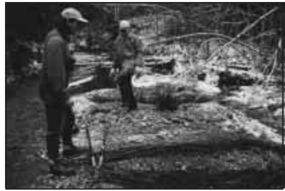
Figure 4-41. Bar stabilization using brush traverses.
