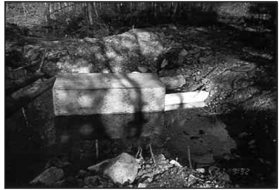
Figure 2-67. Installed beaver box.
