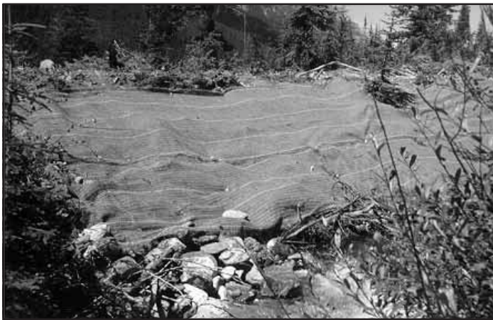
Figure 4-61. Eroding bank re-sloped, toe partially armored and covered with coconut fibre matting.
