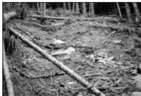
Figure 4-52. Live gully breaks and brush layers on Rover Creek.
