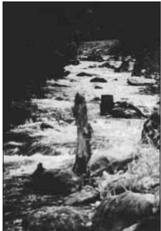
Figure 2-22. Single rootwads were anchored to single boulders to increase complexity. This also shows homogeneity of boulder riffle pattern prior to construction.
