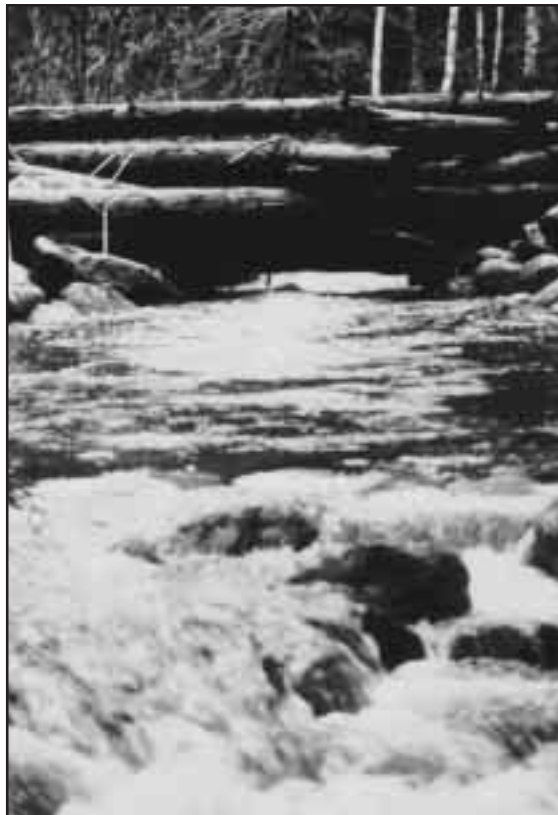
Figure 2-20. LWD and boulders were used to “cap” maximum flows entering the channel.
