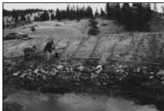
Figure 3-23. Live pole placement and bank stabilization on Shingle Creek.
