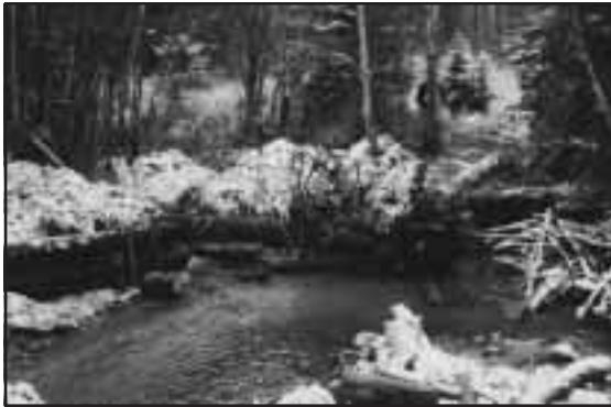
Figure 4-40. Works in progress: streambank stabilization on Inlet Creek incorporating rootwad revetment and log wall armoring.
