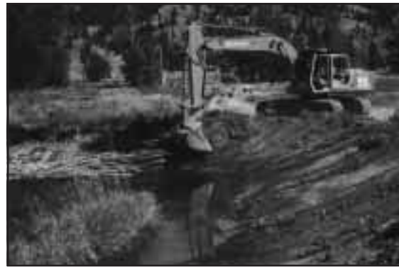
Figure 3-10. Bank stabilization on Deadman River.
