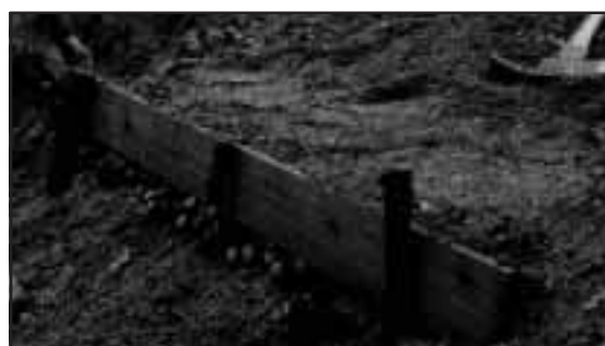
Figure 2-39. Modified brush layer.
