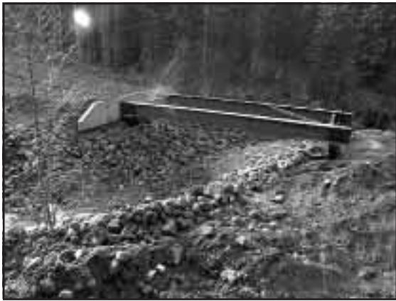
Figure 5-23. Bridge superstructure across reconstructed channel.
