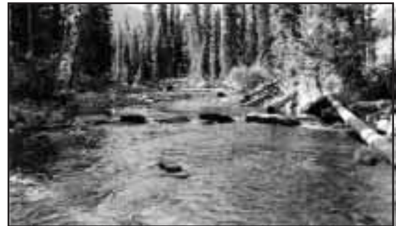
Figure 4-49. Upstream view of vortex type weir.
