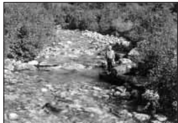
Figure 4-35. Boulder vortex weir and lateral debris jam to enhance existing deep pool habitat with additional depth and cover.
