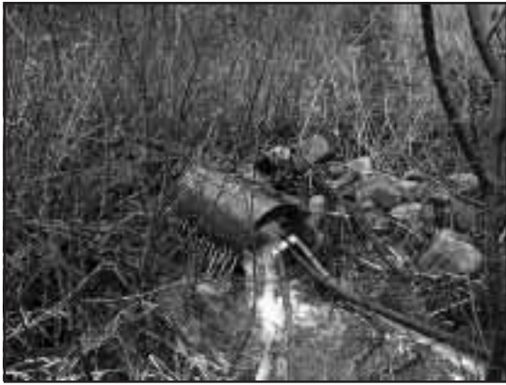
Figure 5-22. Barrel to dissipate pumped water velocity.
