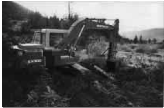
Figure 3-28. Excavator used to tighten and place deadman logs into T-trenches.
