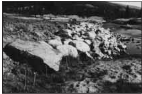
Figure 3-29. Channel manipulation using graded rip-rap and supplemented with planting willow stakes.
