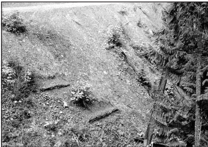
Figure 4-54. Two wattle fences completed on a large raveling slope above Rover Creek. For scale note the worker sitting at the base of the tree.
