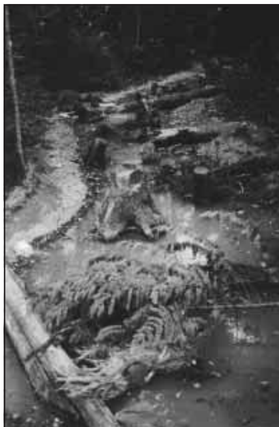
Figure 2-7. Logs placed in channel which followed an unused skidder road.
