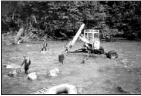
Figure 4-43. “Spider” hoe placing boulder clusters.
