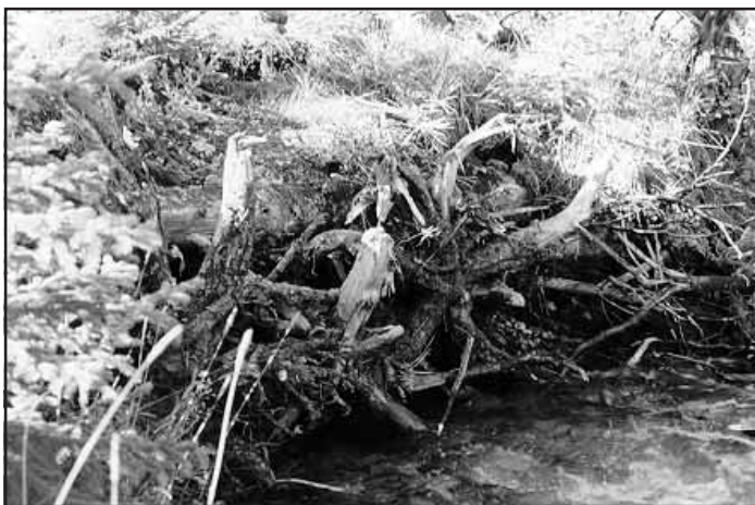
Figure 4-62. Rootwad structure to protect bank and induce pool scour.
