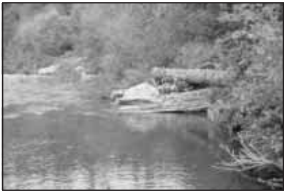
Figure 7-35 Post-restoration view of LWD / boulder deflector.
