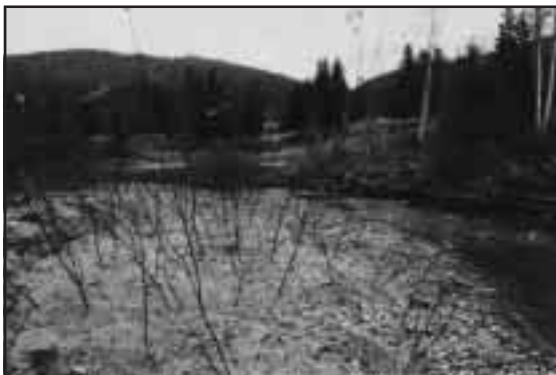
Figure 3-27. Typical river spur on outside bend. Note: large wood pieces, thinned trees and extensive bar planting with willow stakes.
