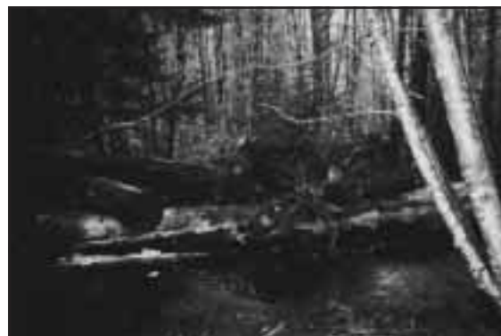
Figure 6-19. LWD jam constructed along left bank of Kwinyarh mainstem to close off an avulsion channel.
