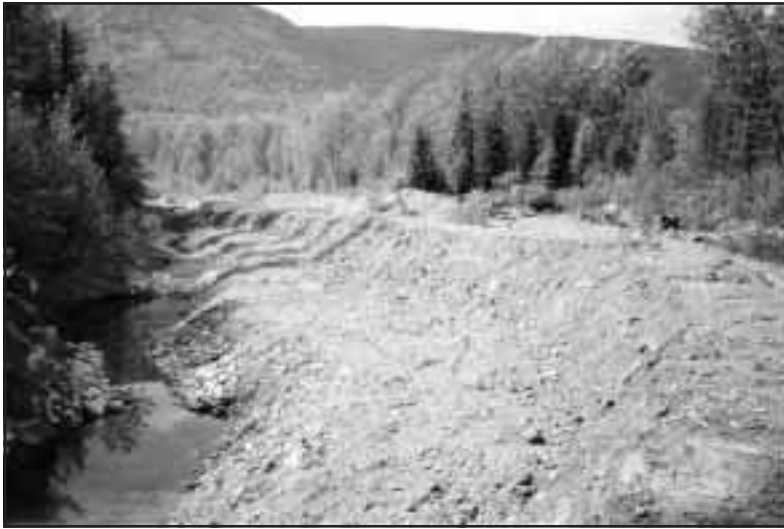
Figure 7-30. Side channel following its excavation to groundwater level and the berm protecting it from high mainstem flows.
