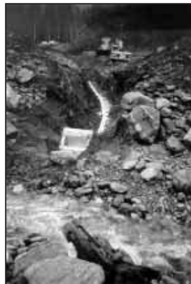
Figure 4-1. Intake box and pipeline installation.
