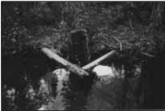
Figure 3-18. Triangular debris catcher on Danforth Creek (Kingfisher).
