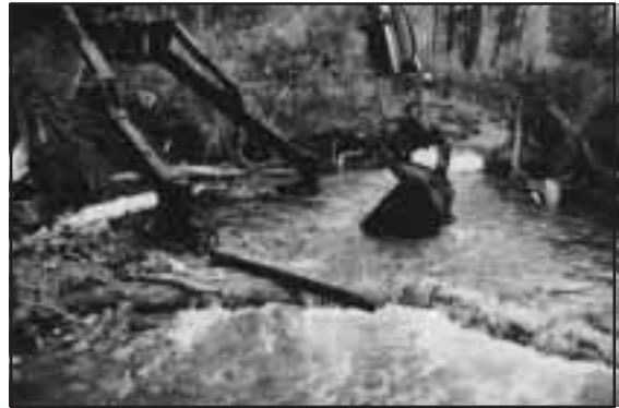
Figure 4-68. Placement of a log V-weir will provide gradient control following debris removal.
