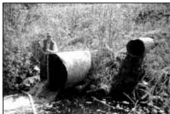
Figure 5-24. Culverts prior to replacement.
