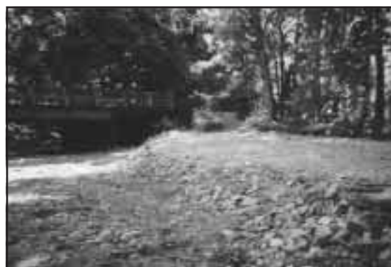
Figure 1-10 . Photograph of Site 2 in Reach 1 of the Goldstream River where the left bank was reconstructed using logs, rip-rap and gravel.
