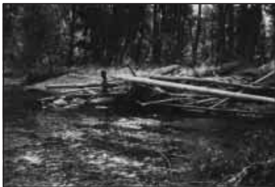
Figure 3- 42. A lateral log jam structure installed in the West Kettle River in 1997. The triangular structure accumulated debris during the spring flood.
