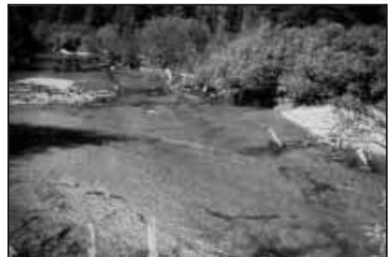
Figure 4-18. Perpendicular LWD post-notch log prescription. Note: increased local velocity and active down-cutting under base flow conditions.
