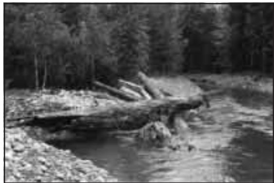
Figure 2-48. LWD structure on the outside of a meander bend.
