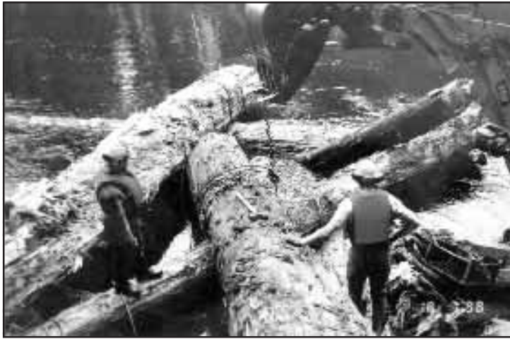
Figure 1-32. Constructing a large log jam on the Mahatta River. Logs are cabled across the structure to stiffen the log jam.
