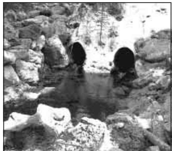
Figure 5-11. Culverts prior to weir construction.
