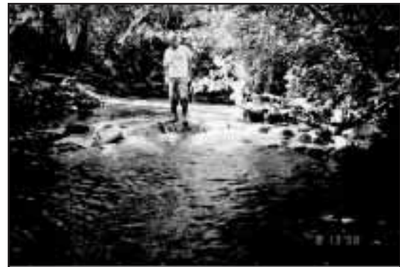
Figure 3-21. Boulder weir to create scour pool and central thalweg.
