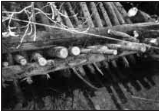
Figure 4-13. Structure #8 on Buckworth Creek, a revetment designed to minimize further undercutting of the stream bank and provide instream cover.
