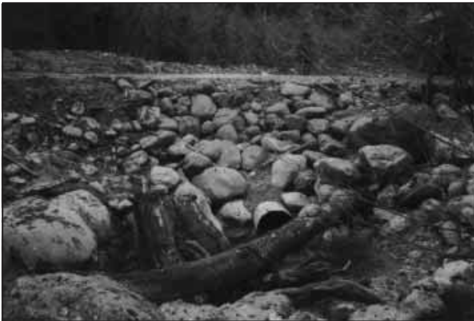
Figure 2-14. New 18 m x 800 mm culvert installed under the Statlu Forest Service Road. Culvert was installed at 0% gradient and submerged to facilitate perennial fish access from Statlu Creek to the new habitat.
