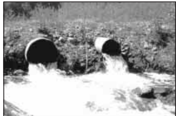
Figure 5-5. Culverts prior to replacement.
