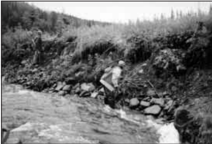
Figure 7-20. Horizontal willow staking of an eroding cutbank on Blue Grave Creek.
