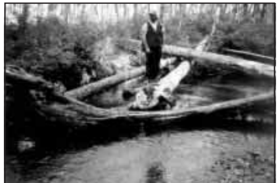
Figure 1-40. Site 13A, upper Spirit Creek after LWD placement.
