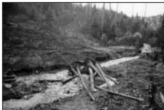
Figure 6-9. Upstream view of Site 3 showing the site immediately after the bridge pull back. The banks were seeded and LWD was placed in the channel to later be dispersed in prescribed locations downstream.
