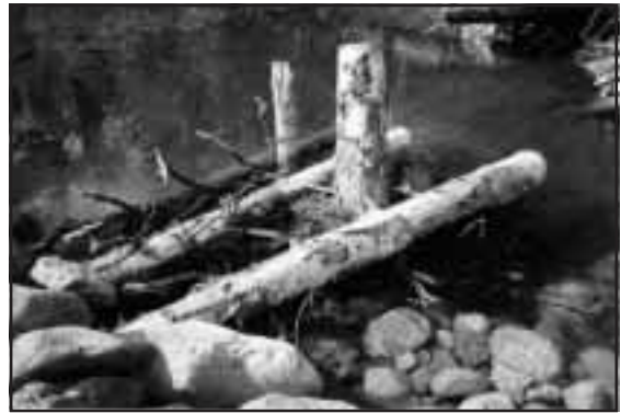
Figure 7-28. LWD structure constructed over a pool excavated below riffle #8.
