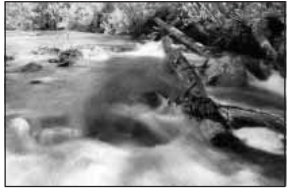
Figure 3-38. Failed diagonal LWD weir. Inadequate ballast/anchoring on left side, installed in 1997.
