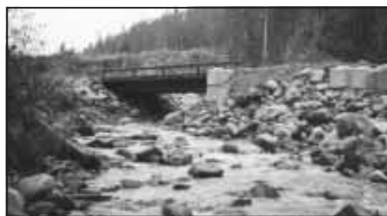
Figure 4-26. Post-work view of clear span bridge stream crossing of Pass Creek.
