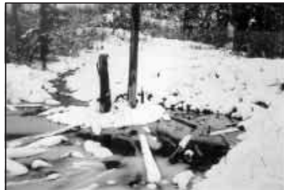
Figure 4-6. Lower pond after removal of peninsula. Note clean water and longer outlet channel with increased flow from main pond.
