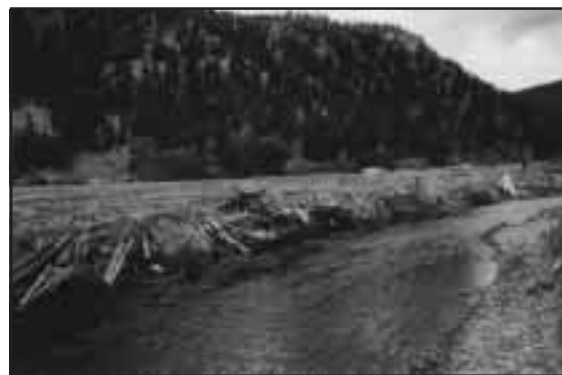
Figure 3-12. Tree revetments to stabilize banks on Deadman River.
