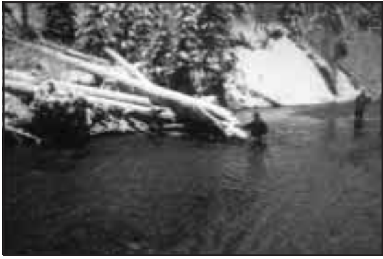
Figure 7-34. Post-restoration view of lateral LWD jam. Note depth of pool scoured out after October rainstorms. Large woody debris cover in pools is increased on average 20% following restoration.
