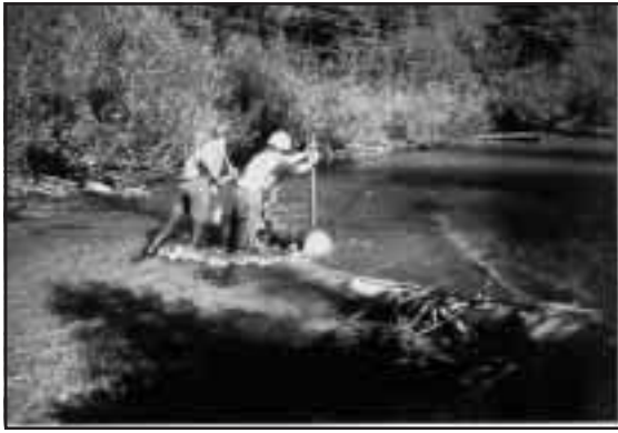
Figure 4-19. Notch log prescription. Work crew removing mid-portion of problem LWD.
