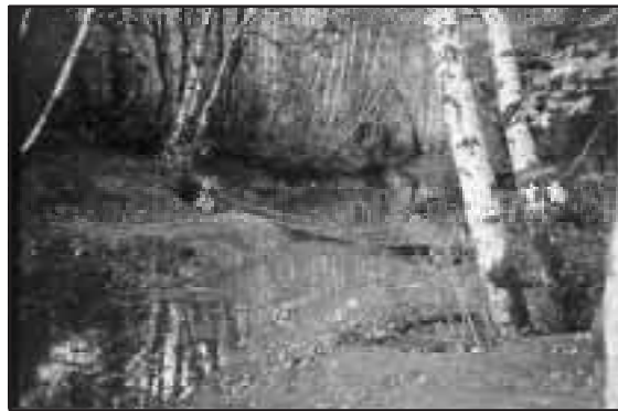
Figure 1-42. After construction, the wetted area of the side channel was greatly increased. Additional LWD still has to be added.
