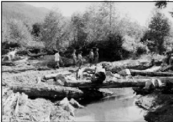
Figure 1-15. Rip-rap banks, LWD structures in the upper Kennedy side channel at 4+90 m.
