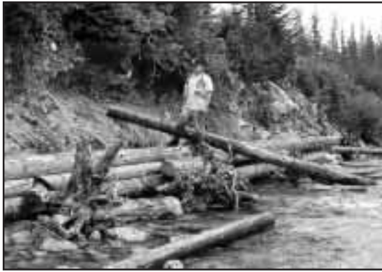
Figure 4-36. Bank revetment with rootwads and lateral debris jam to stabilize toe of slope and increase cover.
