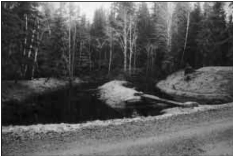
Figure 1-23. Off-channel ponds at the upper Keogh River. The lower pond (center) was excavated within the old cut-off river flood channel, and the upper “flooded” pond (left edge of photo) was created by constructing a berm with material excavated from the lower pond.
