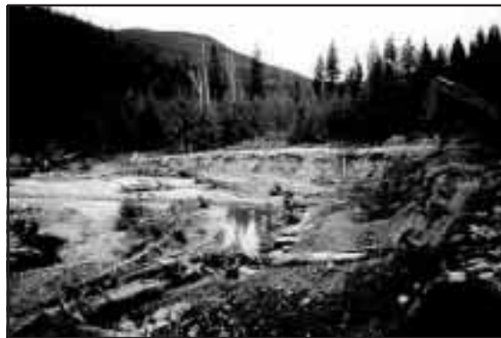
Figure 3-8. Constructing log crib wall along toe of slide.
