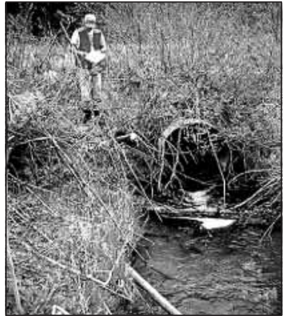
Figure 5-21. Culvert prior to replacement.
