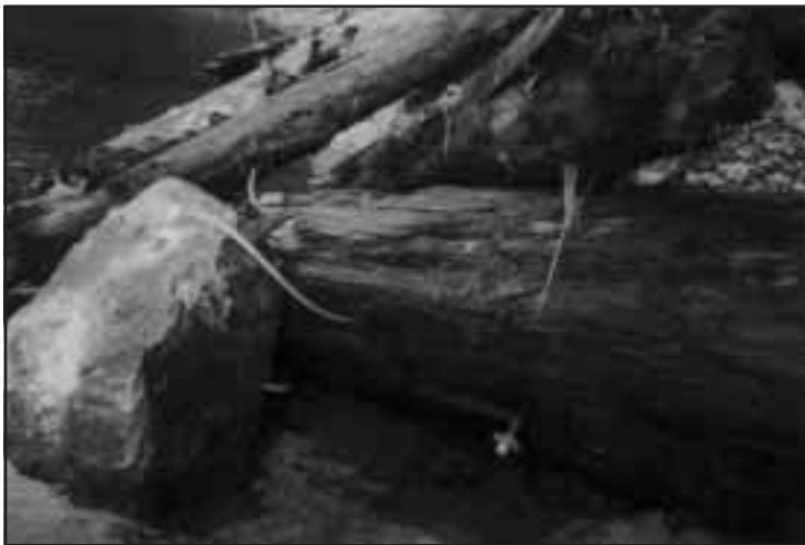
Figure 2-10. Various techniques used to anchor LWD structures. Some slack was left in the cable to accommodate shifting in high flows.
