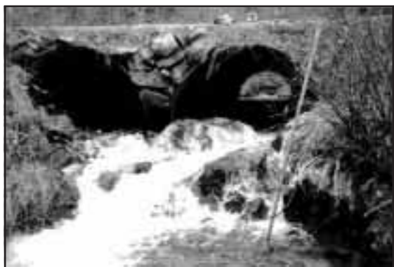
Figure 5-14. Culvert site at 19 km - 1300 Road, Cottonwood River watershed limiting fish access to 1.75 km of habitat. The outfall drop of 30 cm was followed by a cascade of 80 cm height.
