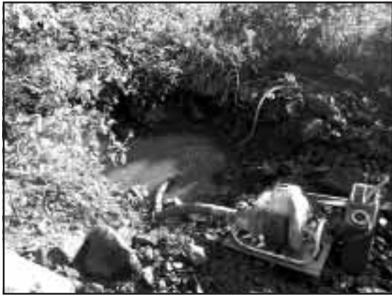
Figure 5-17. Stream diversion during instream works.
