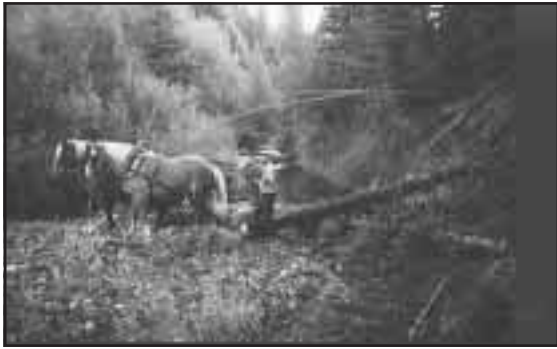
Figure 7-22. Draft horses placing LWD.
