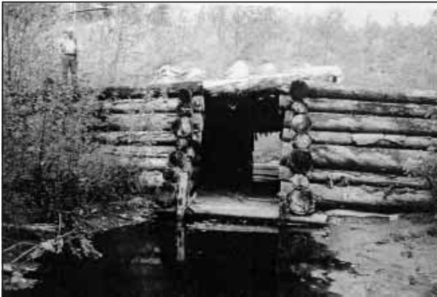
Figure 7-14. A view of the outlet of the box culvert crossing on Stubby Creek.
