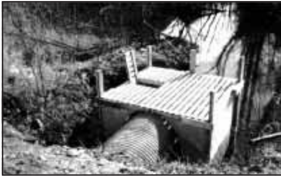
Figure 5-2. Culvert after beaver box installation on Dump Creek.
