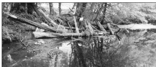
Figure 6-2. The triangulated structures were formed by using a series of triangles with the logs pinned together using rebar.
