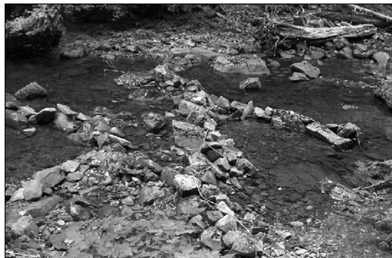
Figure 6-32. This boulder weir was constructed in reach 3. The main objective is to capture gravel moving downstream, however low velocity rearing habitat has also been created. The majority of the weirs were cabled together for much needed stability.
