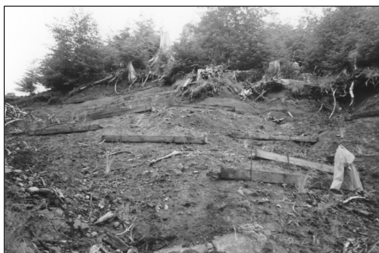
Figure 6-4. Construction view of bioengineered landslide.
