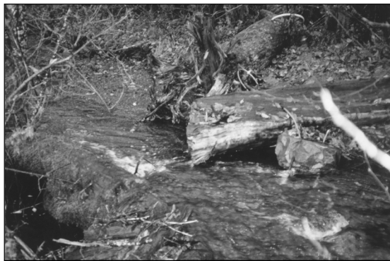
Figure 6-16. Post-construction view of a triangular logjam.
