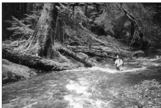
Figure 6–14. View looking upstream at a typical V-shaped log spur on Clew Creek.
