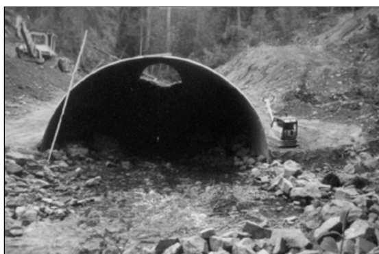
Figure 6-42. Arch culvert installed with flows re-established. The final construction stage was to replace road fill over the arch.
