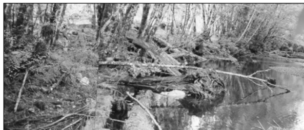
Figure 6-1. In Copper River mainstem, rocks attached by cable and epoxy ballasted the structures.
