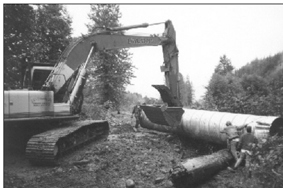
Figure 6-38. Installation of new 1500 mm culvert.
