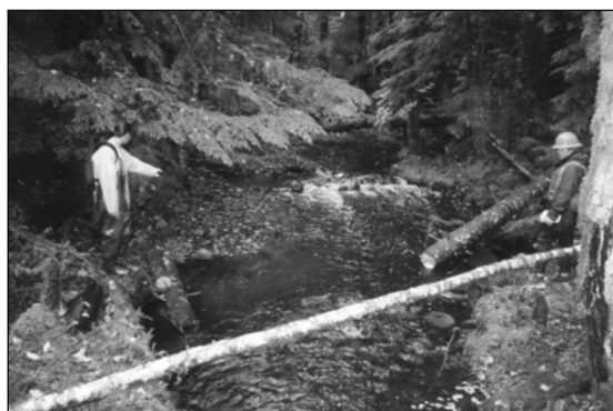
Figure 6–15. View looking upstream at a rock riffle and two LWD structures constructed by hand in Tributary 2.0 LB.
