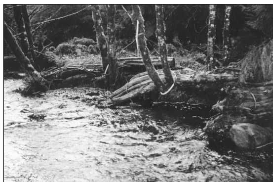
Figure 6-20. Post-construction view of log deflectors.
