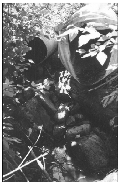
Figure 6-37. Outlet of two culverts perched 50 cm above the bed and only accessible at high flood river flows (inlet to left culvert buried).
