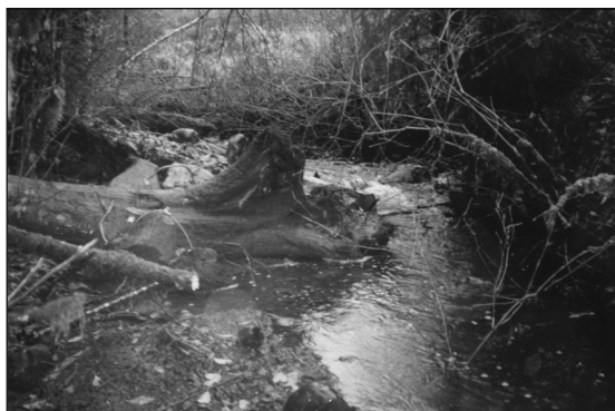
Figure 6-17. Post-construction view of a triangular logjam.
