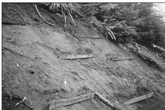
Figure 6-5. Construction view of bioengineered landslide.
