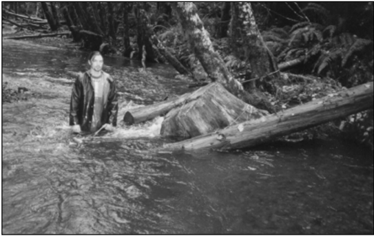
Figure 6–9. Placing instream structures in Weeping Willow Creek is expected to increase the scour and cover for fish.
