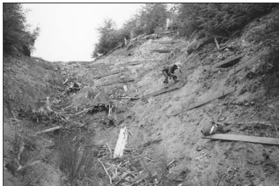
Figure 6-3. Construction view of bioengineered landslide.
