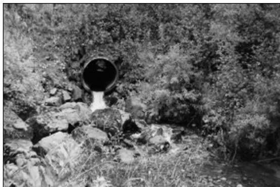
Figure 6-40. "Before" photo of 1960s constructed wooden stave culvert creating a full fish passage barrier on lower Fenton Creek.
