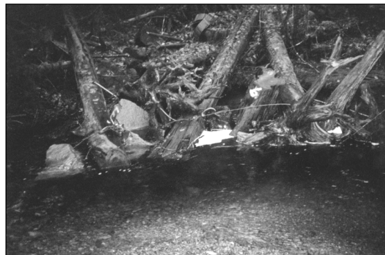
Figure 6-21. Post-construction view of a triangular logjams.
