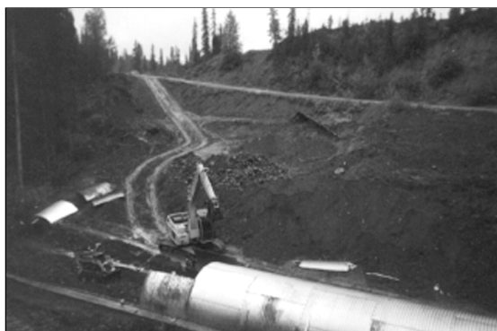
Figure 6-41. Placement of new arch culvert on concrete footings.
