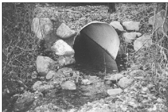
Figure 6-39. The new culvert provides upstream access to off-channel habitat and enables downstream migration of smolts.
