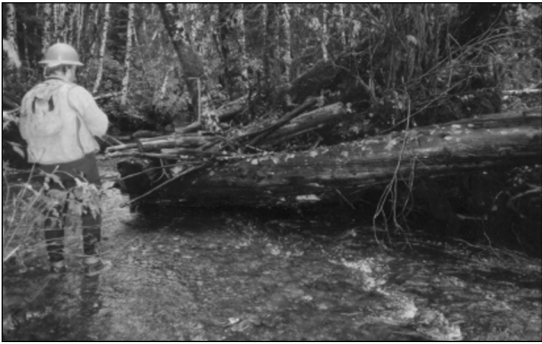
Figure 6–10. V-shaped lateral LWD spurs were placed in 11 locations in Weeping Willow Creek.
