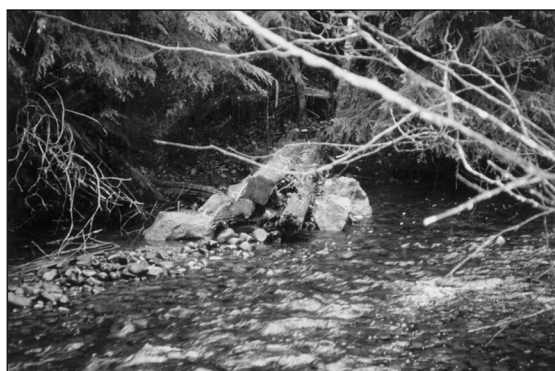
Figure 6-23. Post-construction view of a log deflector.
