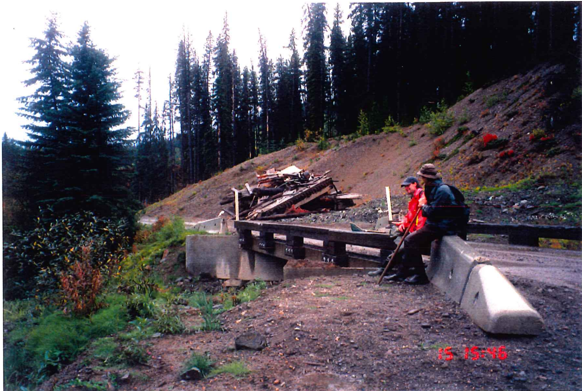
Plate #27: Logging bridge on Henrietta Creek Reach 4 (Site #13).
