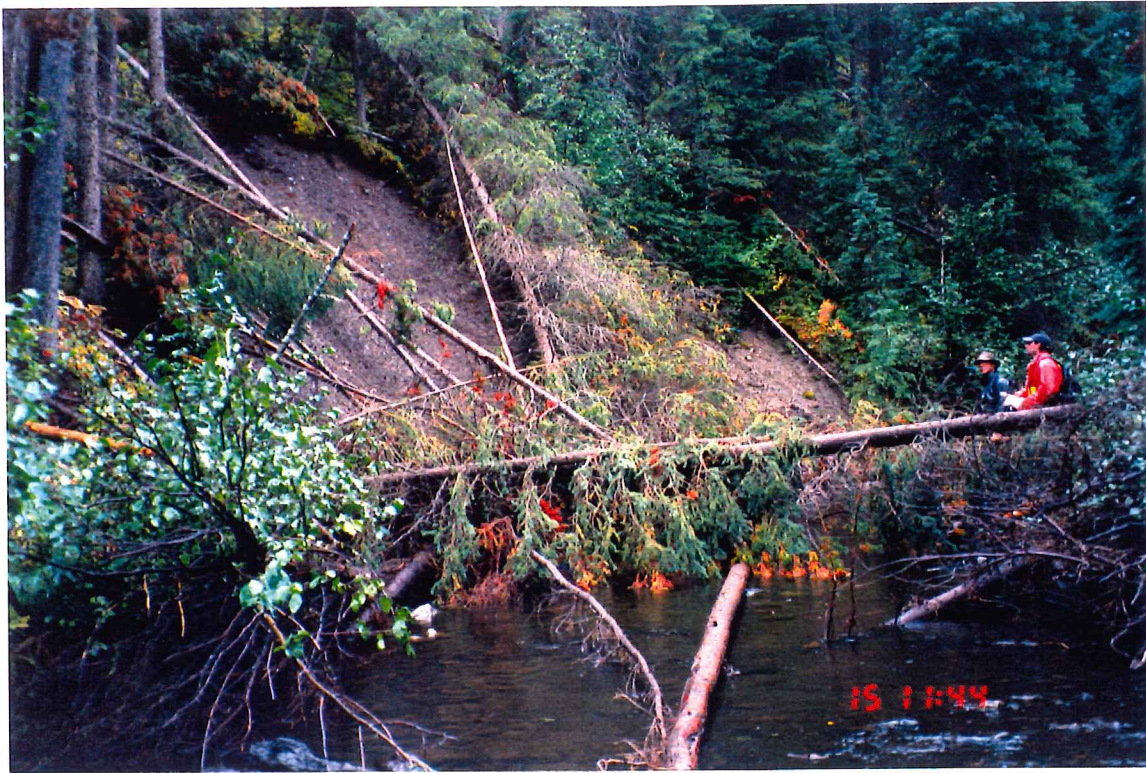
Plate #21: Natural slope failure on Henrietta Creek Reach 4 (Site#12).
