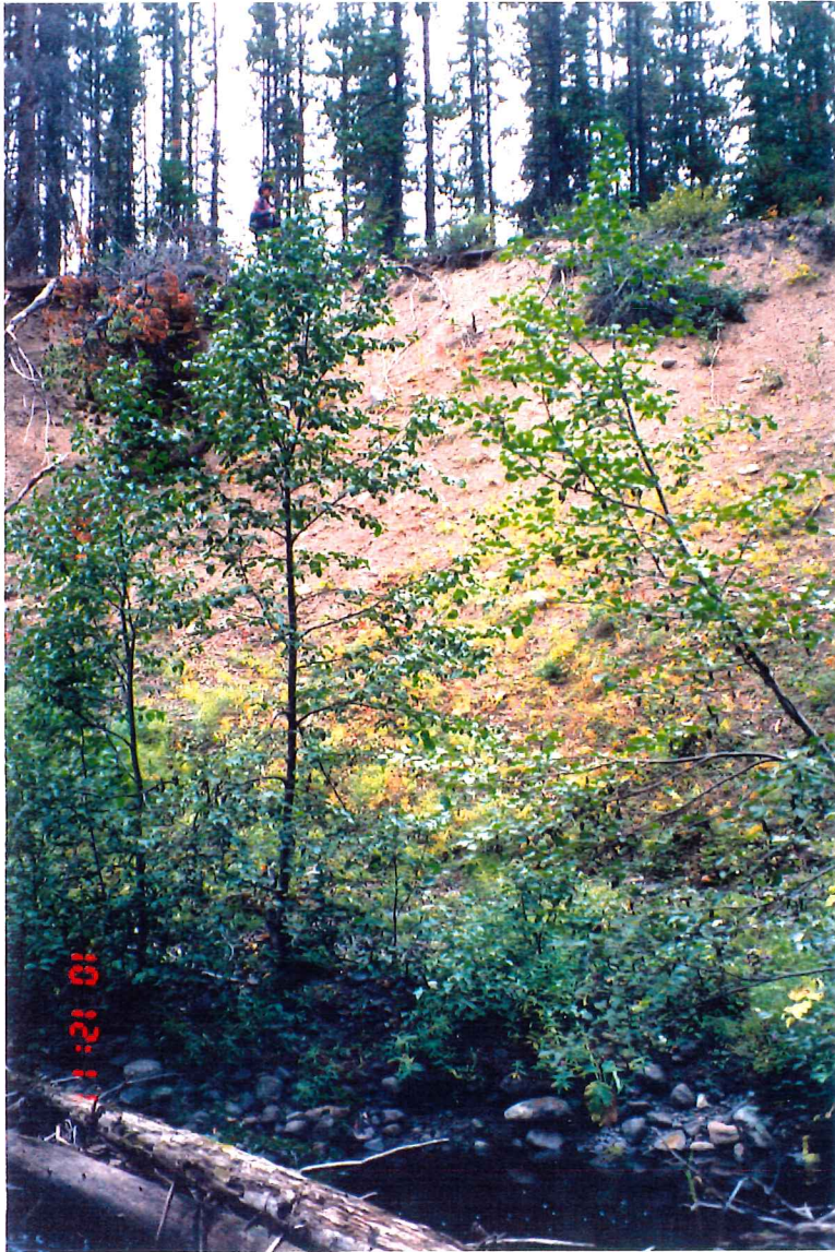
Plate #13: Natural slope failure on Lord's Creek Reach 1 (Site #8).
