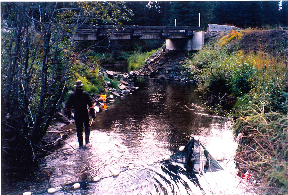
Plate #26: Logging bridge on Henrietta Creek Reach 4 (Site #13).
