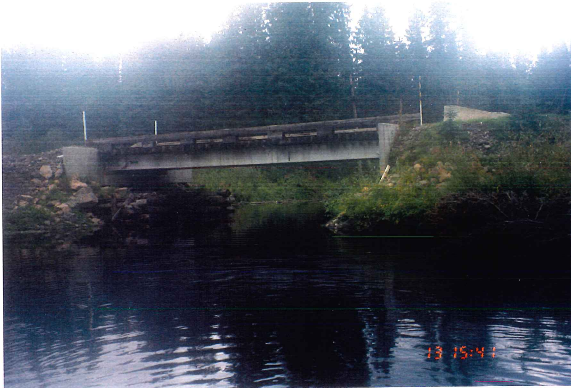
Plate #22: Logging bridge on Pinkut Creek Reach 6 (Site #11).
