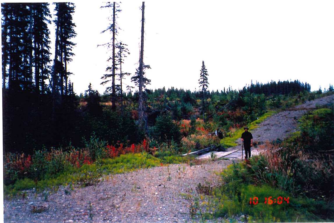
Plate #23: Logging bridge on Lord's Creek Reach 1 (Site #5).
