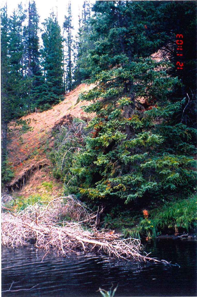
Plate #5: Natural slope failure on Pinkut Creek Reach 6 (Site #3).
