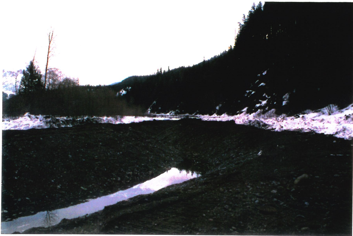
Photo 3. 16-Km side channel after bank sloping.
