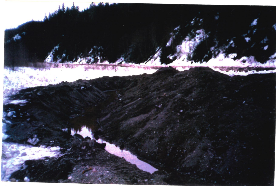
Photo 2. 16-Km side channel during the excavation.
