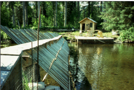
Counting weir at Damshilgwet Creek
