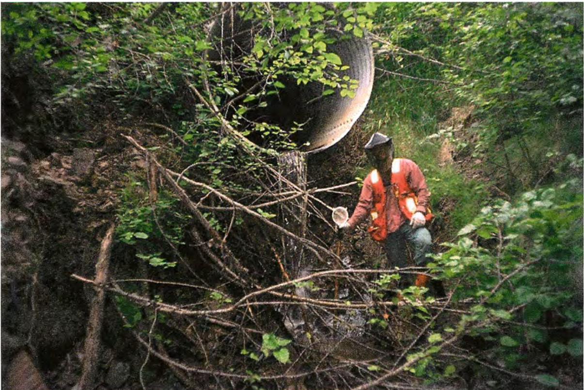
Direction of Photo: U CD #: 1 Image #: 19 Roll #: TC2 Frame #: 19 Comment: Culvert at Granisle Highway road crossing.
