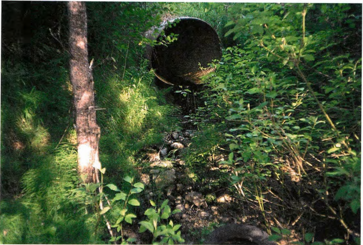
Direction of Photo: U CD #: 1 Image #: 28 Roll #: TC1 Frame #: 3 Comment: View at sample site approximately 40 metres downstream of Granisle Highway (shows culvert).
