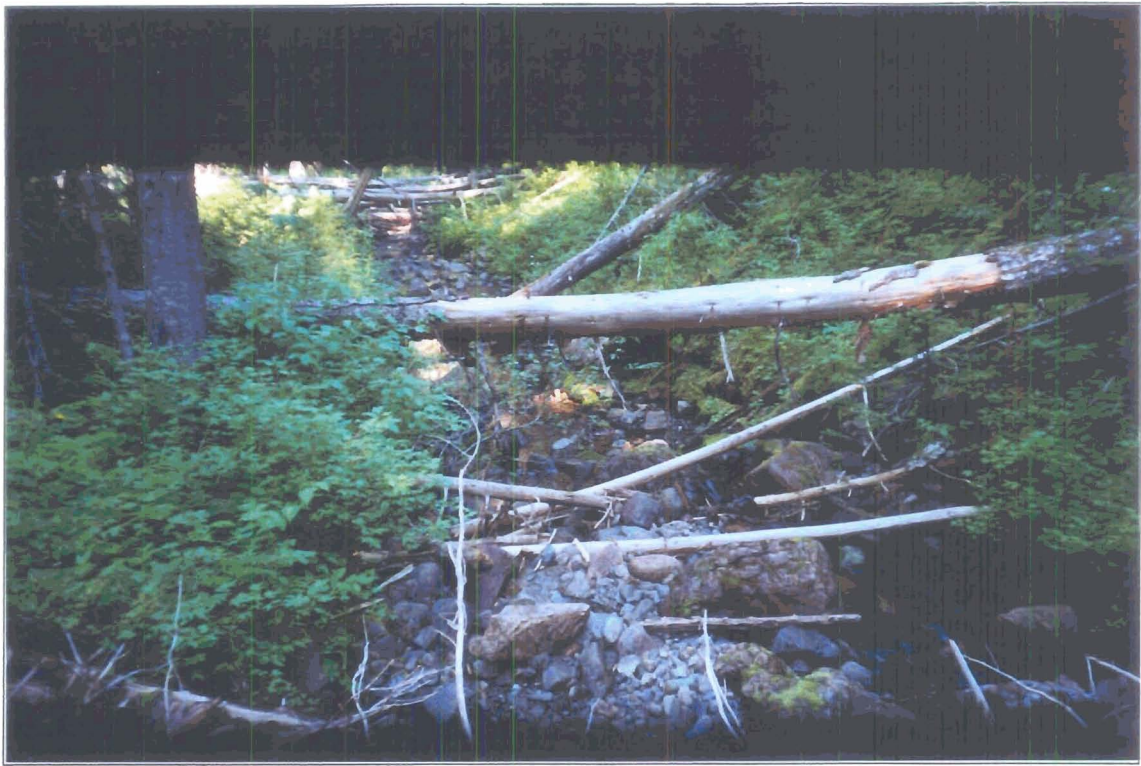
Site #38, downstream photo of substrates. Roll #62, Frame #19, Date: 2001/08/15
