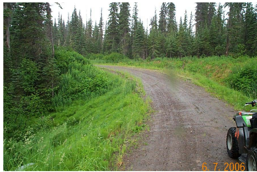
Figure 15. runoff from relatively small sediment source filters through relatively thick vegetation on road fill.
