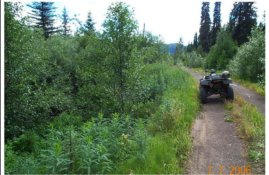
Figure 20. Small amount of sediment completely contained to road surface, ditches completely covered with vegetation
