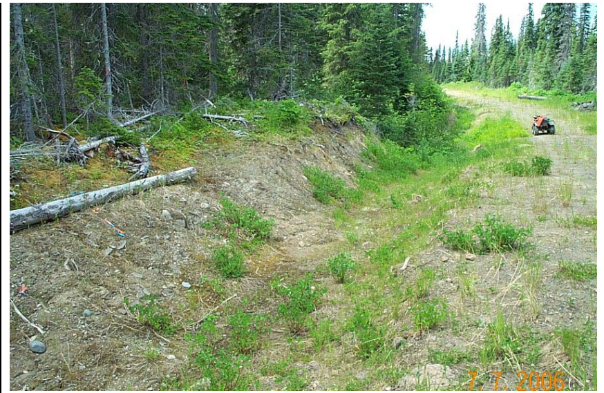
Figure 10. Crossing SB26-eroded material from small areas along ditch cut-slopes filter through thin vegetation before spilling into stream
