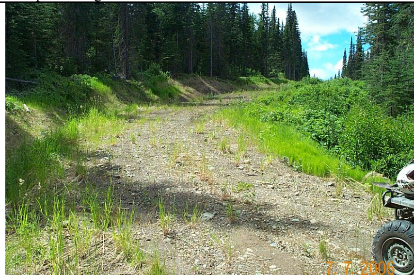
Figure 7. Crossing SB27 long uninterrupted road surface.
