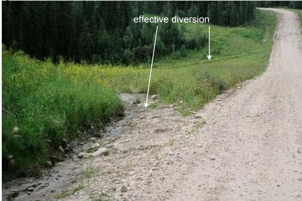
Figure A1-4 Long tail ditches with a progressively decreasing slope helps to slow and re-direct road surface runoff water away from the stream where it can percolate into the forest floor.
