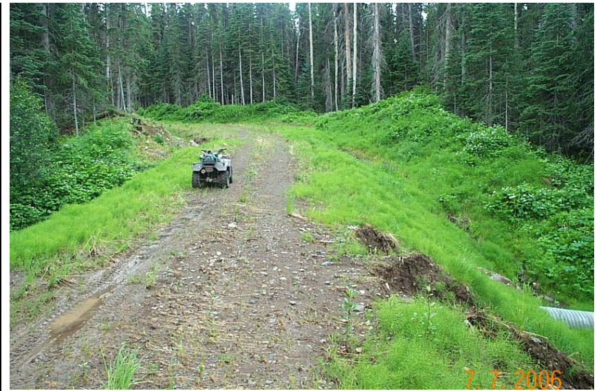
Figure 6. Crossing SB19-runoff water cuts road fill and spills directly into stream.
