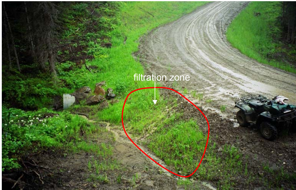
Figure A1-8 A small filtration zone coupled with sparse grass and a steep gradient is shown to be ineffective at filtering sediment.
