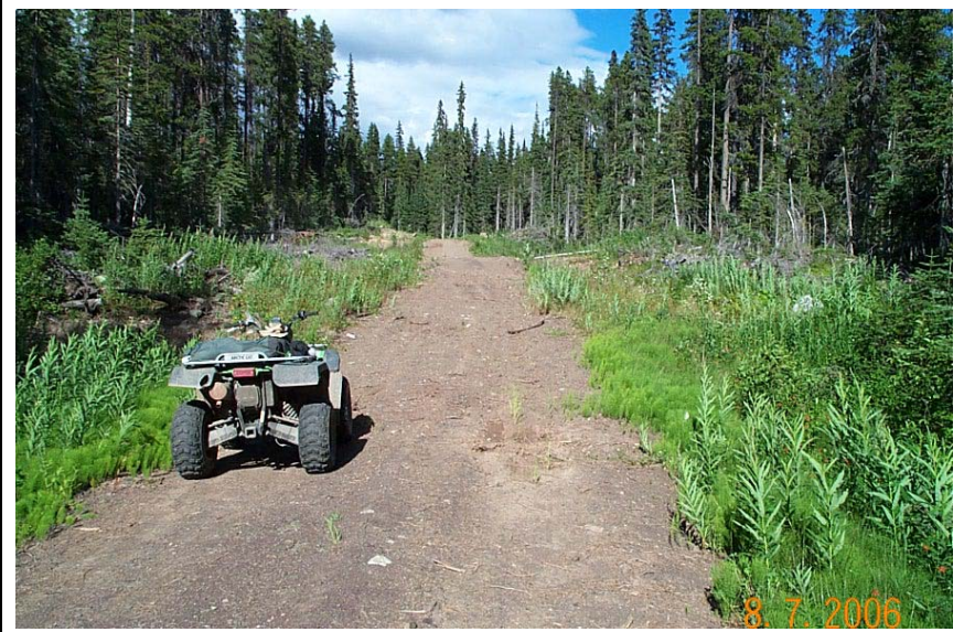
Figure 16. Sediment from road surface mostly trapped by depressions in road.
