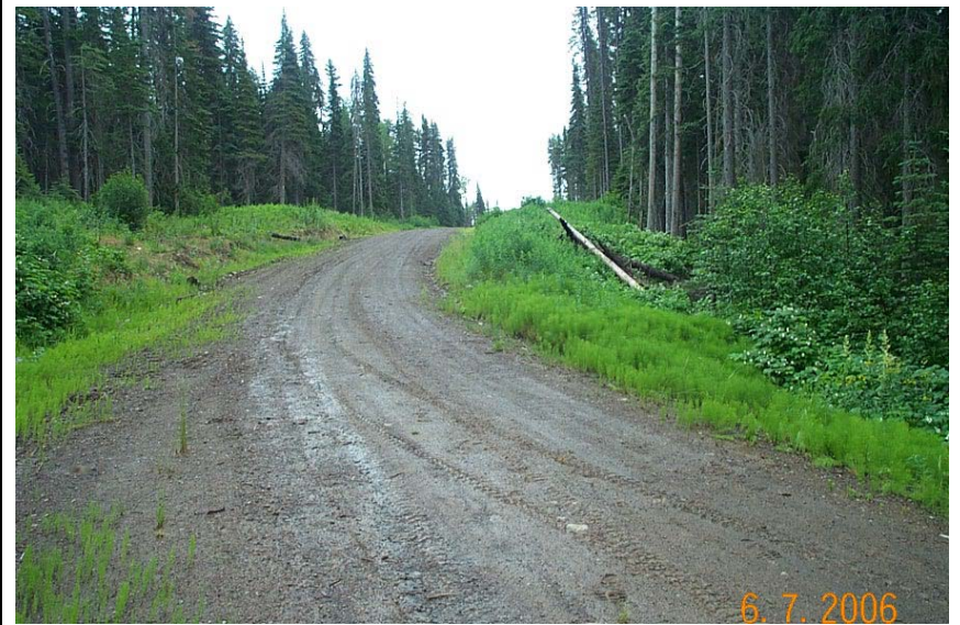
Figure 12. Crossing SB14-runoff water confined to road surface spills over shoulder into stream.
