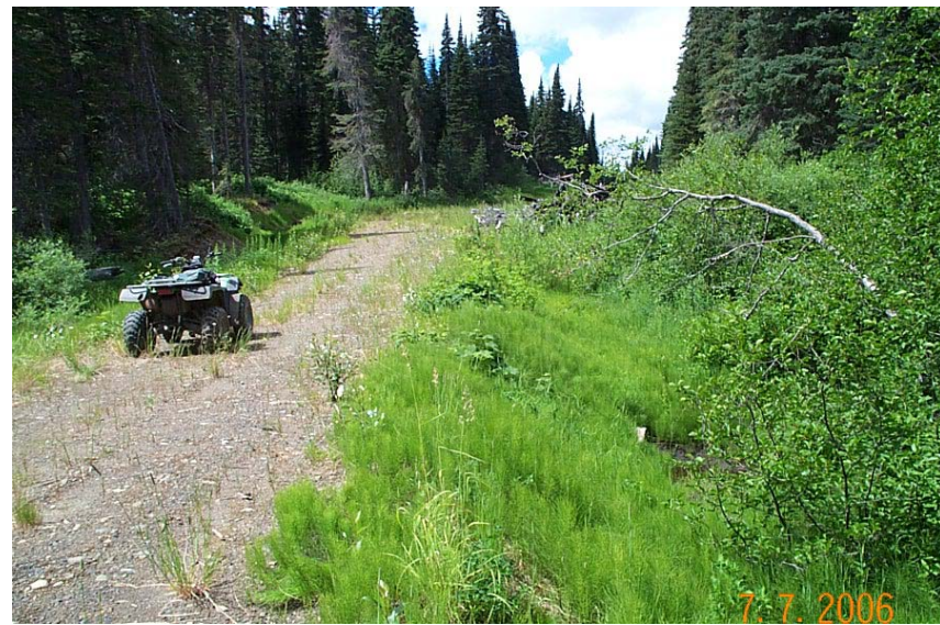
Figure 19. Road surface crowned with coarse material, ditches and fill slopes completely covered with vegetation.
