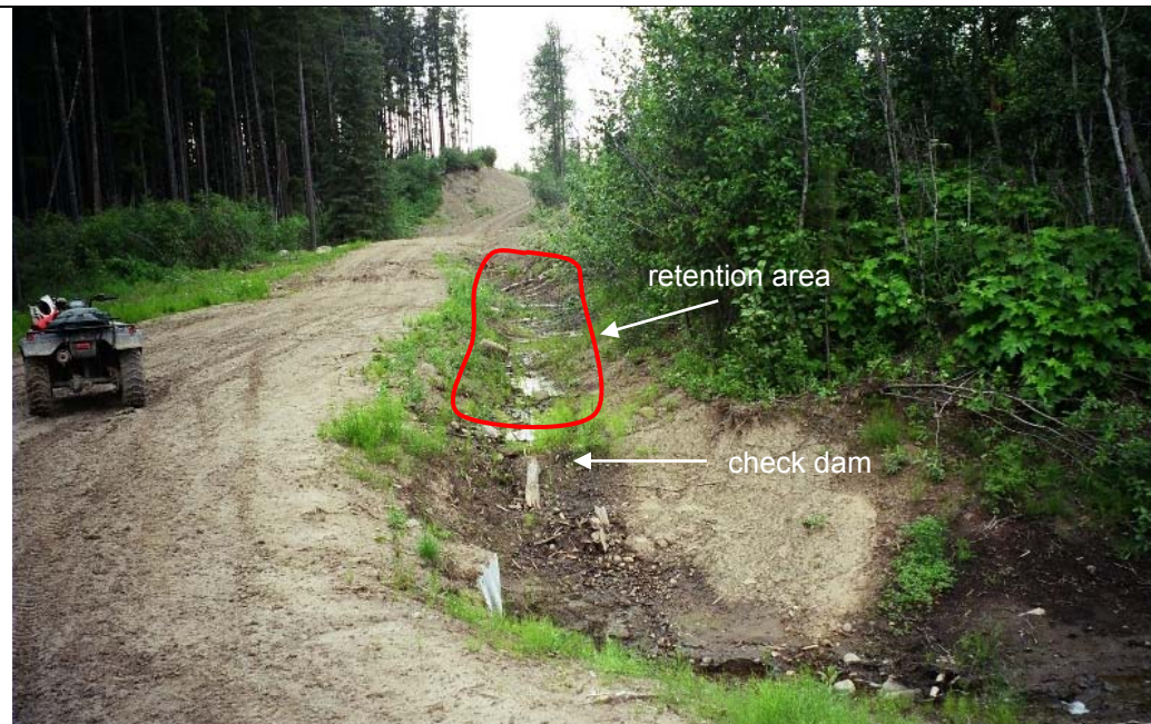
Sediment pond created by placement of large rocks in the ditch structure. Relatively low sediment in-filling has occurred and structure functions as intended.
