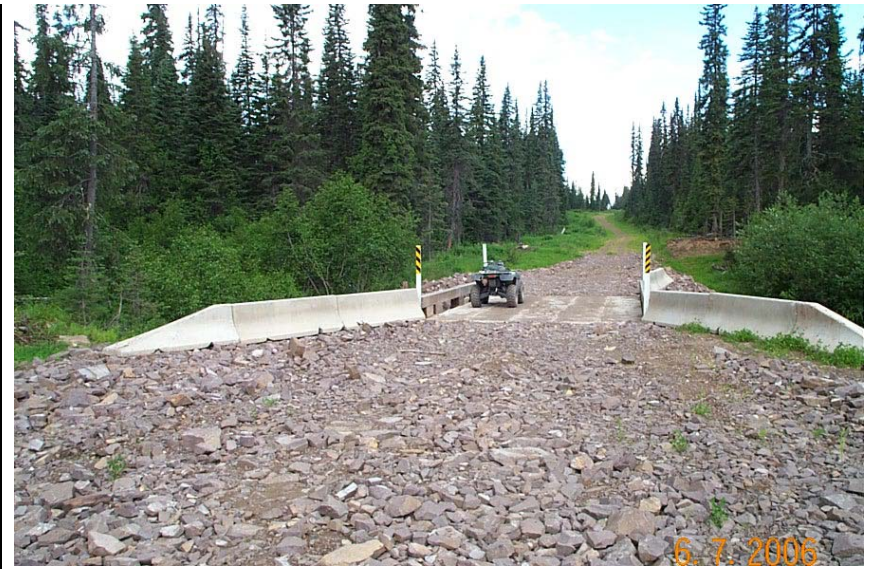
Figure 18. Crossing SC08- bridge deck slightly elevated and all sediment sources completely covered with large, coarse material.
