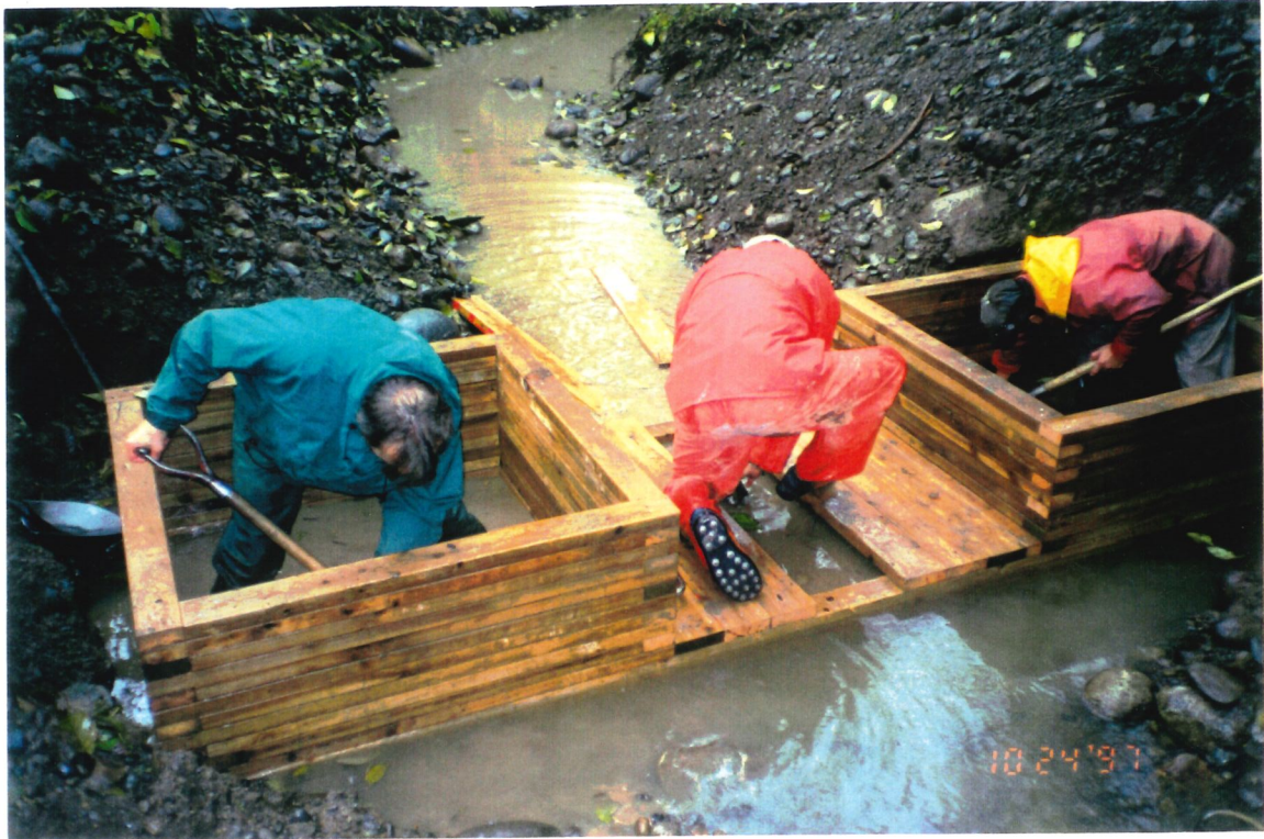
Photo 5: Box culvert construction; controls flow into side channel.
