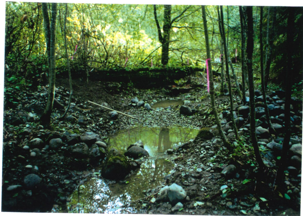
Photo 2: Side channel after excavation.
