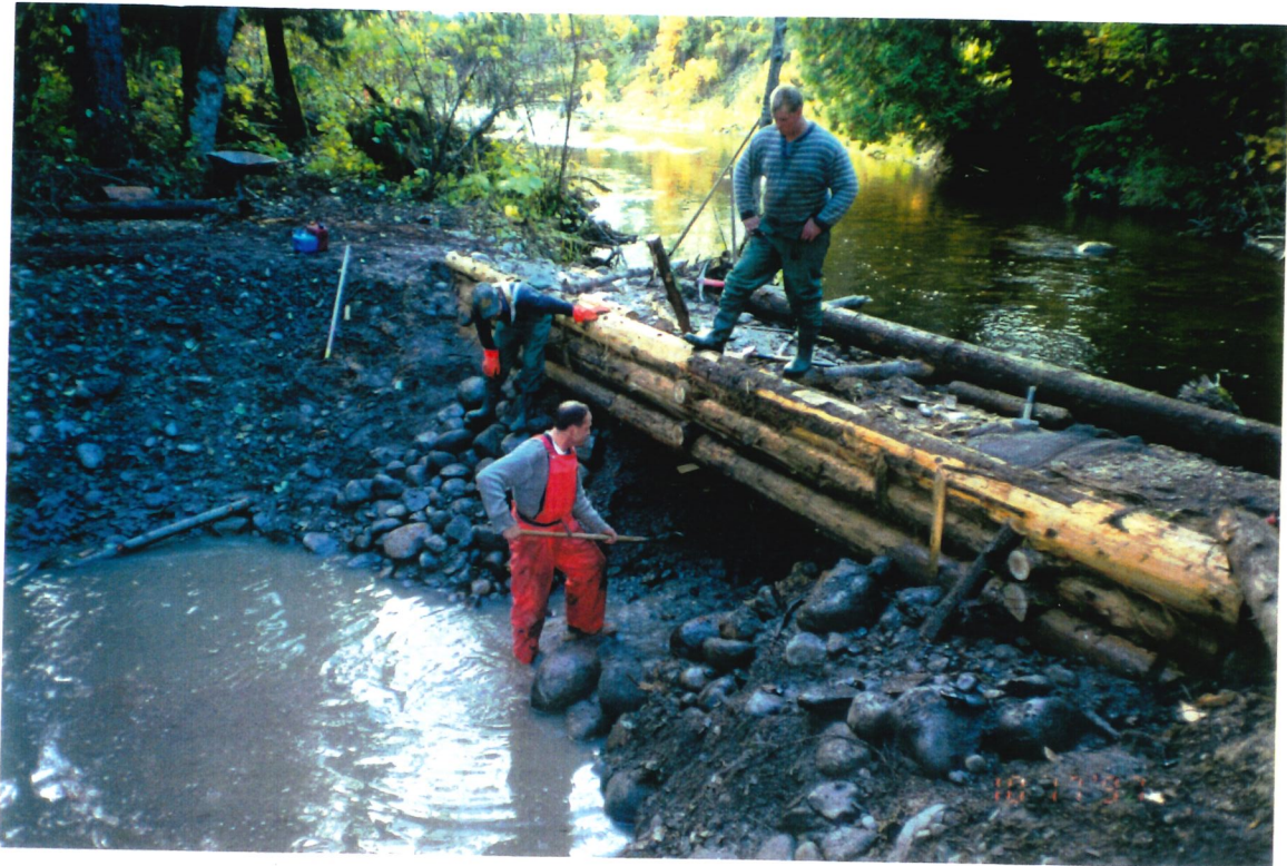
Photo 3: Berm construction.
