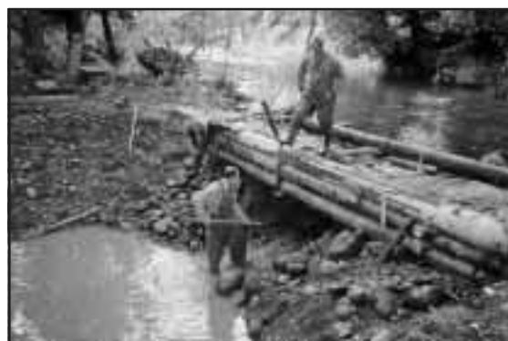
Figure 6-13. Construction of a berm to protect off-channel development.
