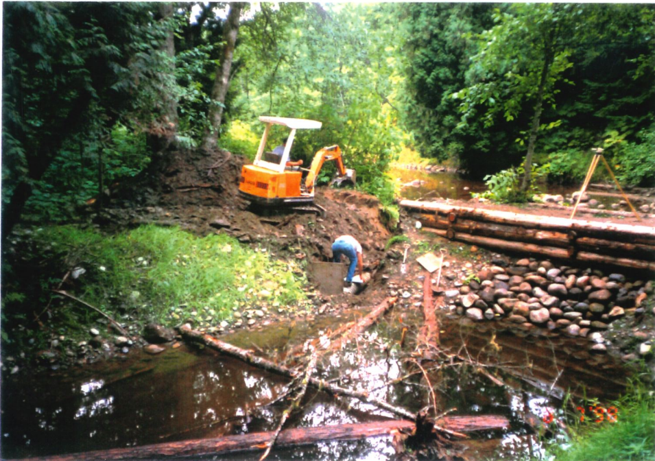
Photo 8: Culvert installed August 1998 to allow additional water flow from Deep Creek.
