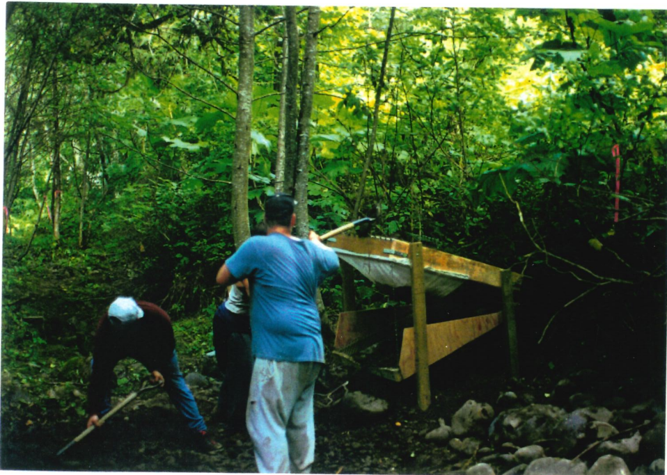
Photo 4: Gravel grader, constructed by TSES.
