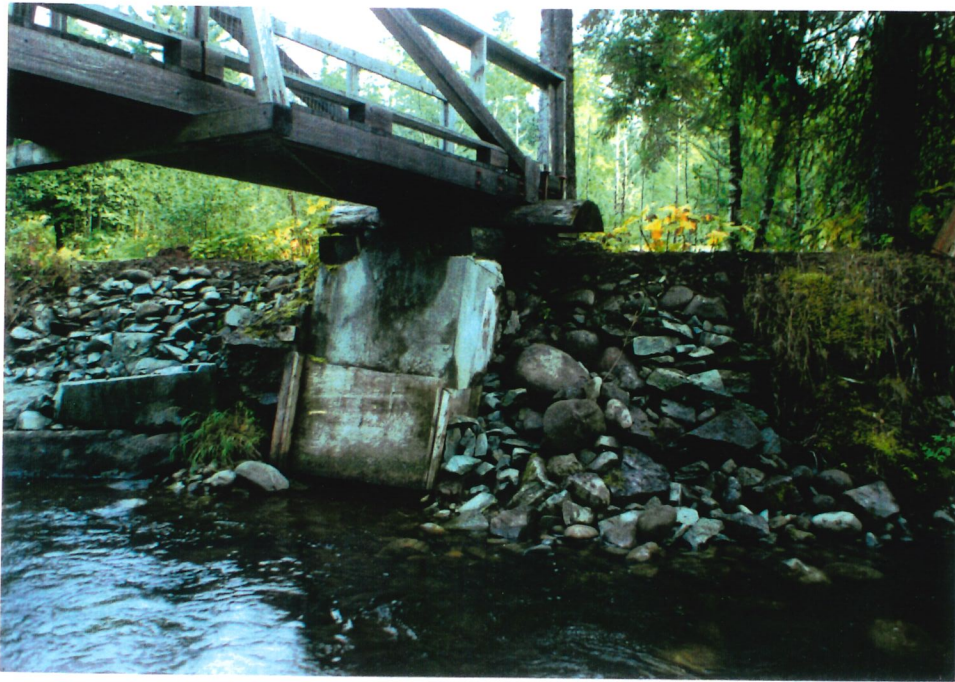
Photo 7: Bank stabilization below the walking bridge.
