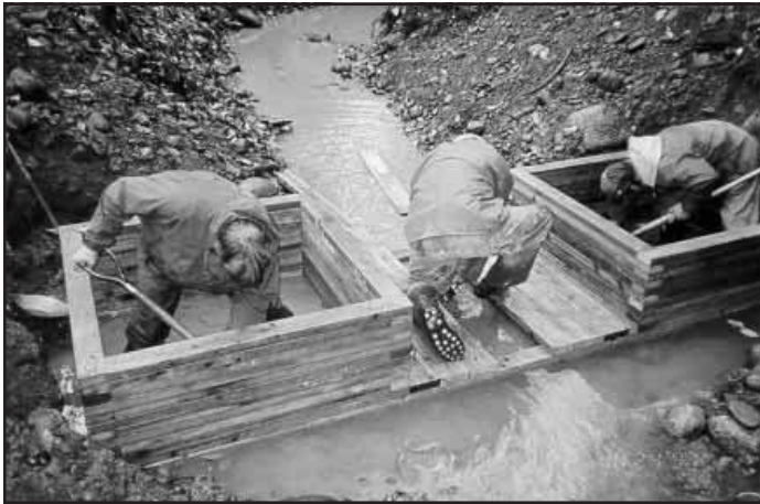
Figure 6-14. Box culvert construction; controls flow into side channel.
